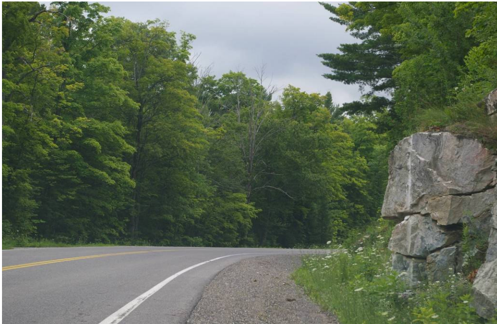
Figure 2.4 Fixed object hazard adjacent to CR 511 near the community of Tatlock
