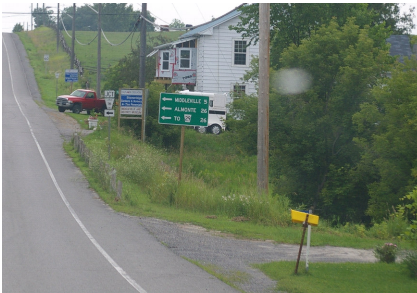
Figure 2.5 Three cable guide rail system does not provide adequate protection of embankment
