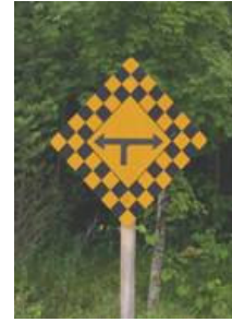
Figure 2.13 Non-standard checkerboard sign (CR 36 near community of Bolingbroke)
