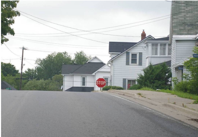
Figure 5.10 Stop sign placement on CR 511 approaching CR 12 (South Street) – south approach
