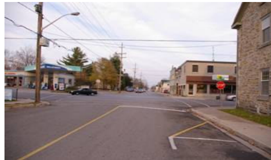
Figure 5.6 View of stop sign on eastbound approach
