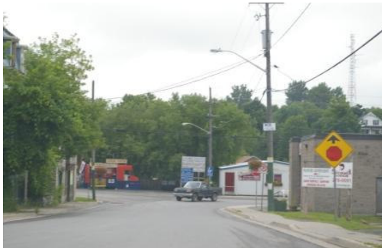
Figure 5.11 Stop sign placement on CR 511 approaching CR 12 (George St) – east approach
