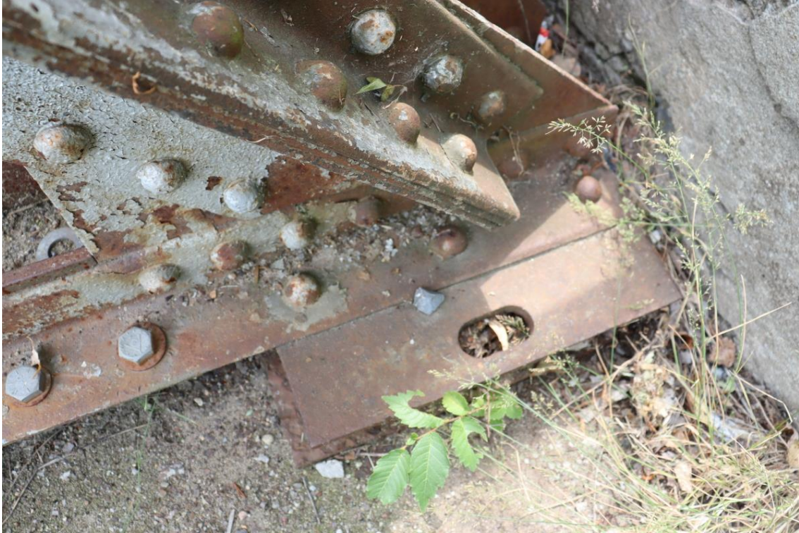
Figure 33: NW truss bearing
