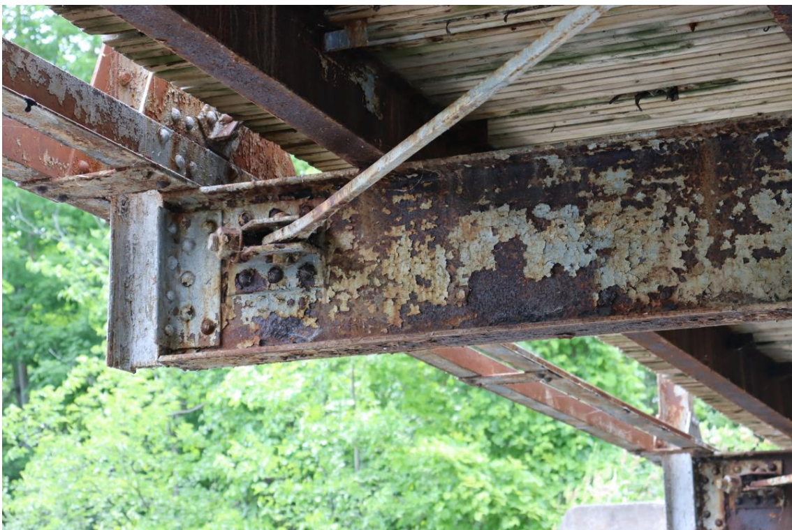
Figure 22: Floor beam 2 south end
