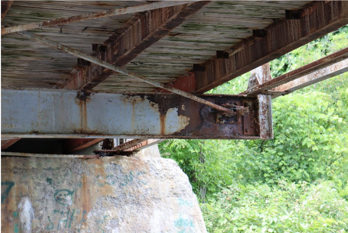
Figure 23: Floor beam 1 north end
