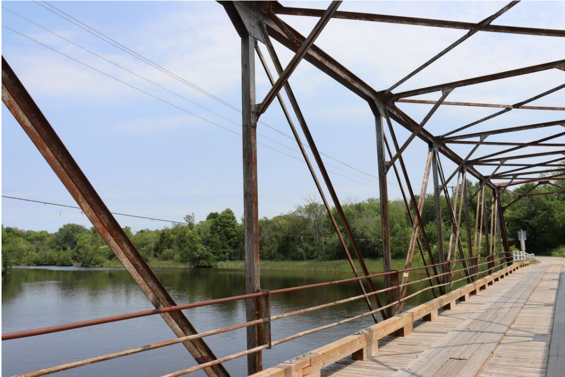
Figure 65: North truss
