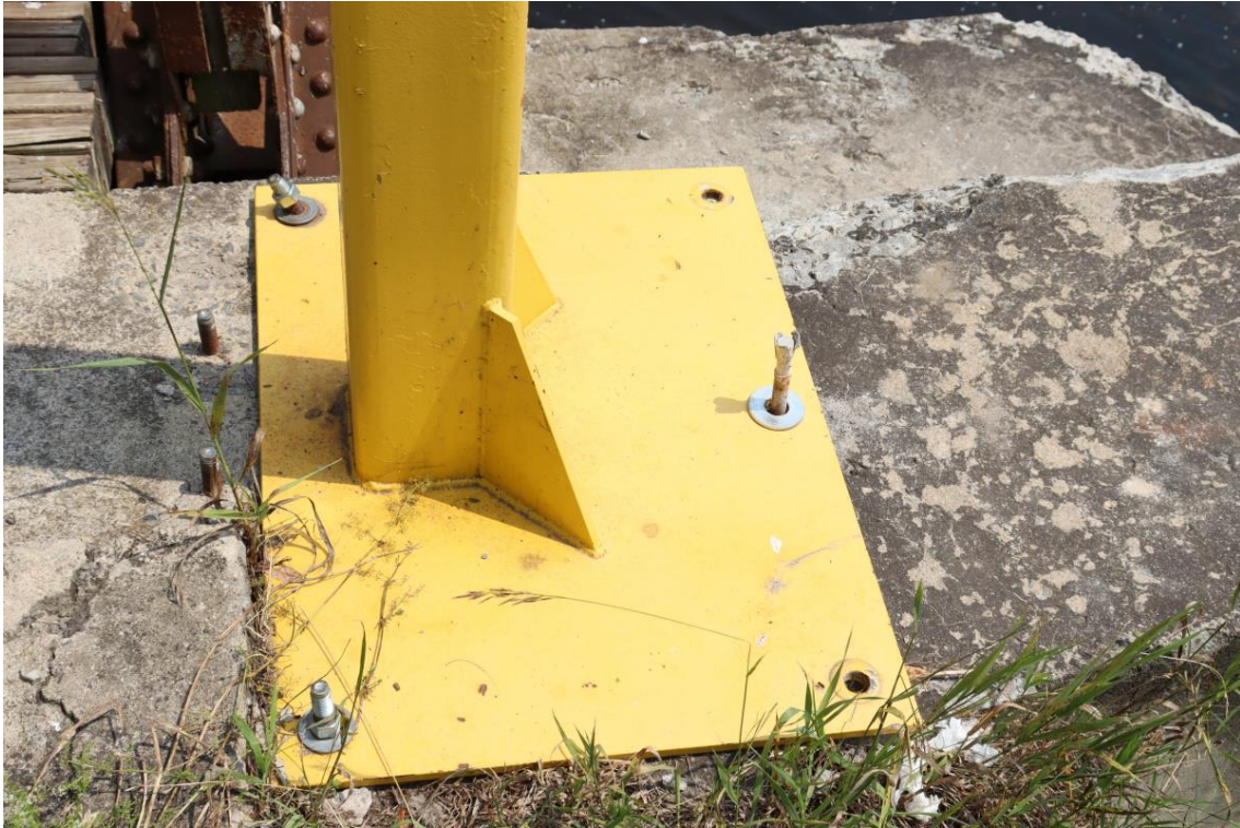
Figure 41: SW portal base
