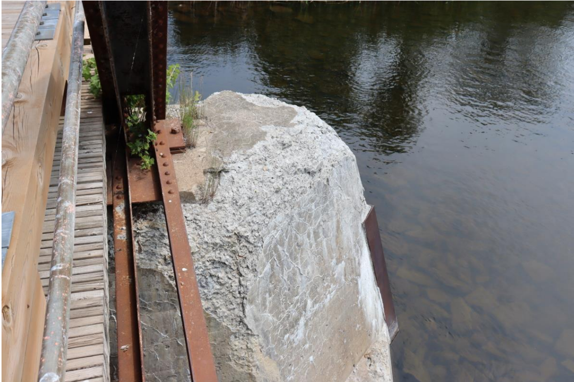
Figure 55: Pier top south side from west
