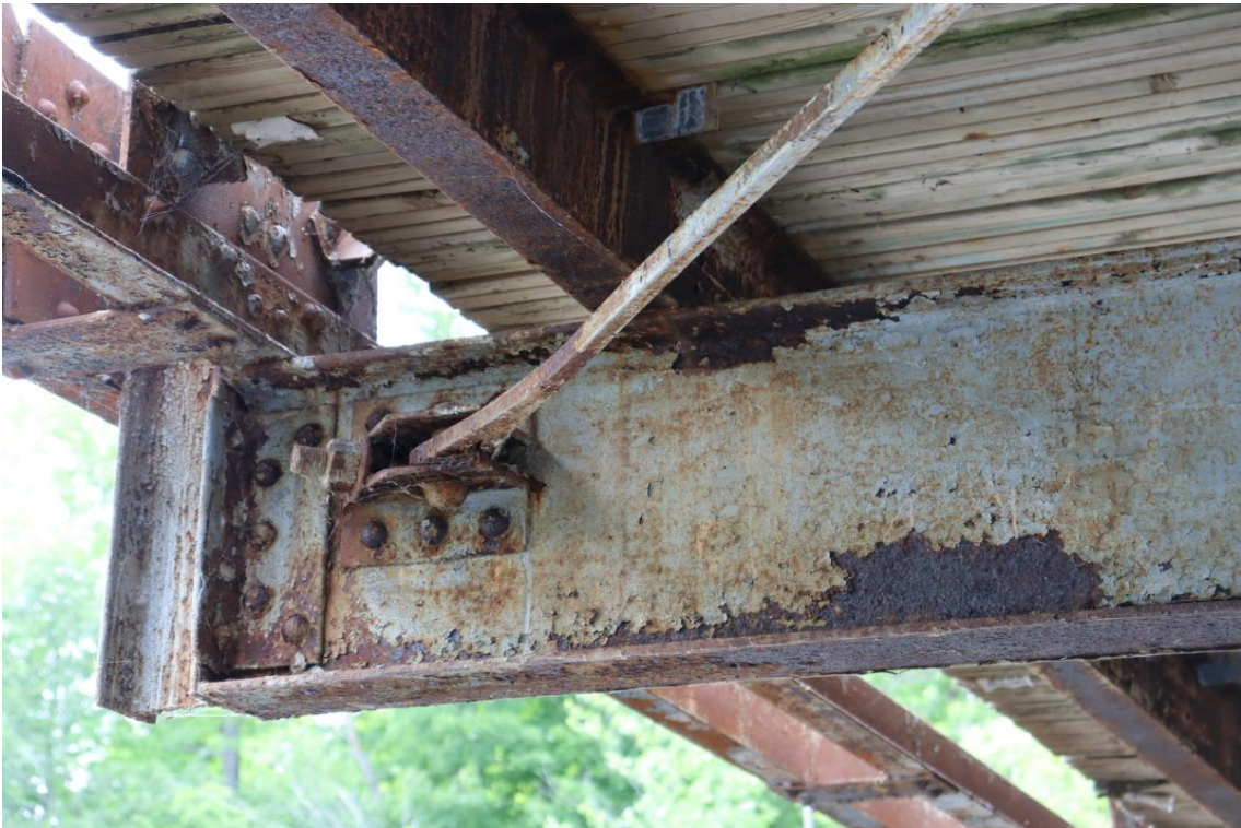
Figure 18: Floor beam 4 south end
