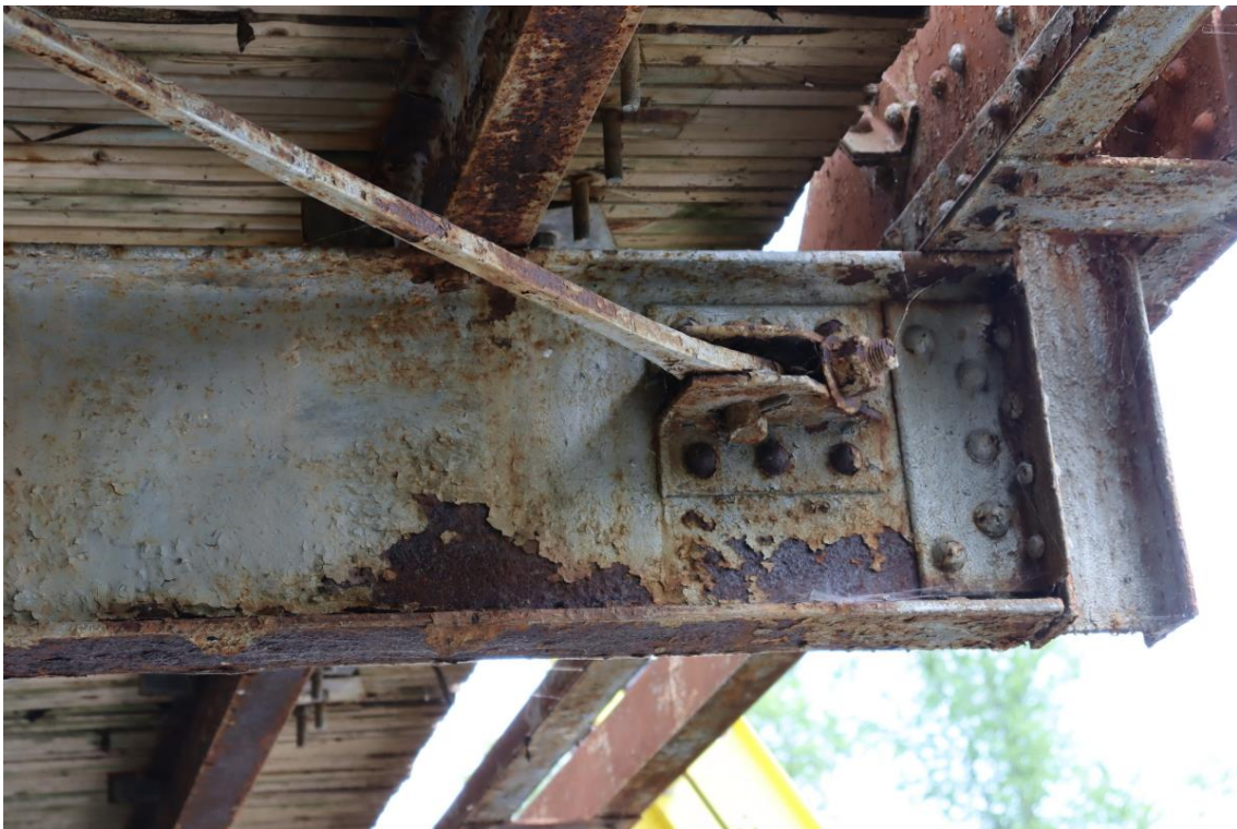
Figure 16: Floor beam 5 south end
