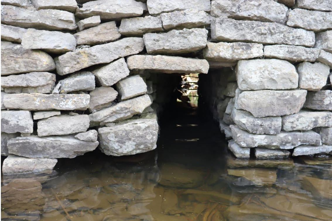
Figure 51: Drainage opening through causeway
