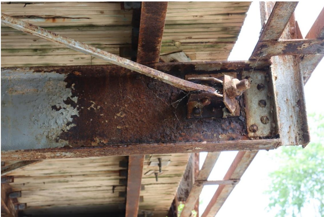
Figure 12: Floor beam 7 south end
