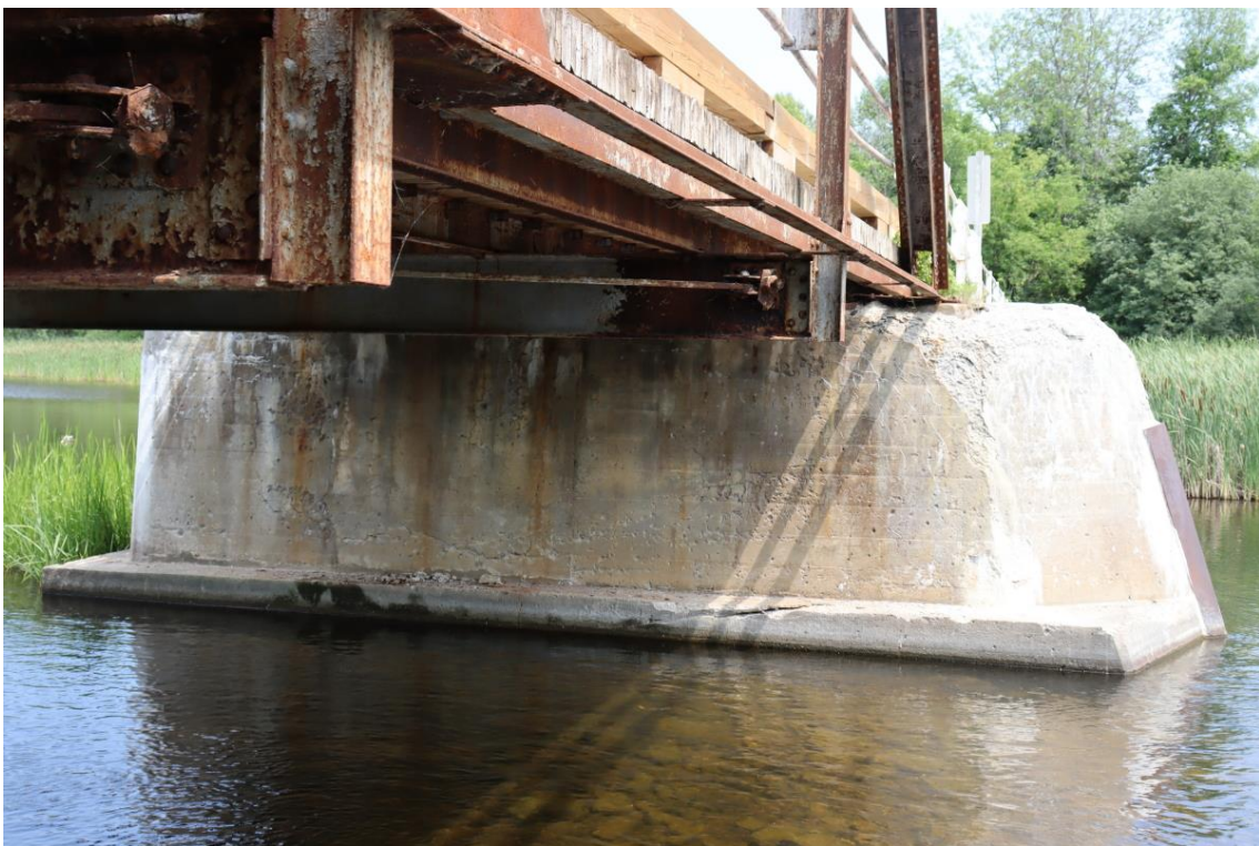
Figure 40: West face of pier
