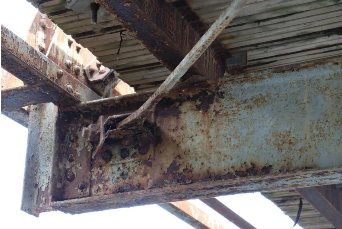
Figure 13: Floor beam 6 north end
