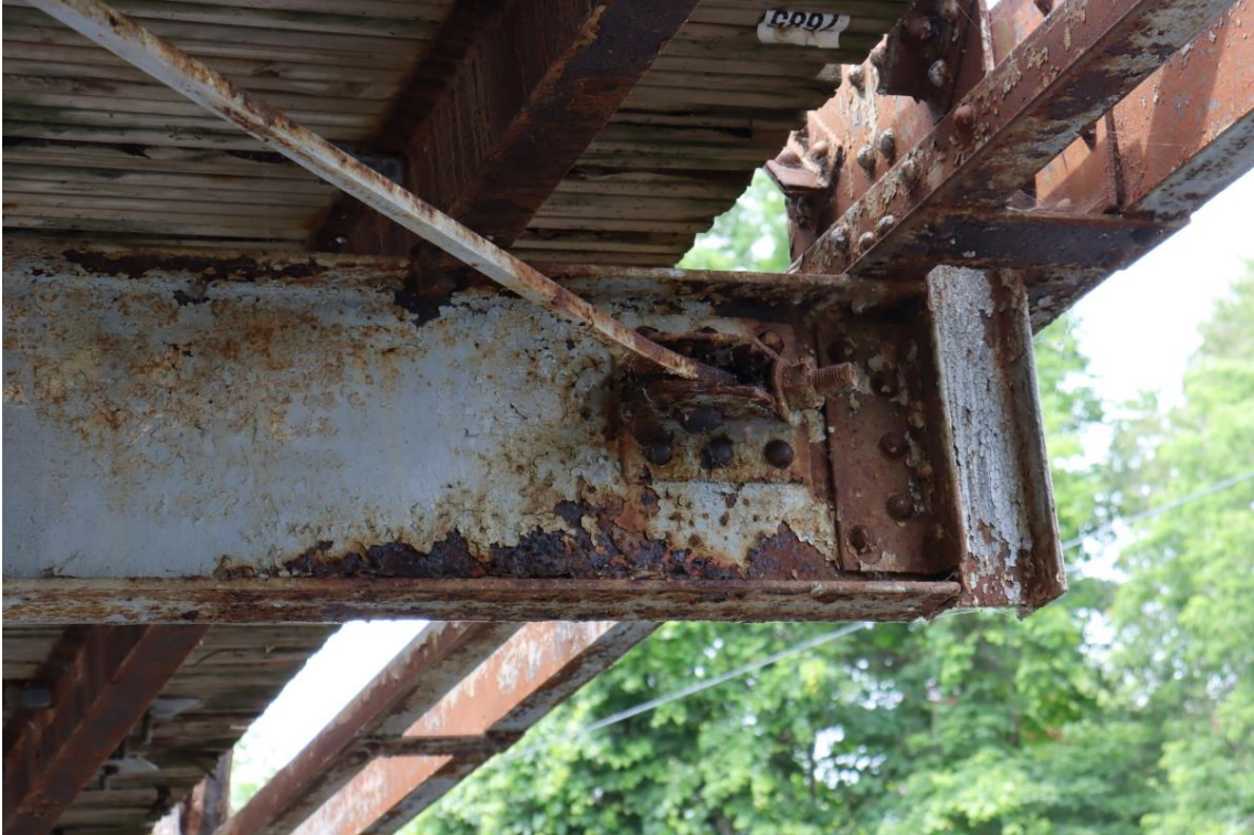
Figure 17: Floor beam 4 north end
