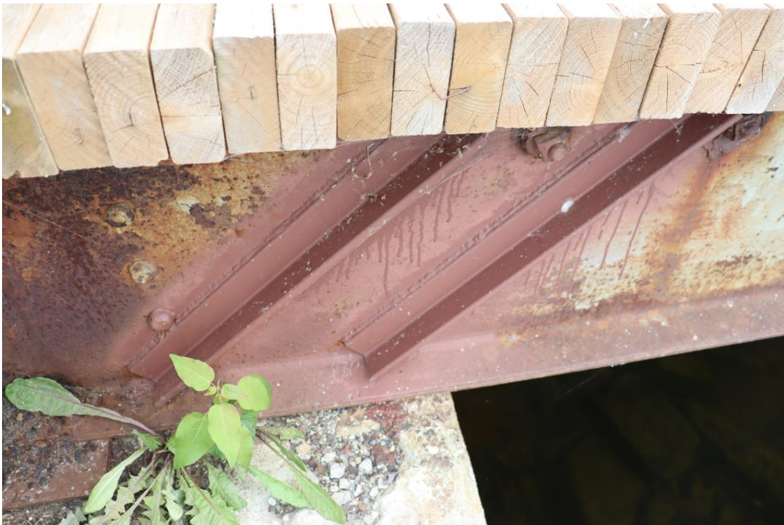
Figure 26: NE girder end web stiffening
