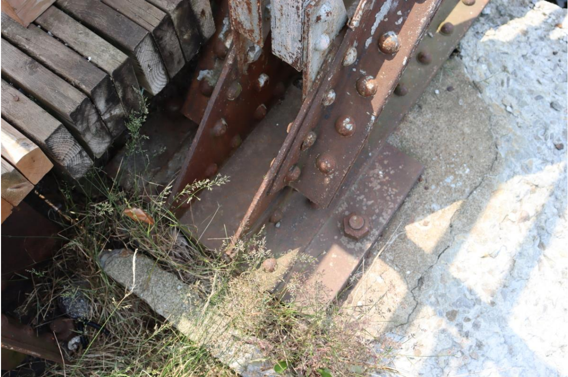
Figure 45: North pier truss bearing
