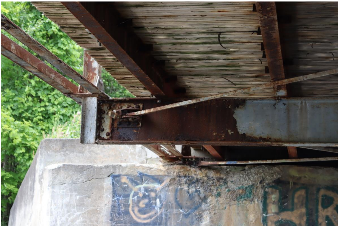
Figure 24: Floor beam 1 south end
