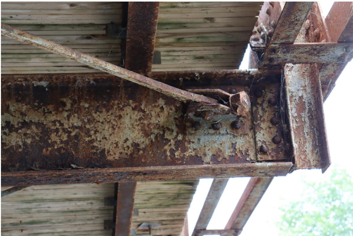
Figure 14: Floor beam 6 south end
