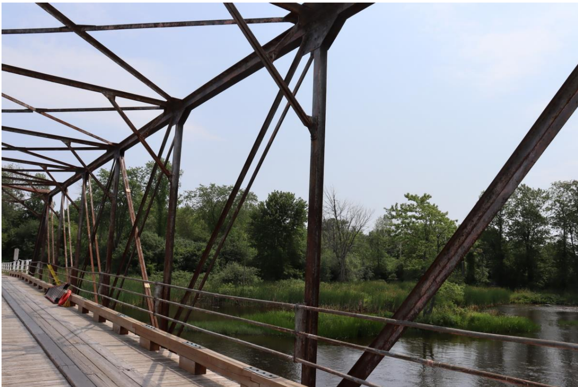
Figure 62: South side truss
