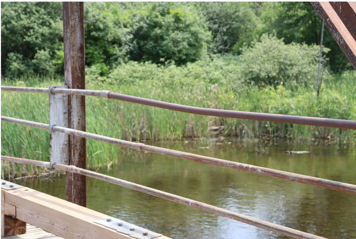
Figure 58: South pipe railing
