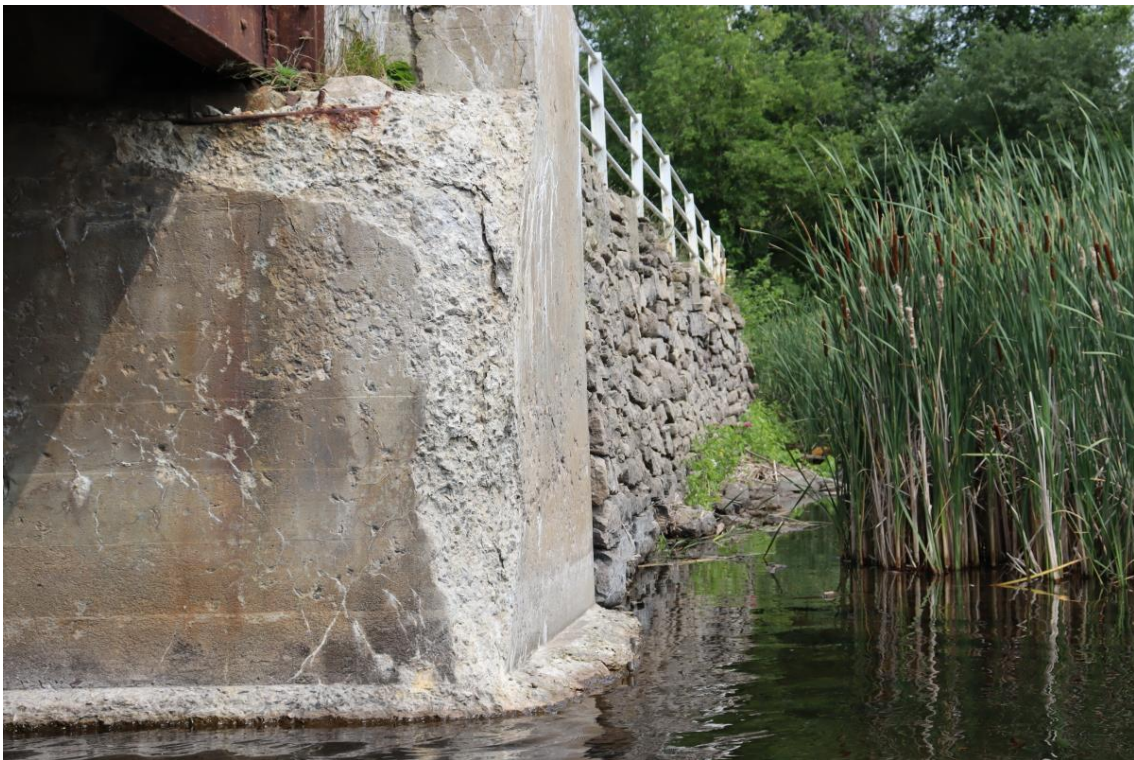
Figure 28: East abutment and causeway from south
