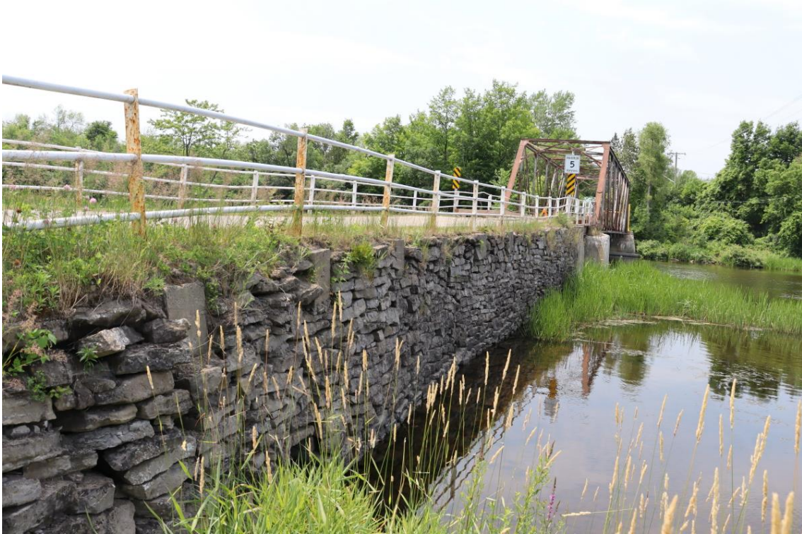
Figure 53: North dry-stone retaining wall east approach
