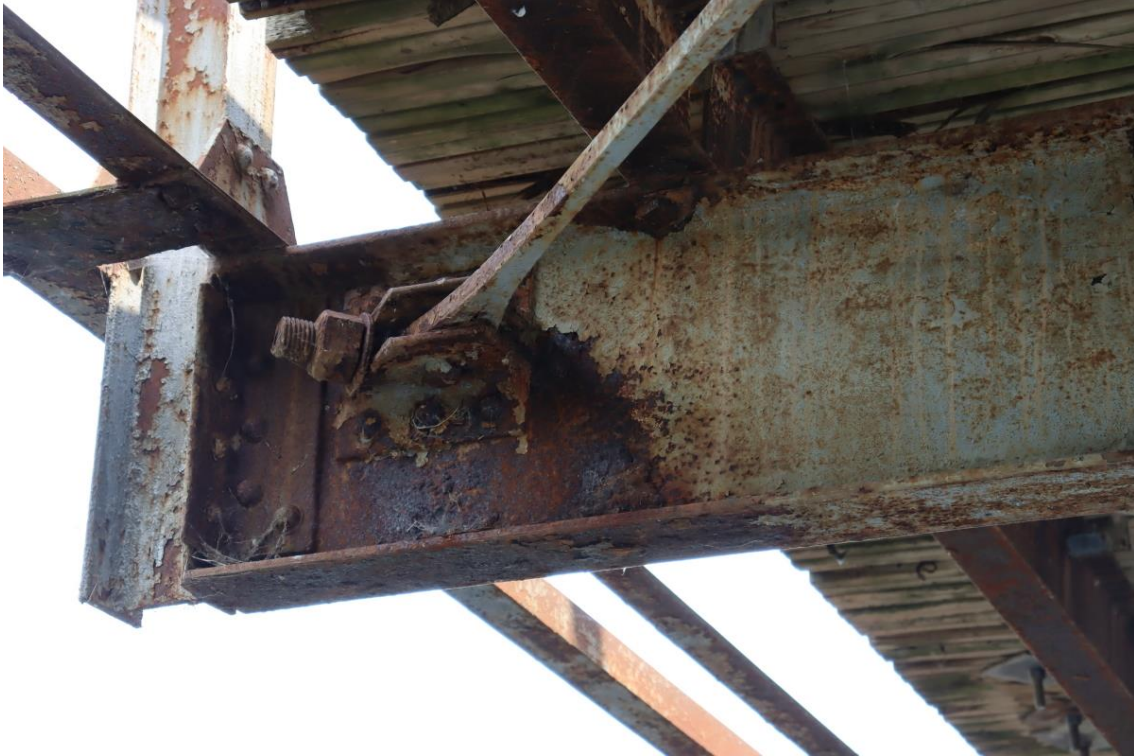
Figure 11: Floor beam 7 north end
