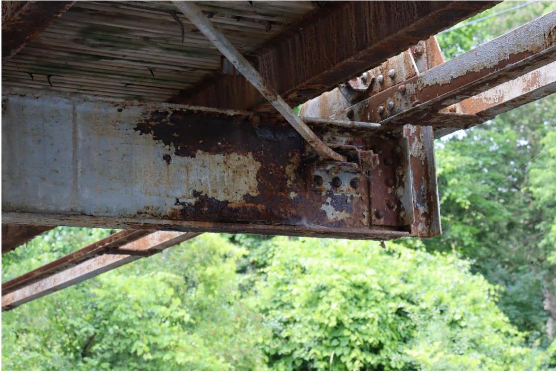
Figure 21: Floor beam 2 north end
