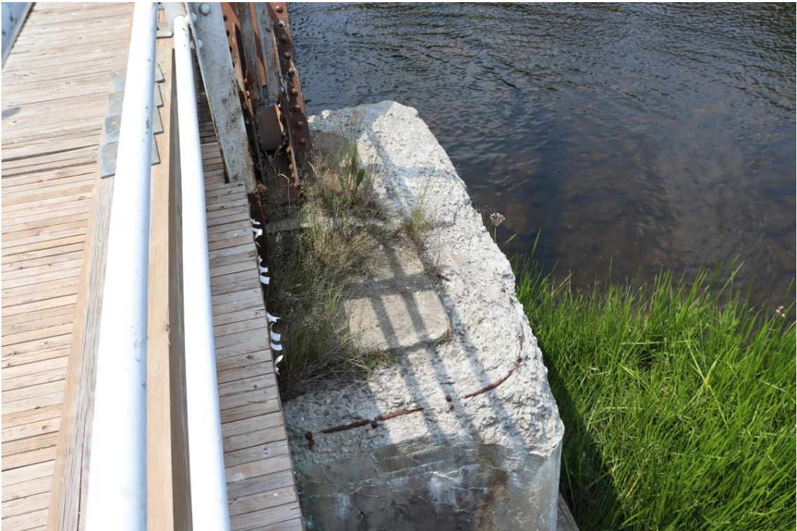
Figure 46: Pier top north end
