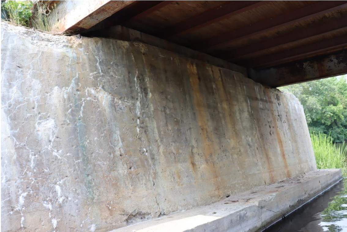
Figure 27: East face of pier
