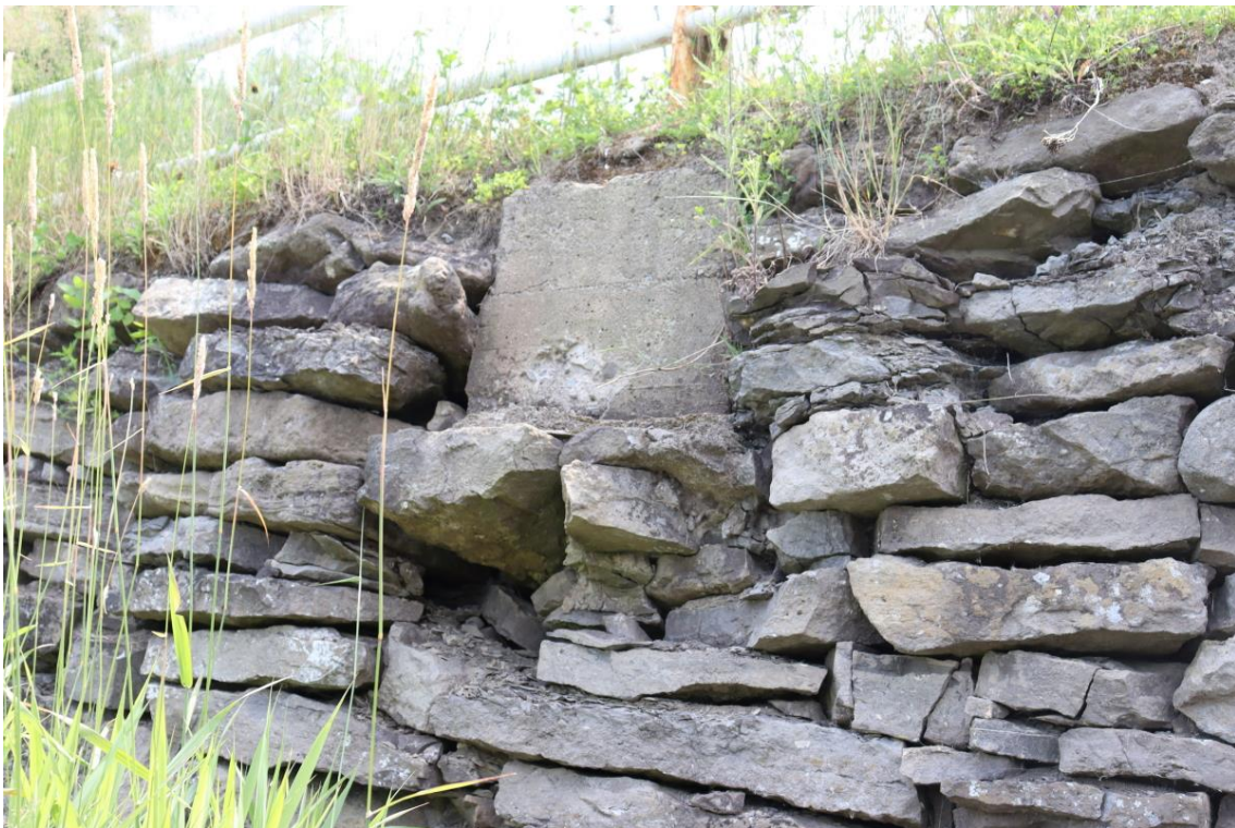
Figure 50: North-east quadrant dry-stone retaining wall
