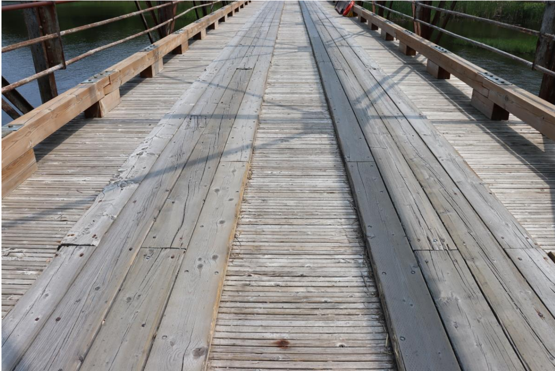
Figure 61: Deck surface looking west
