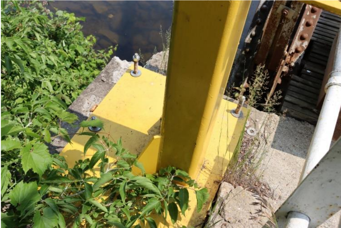
Figure 67: NW portal base
