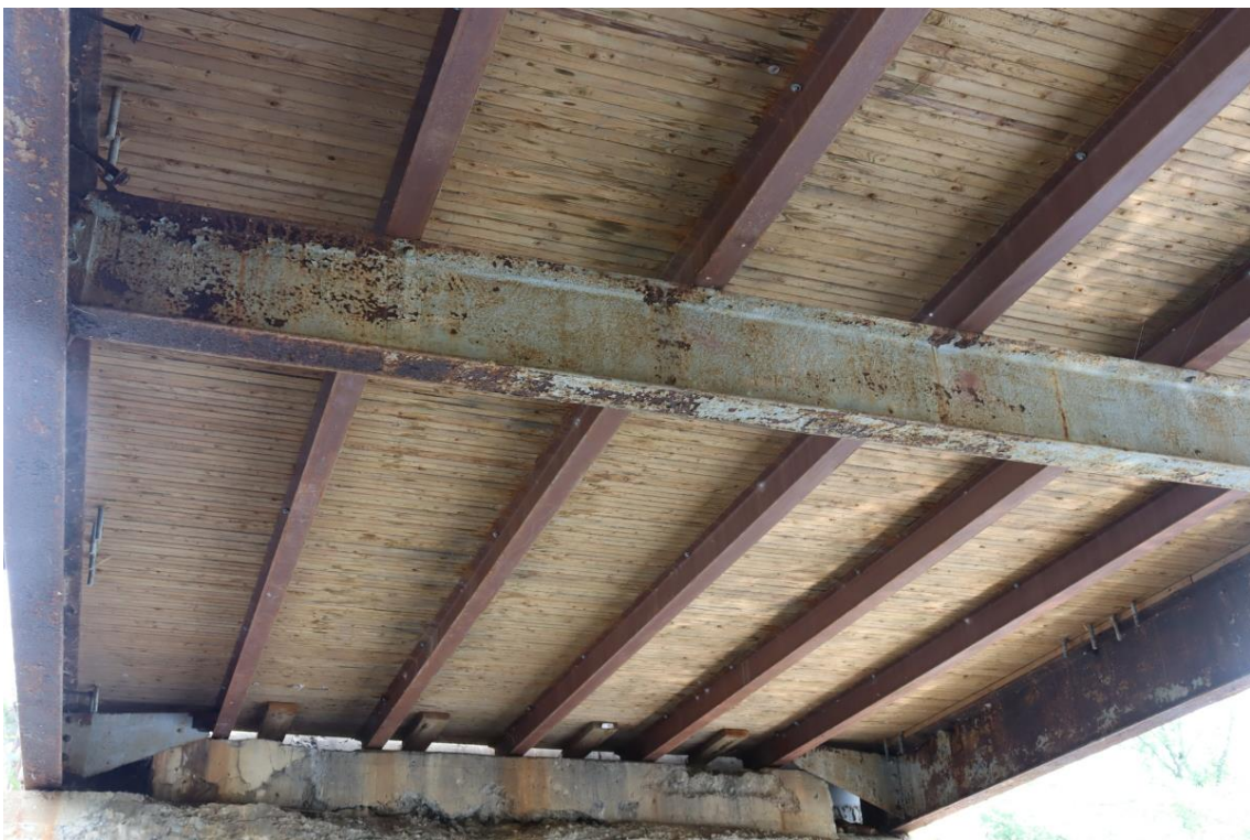
Figure 30: East span east end soffit
