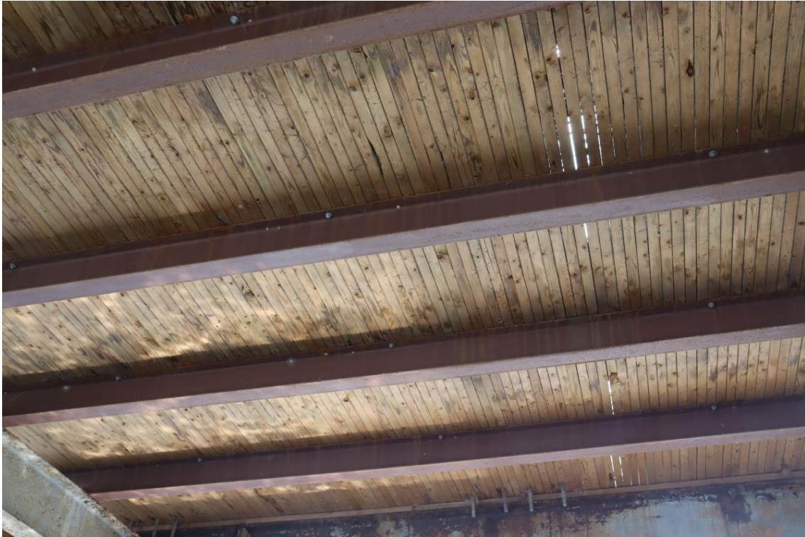
Figure 29: East span west end soffit
