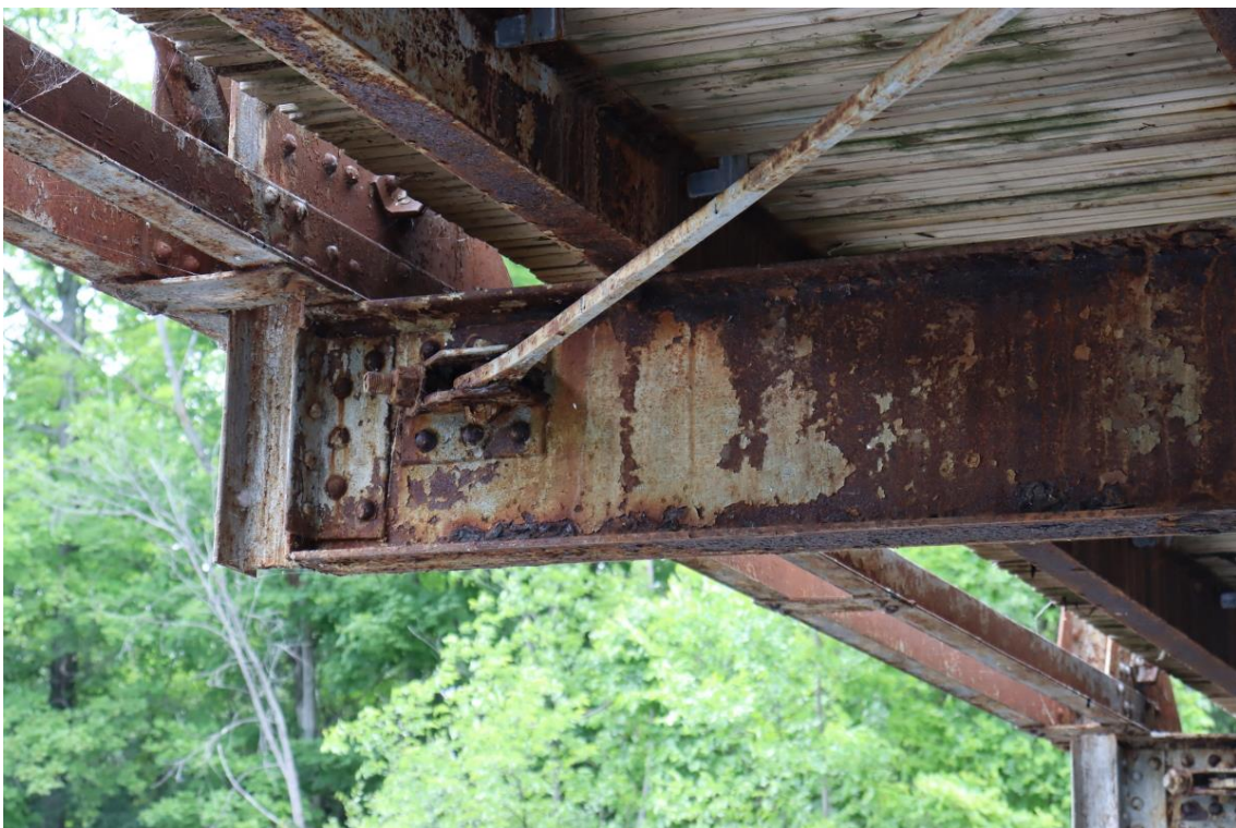
Figure 20: Floor beam 3 south end
