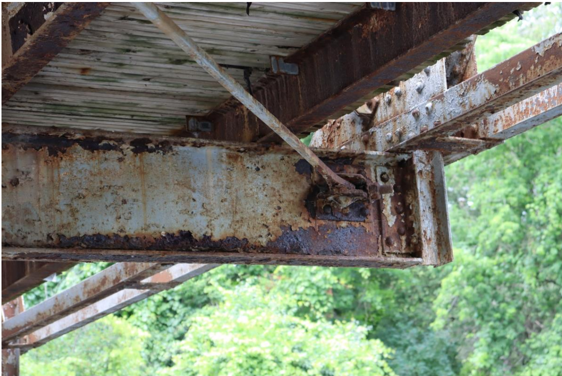
Figure 19: Floor beam 3 north end
