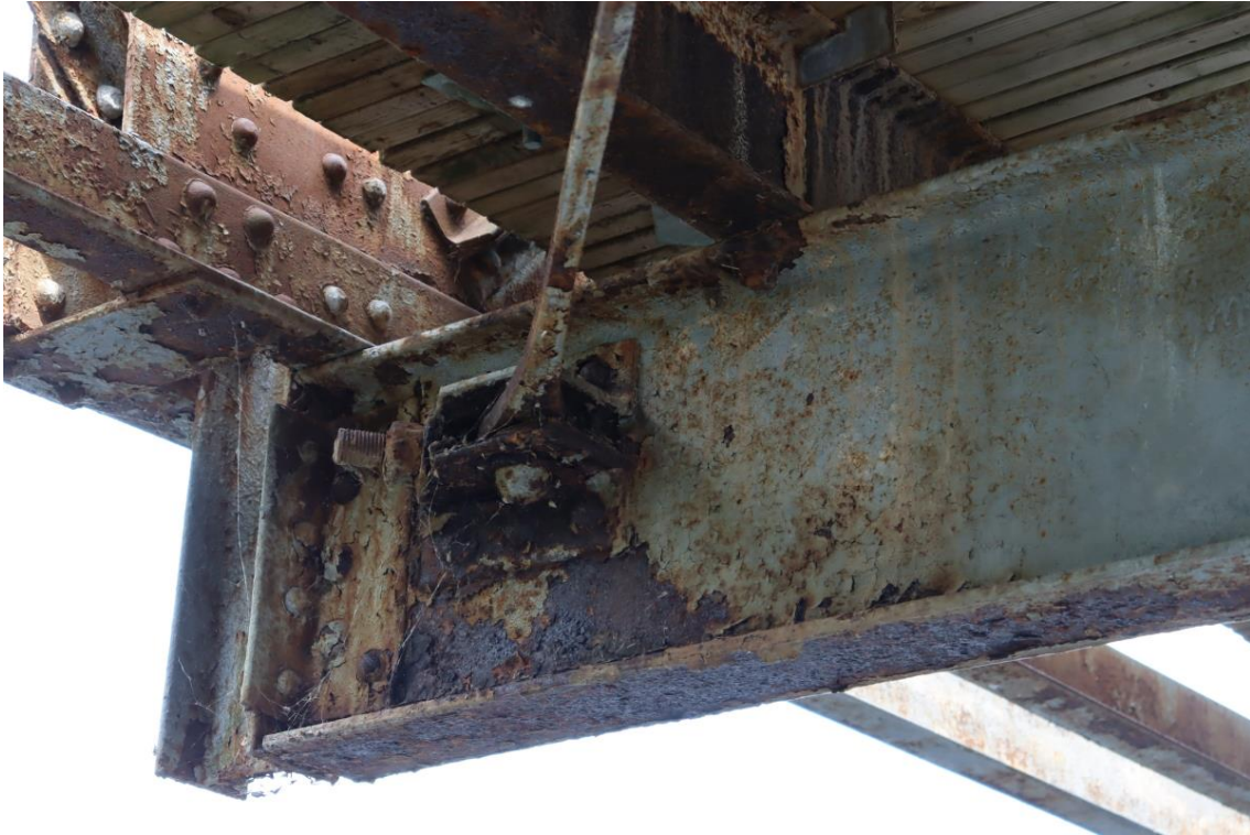
Figure 15: Floor beam 5 north end
