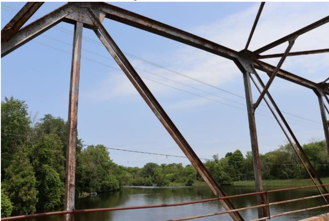
Figure 66: North truss section
