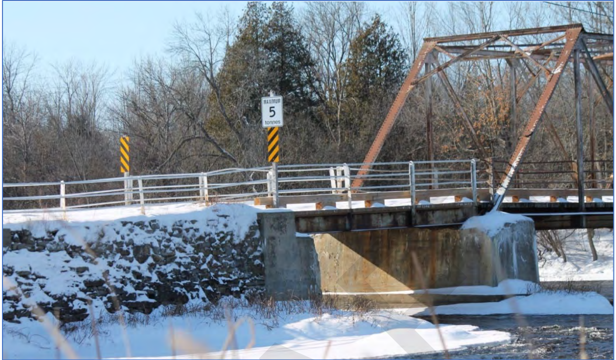
Photo 15: View southwest of dry-stone retaining wall, pier, and 9.2 m span.
