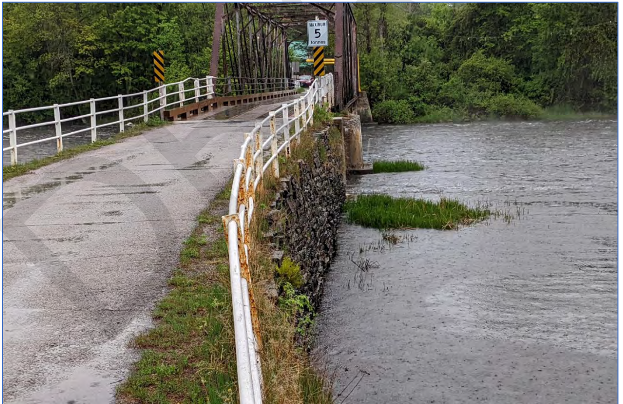
Photo 16: View west of the retaining wall and Bridge.
