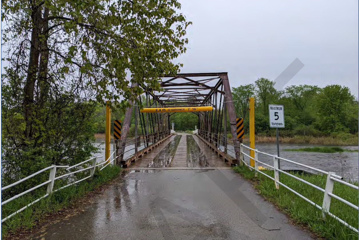
Photo 9: View east across the Bridge.
