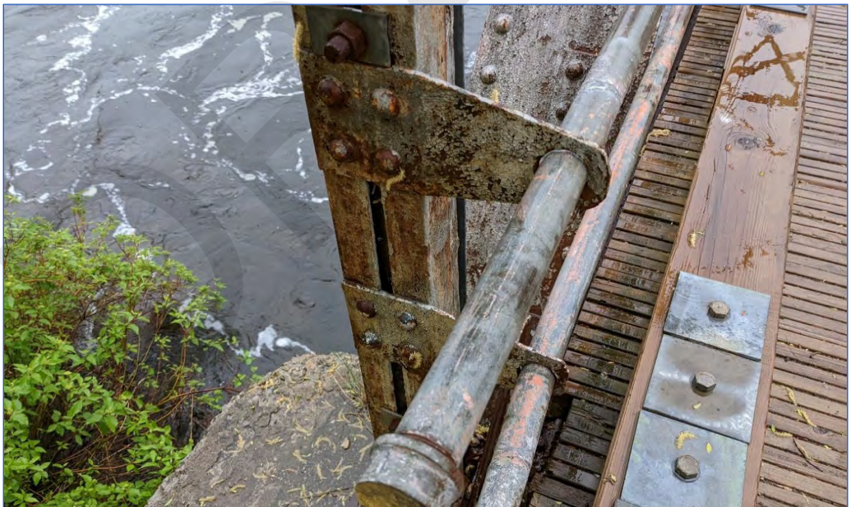
Photo 12: View of the guiderails.
