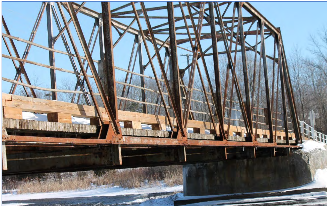
Photo 18: View east towards the Bridge substructure and east abutment.
