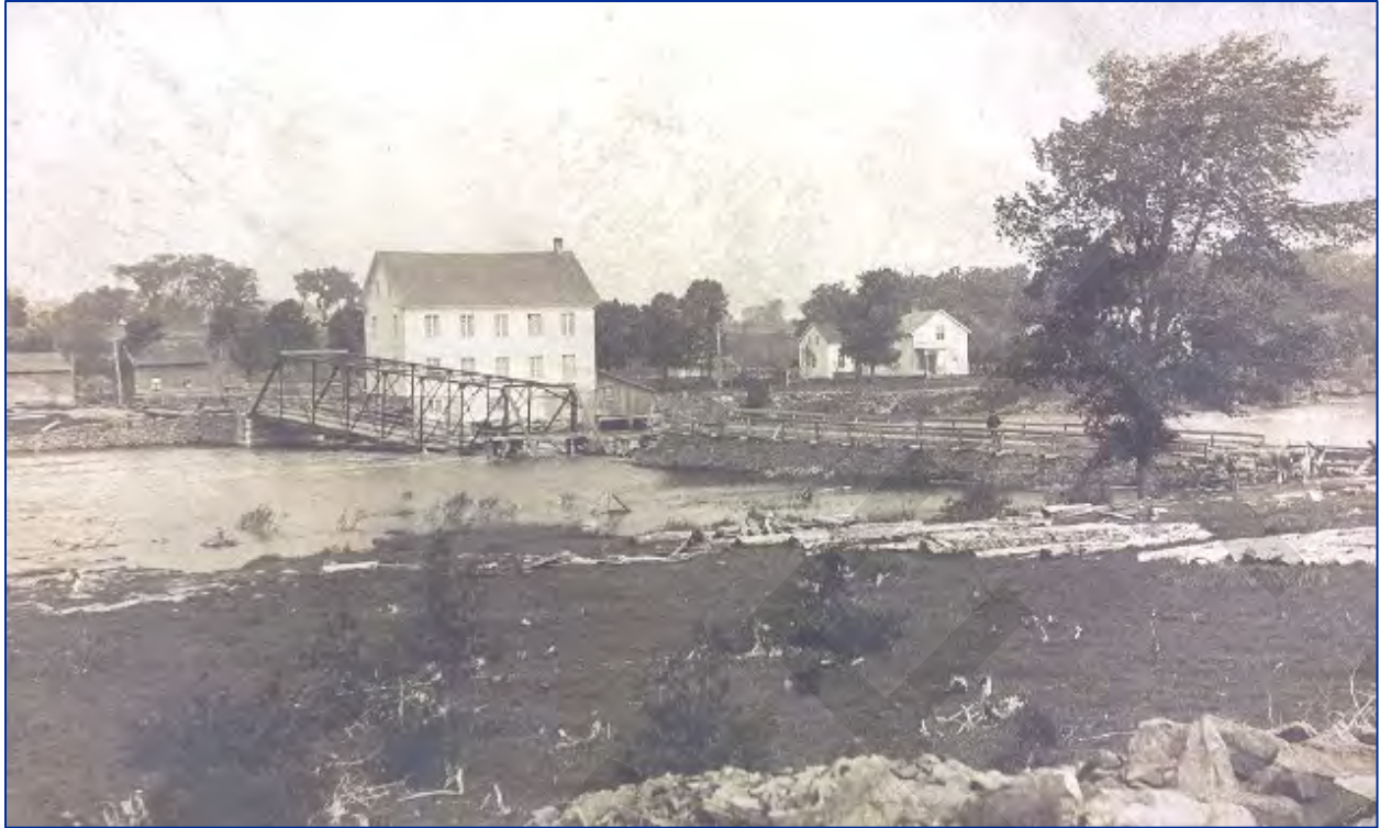
Figure 12: View of the damaged Andrewsville Bridge, 1904. 122
