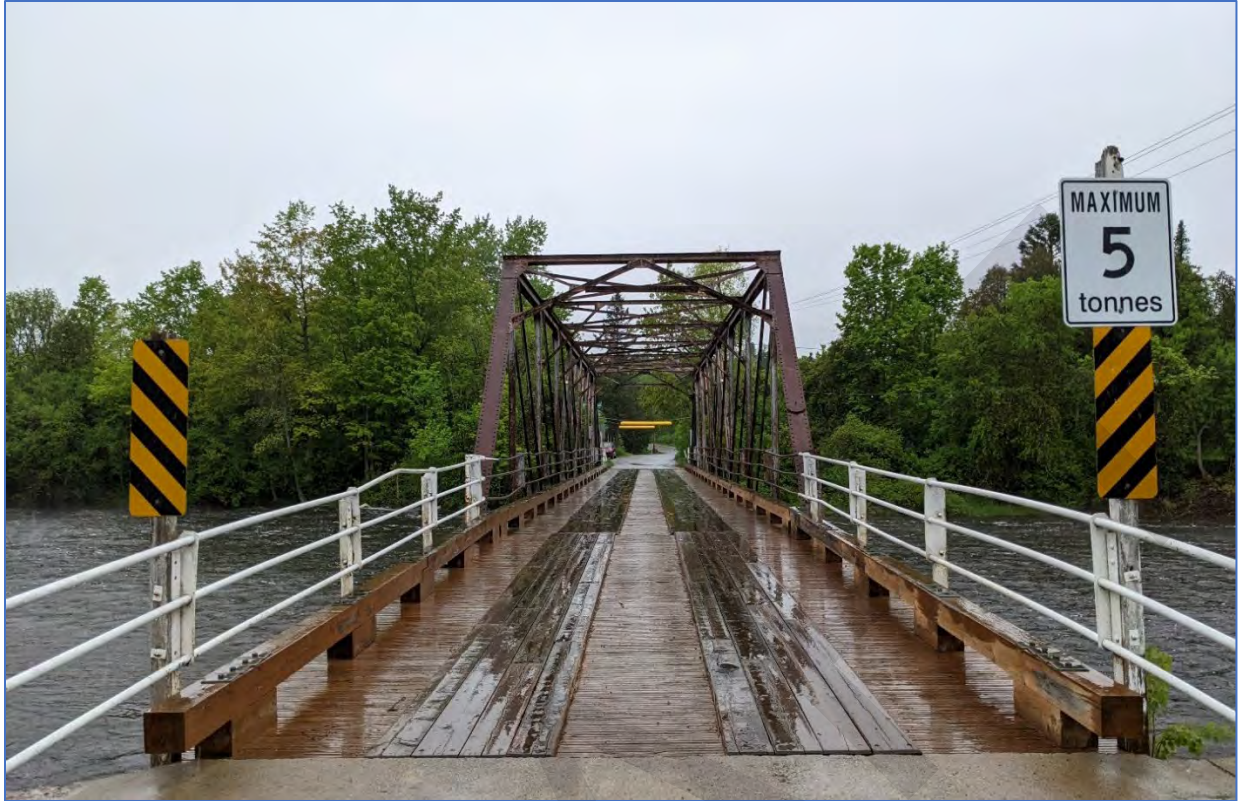
Photo 11: View west towards Andrewsville.
