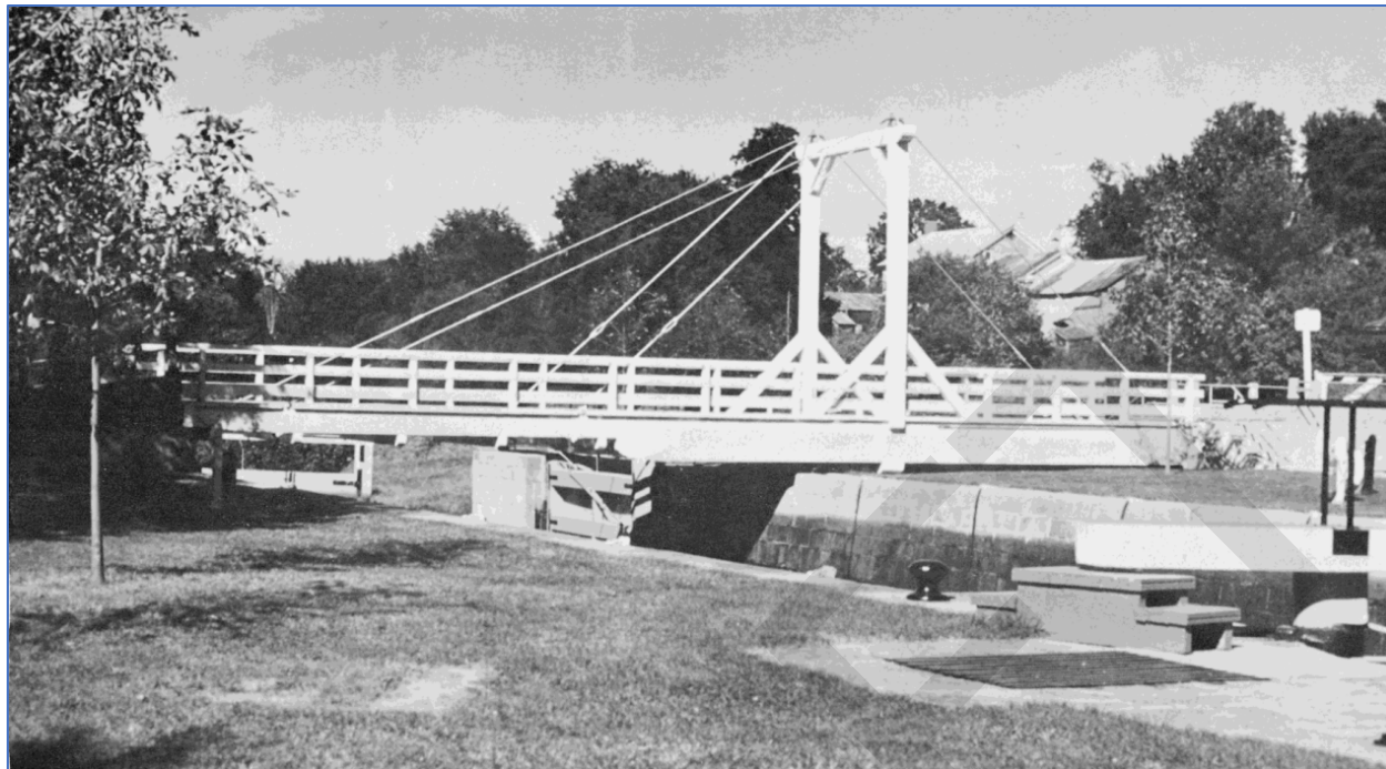
Figure 14: View of the swing bridge at Upper Nicholson's Lockstation, 1976. 124
