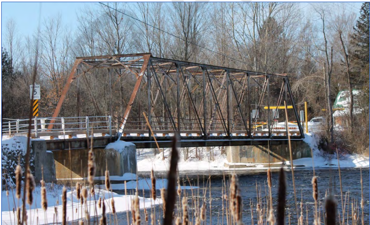
Photo 8: View southwest towards the Bridge.
