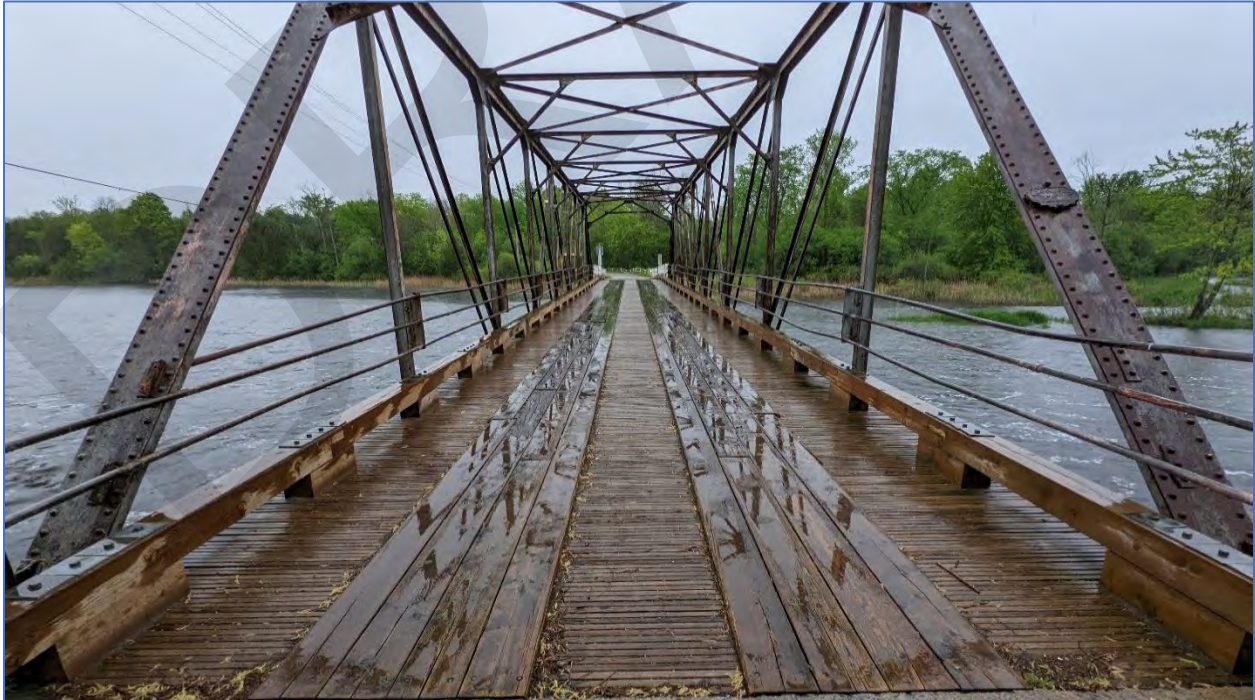
Photo 10: View east across the Bridge.
