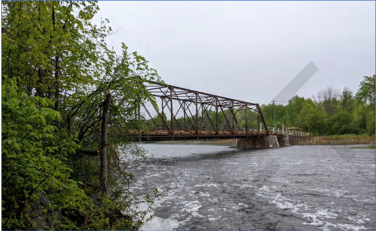
Photo 7: View north towards the Bridge.
