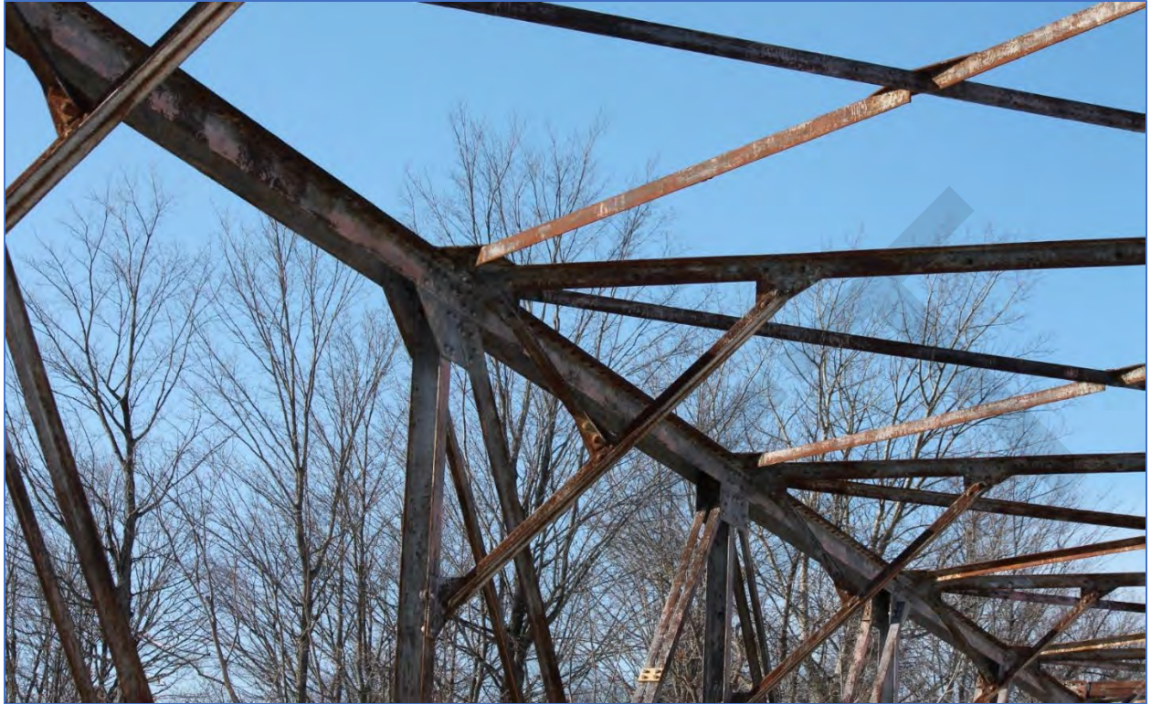
Photo 13: View of diagonal and vertical construction.
