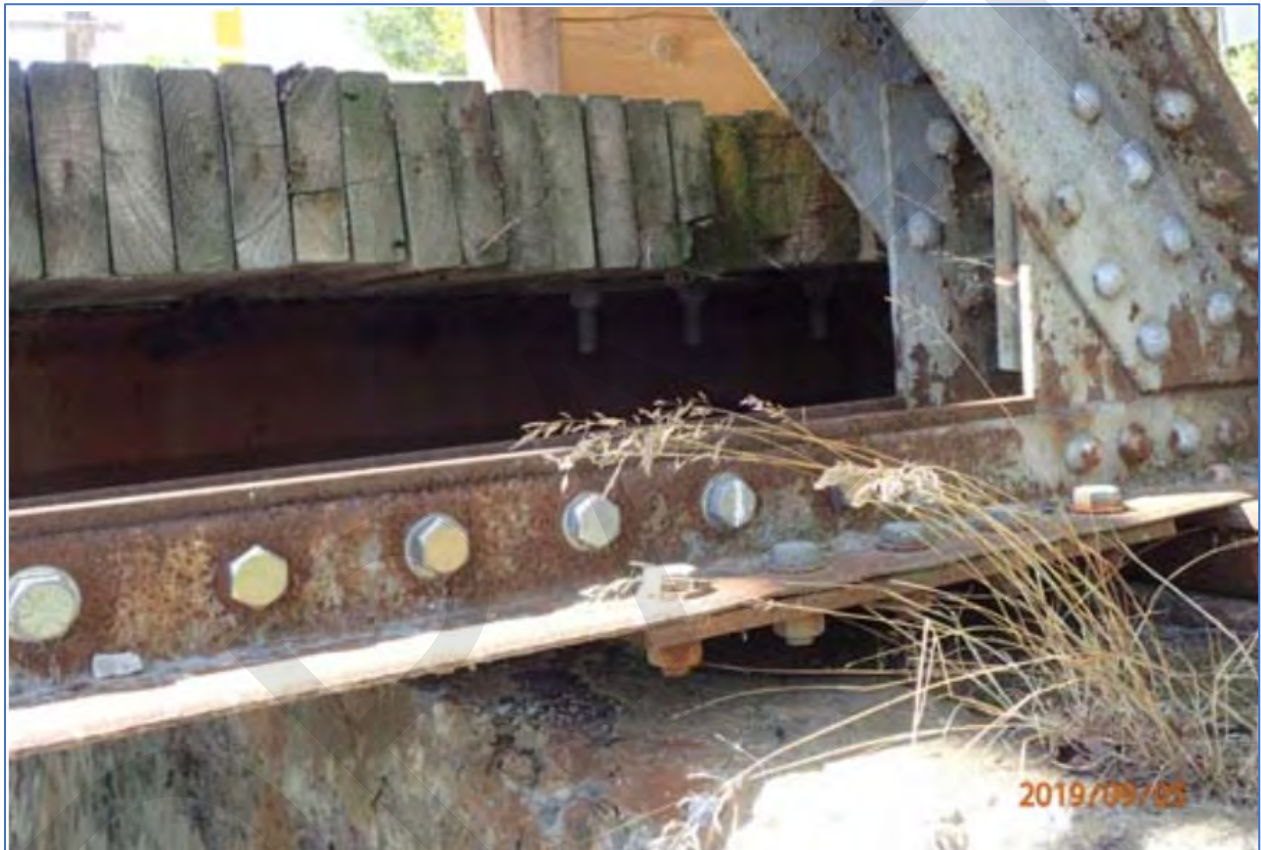
Photo 17: View of bolted stringer ends. 168
