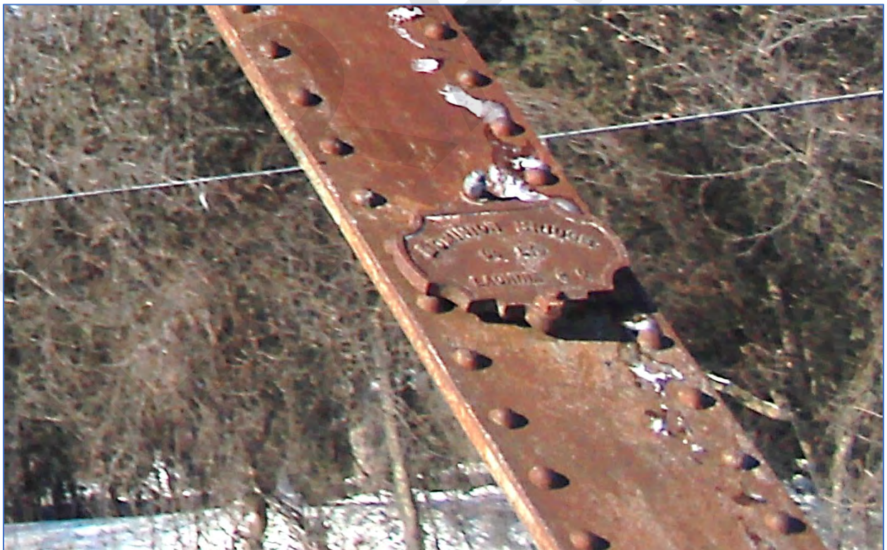
Photo 14: "Dominion Bridge Co, Ltd. Lachine. P.Q." plaque.
