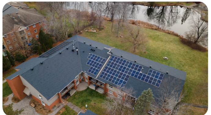
30 McGill Street, Smiths Falls Solar Panel Project
