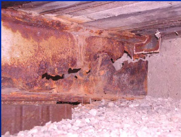
Condition of stringer, June 2005
