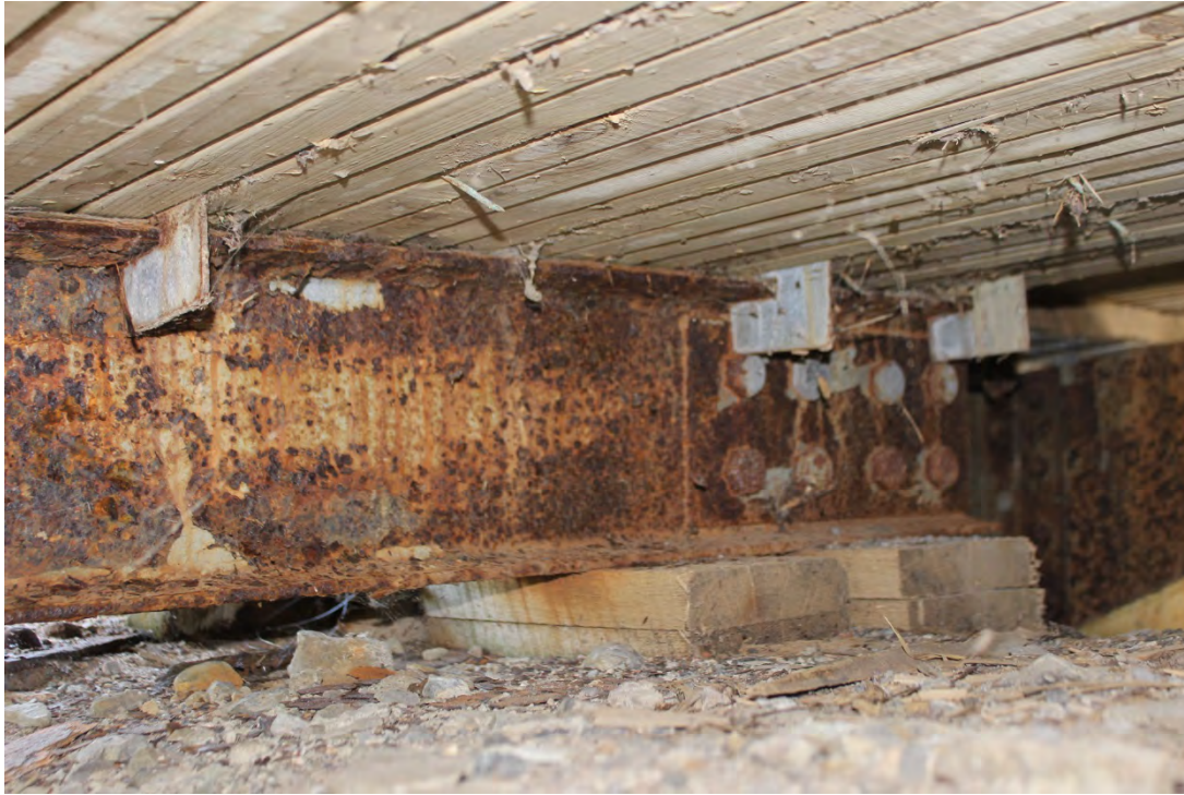
Image 11. Truss Stringer 5 at Pier Bearing
