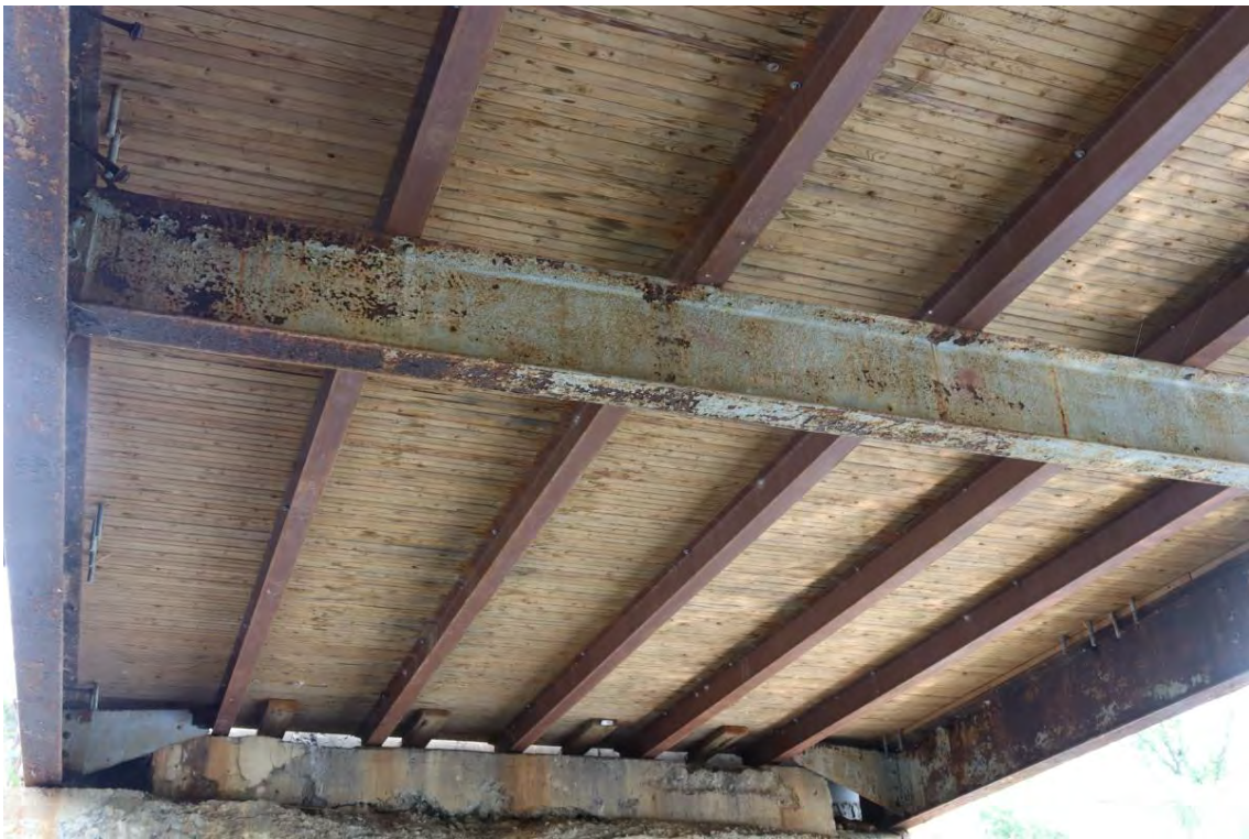
Figure 30: East span east end soffit
