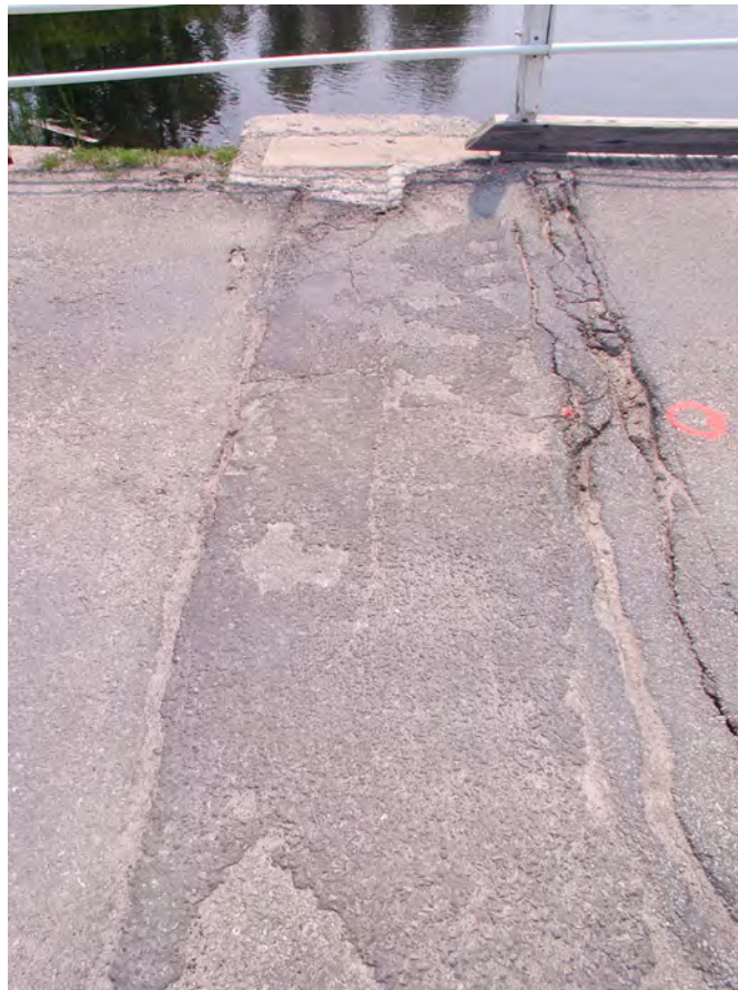
Photograph 6: East expansion joint, looking south.
