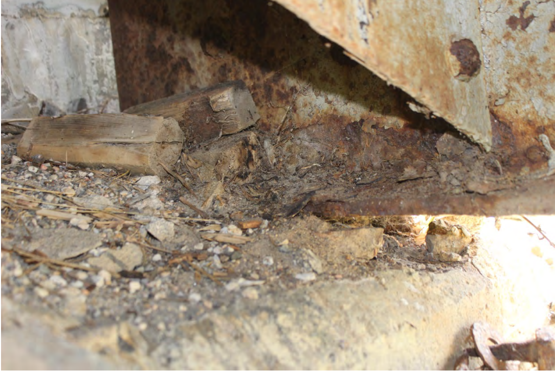
Image 31. South girder interior side bearing area at east abutment
