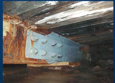
Repaired stringer, February 2006
