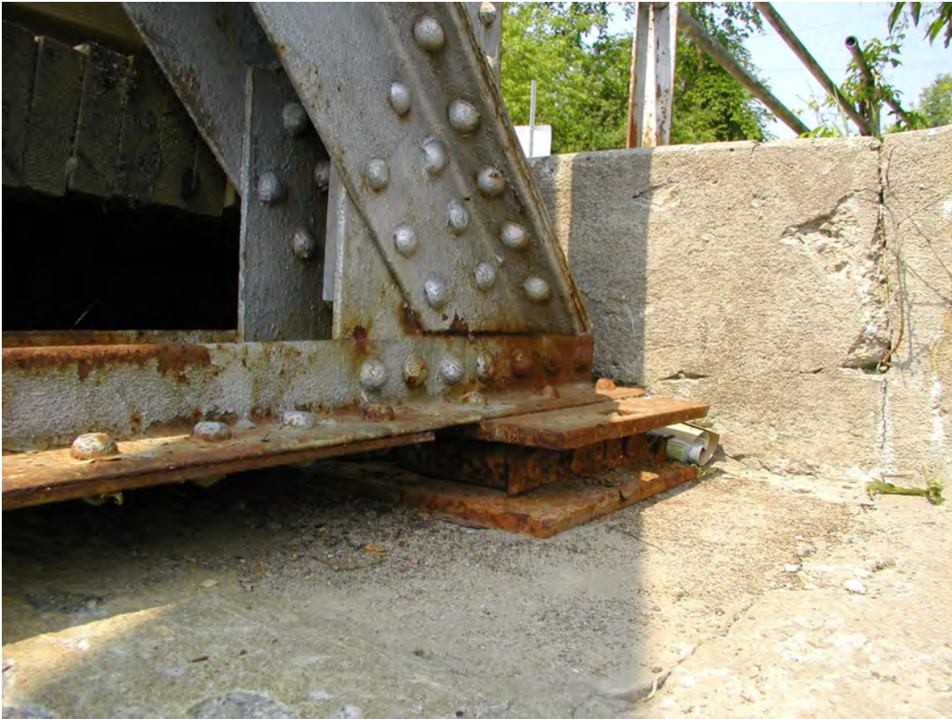
Photograph 21: Bearing configuration at West Abutment.
