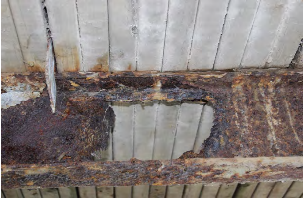
Image 13. Perforated Stringer 2 west end approach span, looking north
