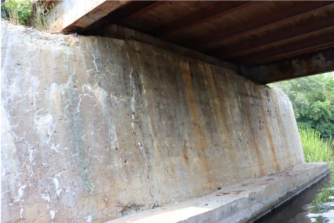
Figure 27: East face of pier
