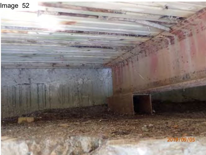
West end ballast wall & stringer
