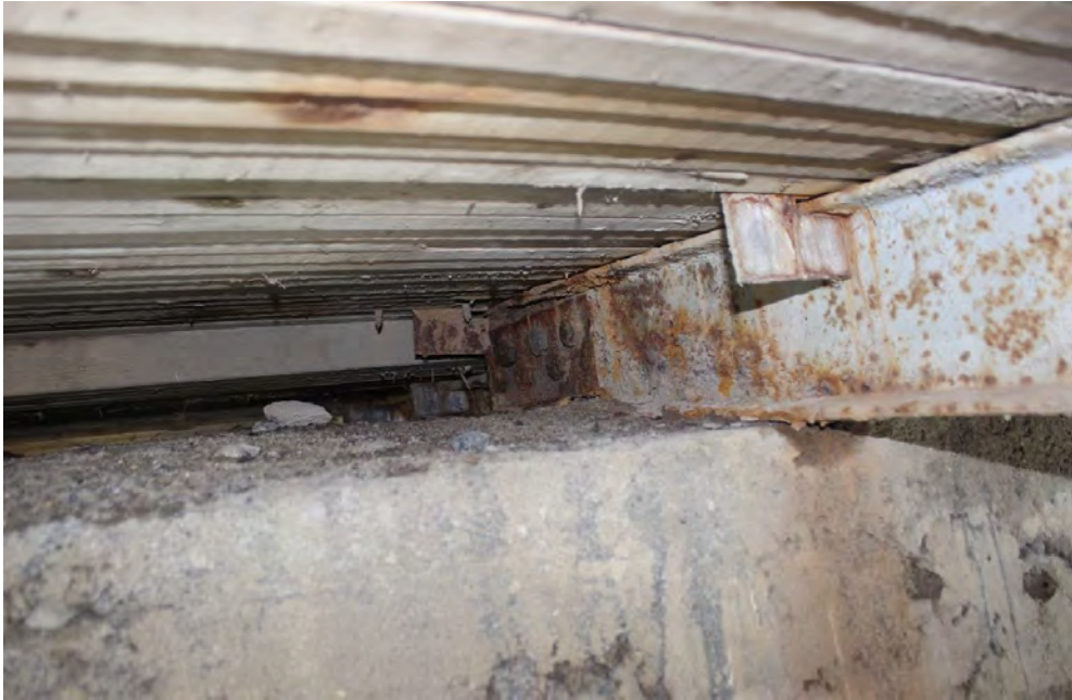
Image 17. Approach span stringer resting on east abutment
