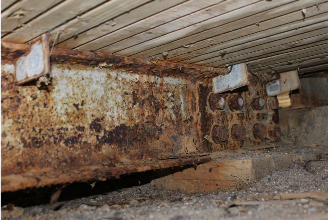
Image 9. Truss Stringer 3 at Pier Bearing
