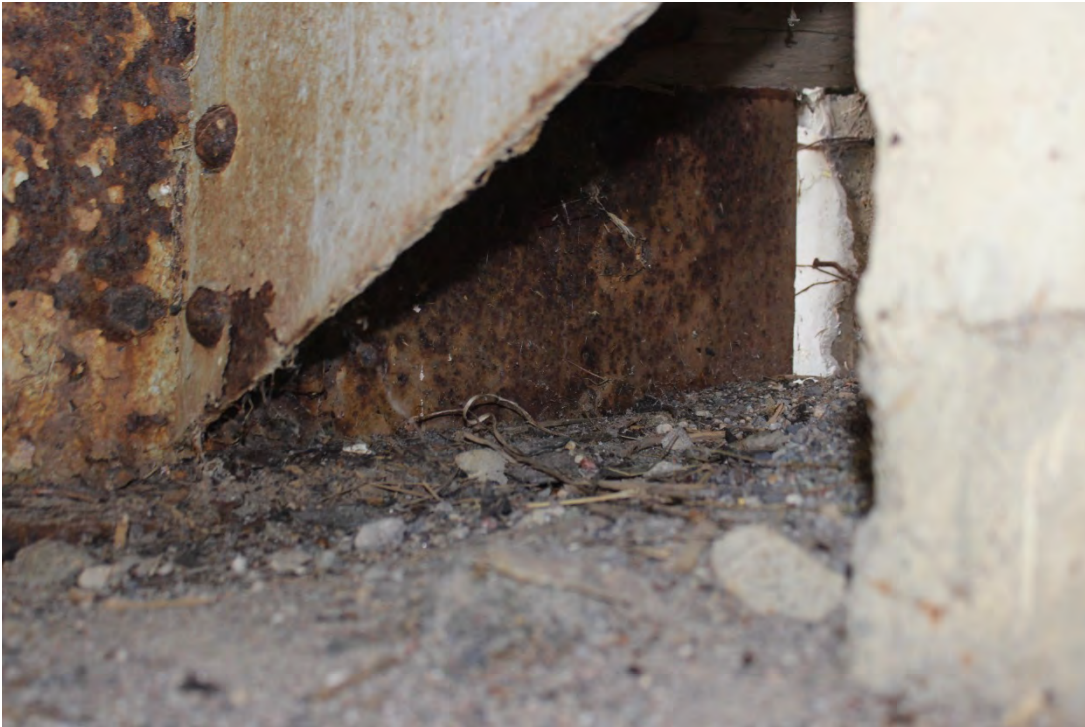
Image 32. North girder interior side bearing area at east abutment
