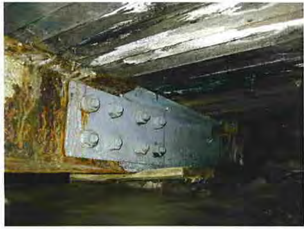
Photograph 7: Detail of repaired stringer at the West Abutment.
