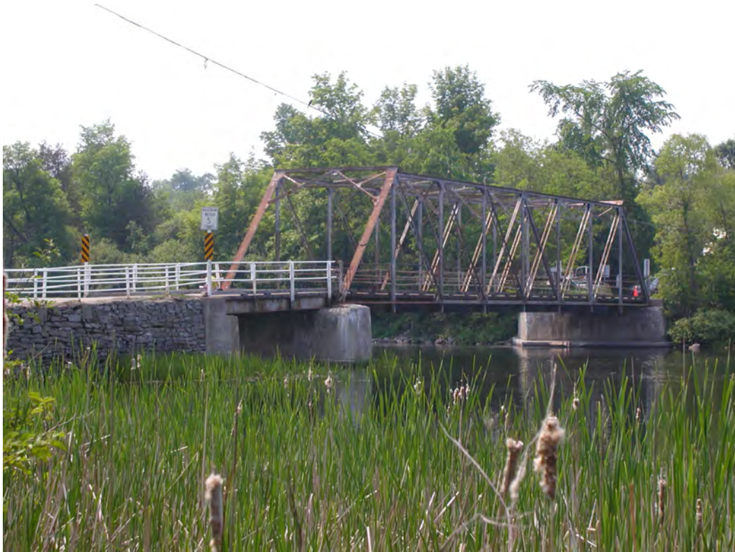
Photograph 1: North elevation of Andrewsville Bridge.
