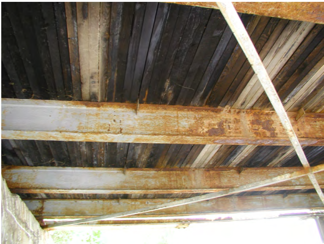
Photograph 14: View of longitudinal stringers and deck just west of pier.
