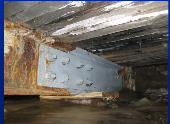
Repaired stringer, February 2006
