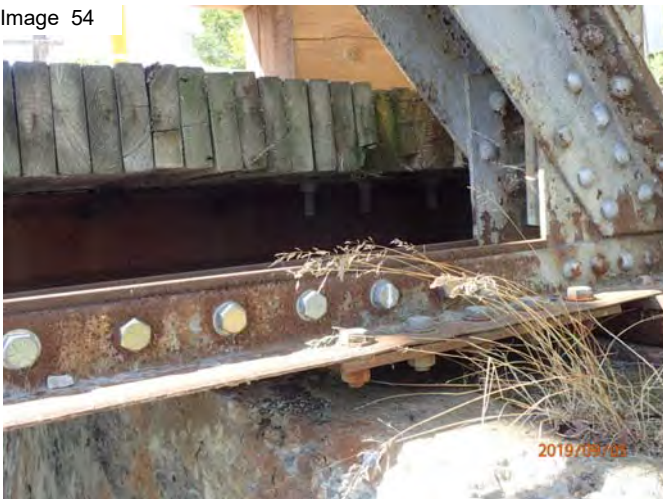
NE corner detail
