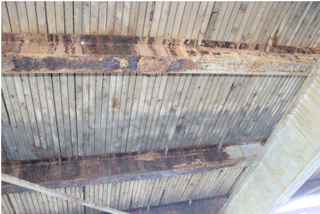
Image 2. Stringers 3 & 4 in Bay 3 looking downstream
