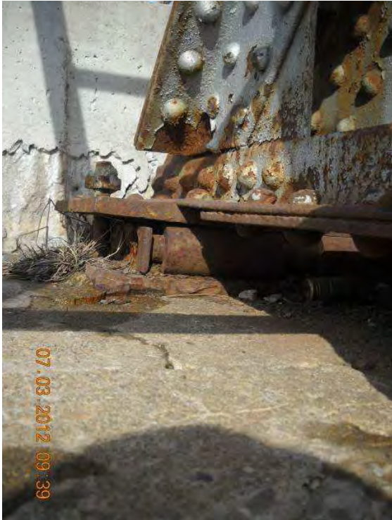
Photograph 8: Condition of truss bearing. Southeast bearing shown.
