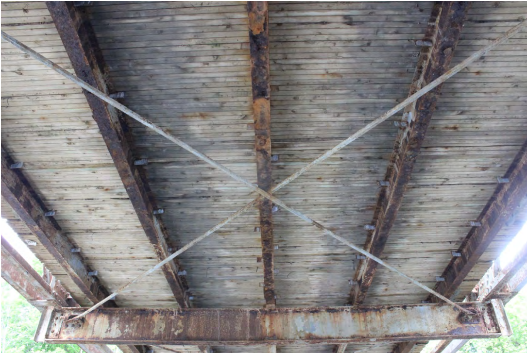
Image 20. Truss Bay 5 looking west
