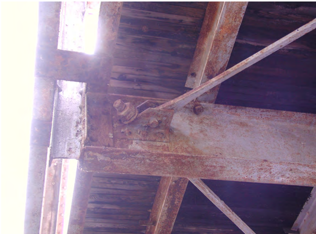
Photograph 16: Detail of cross-bracing connection at floorbeam.
