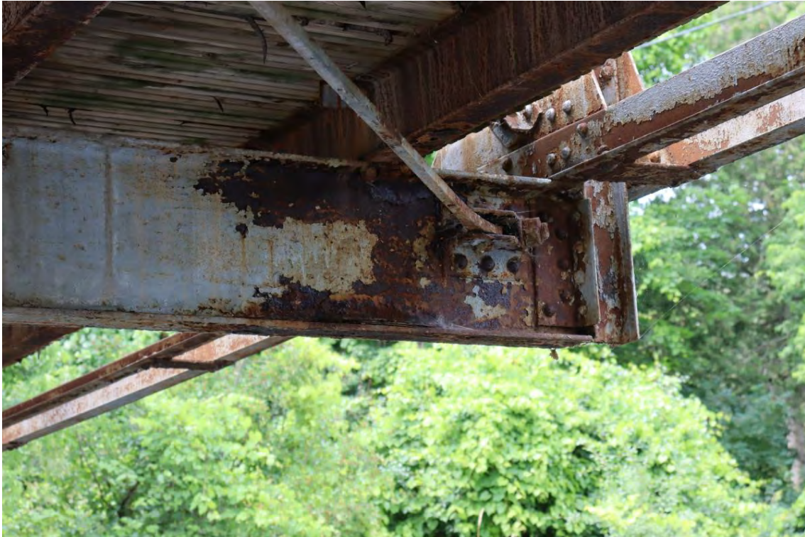
Figure 21: Floor beam 2 north end
