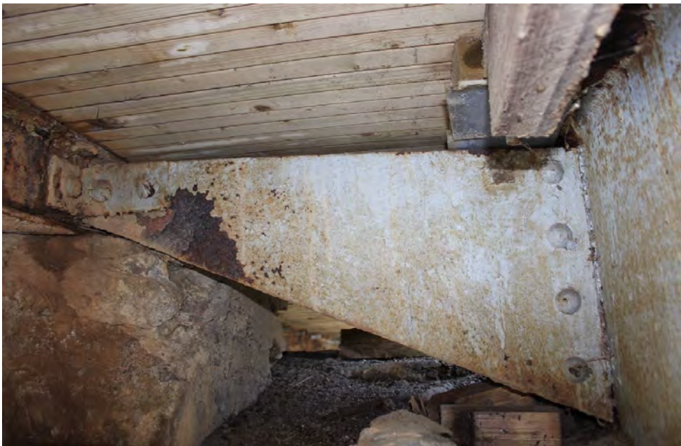
Image 18. Outrigger attached to approach girder supporting Stringer 5 at pier
