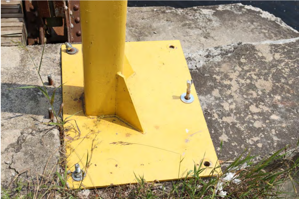
Figure 41: SW portal base
