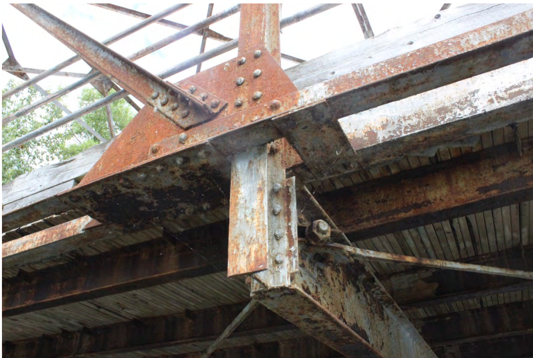
Image 24. South bottom chord between Bays 6 and 7. (Typical condition)
