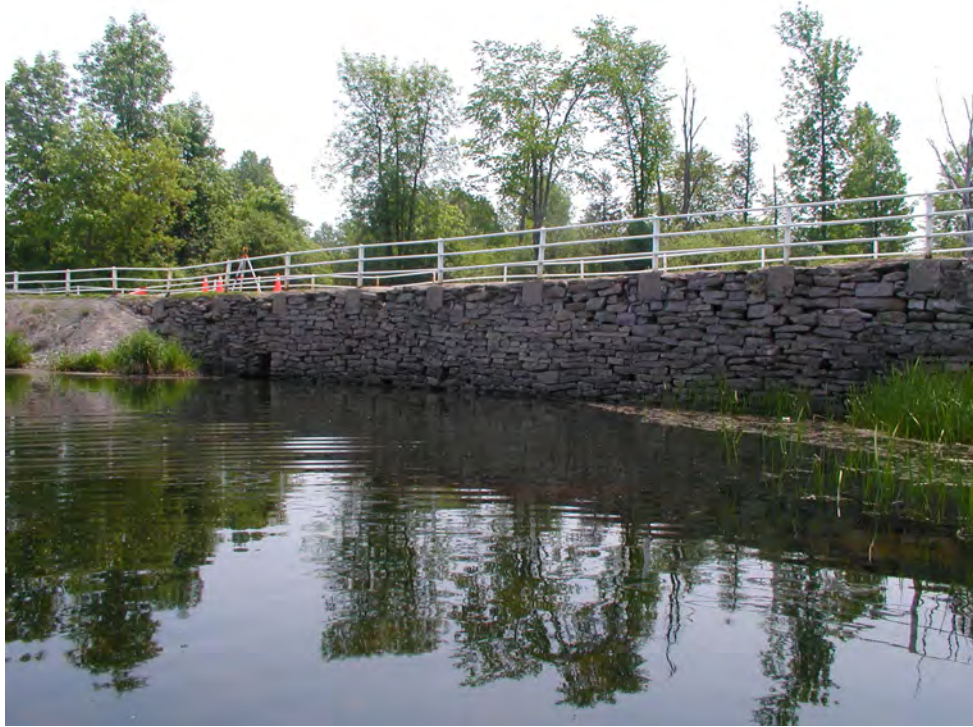
Photograph 3: North elevation of east stone retaining wall.
