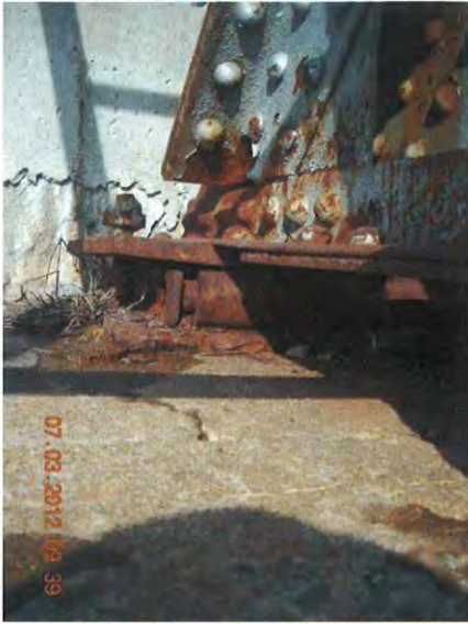
Photograph 8: Condition of truss bearing. Southeast bearing shown.
