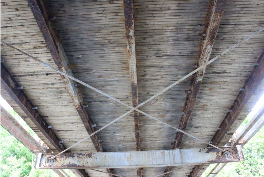
Image 21. Truss Bay 6 looking west
