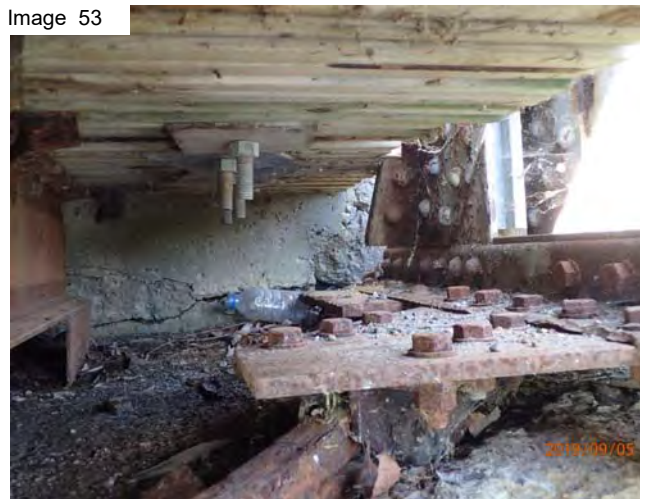
NW corner bearing
