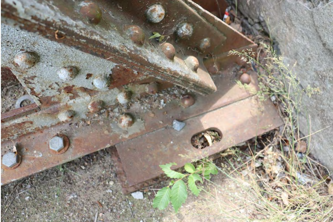
Figure 33: NW truss bearing
