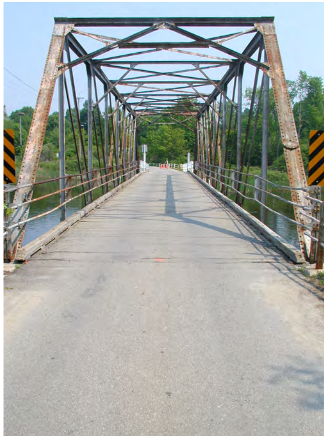
Photograph 4: View across truss span, looking east.
