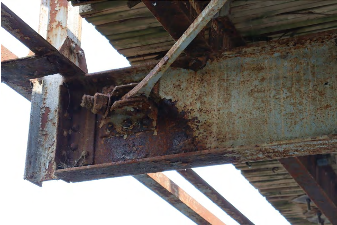
Figure 11: Floor beam 7 north end
