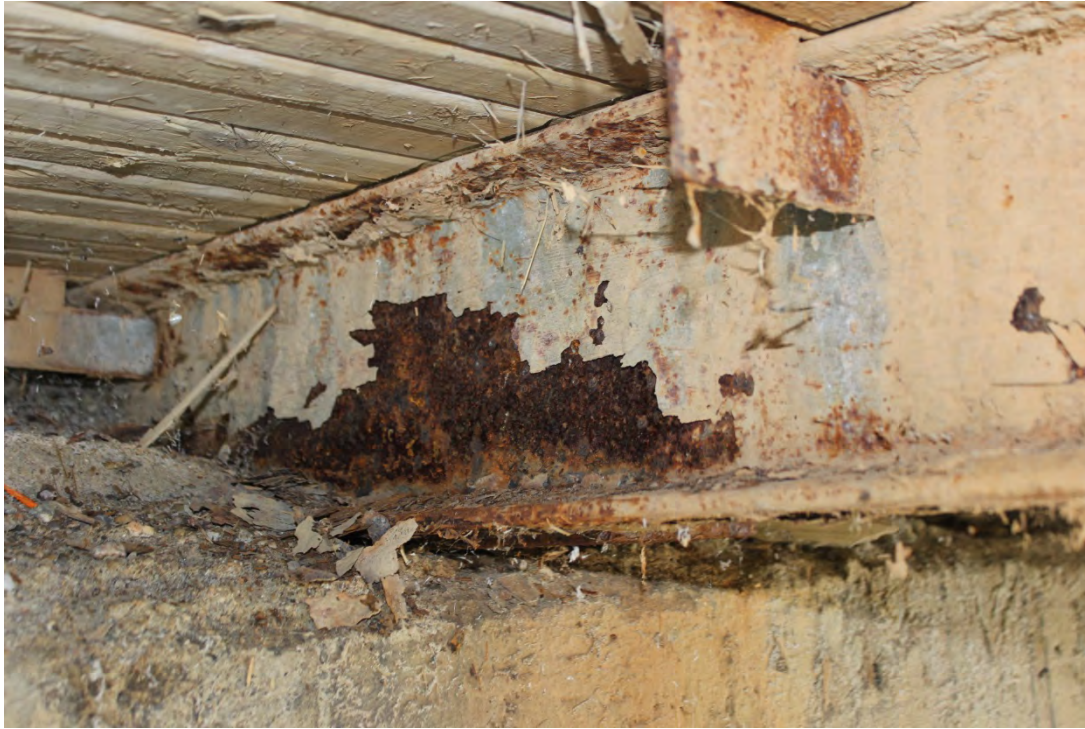
Image 27. Stringer 3 bearing area at east abutment
