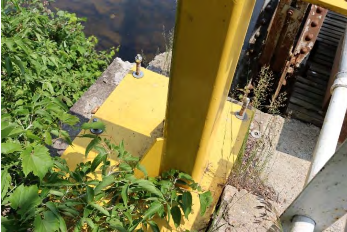
Figure 67: NW portal base
