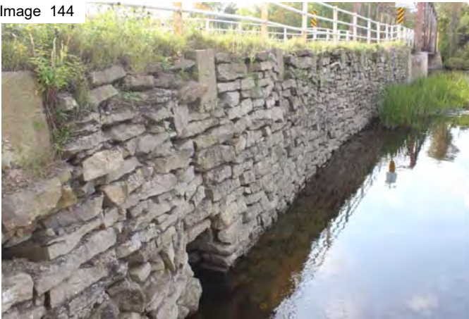
Under-cut rail post foundation SE quadrant
