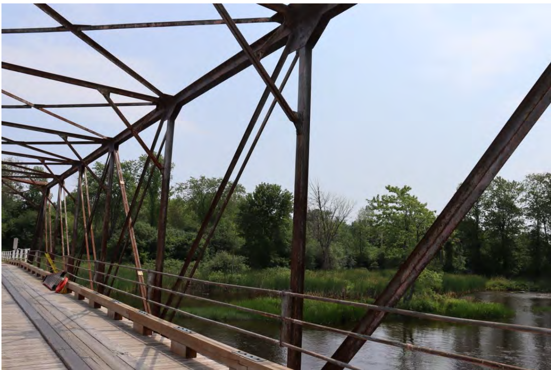
Figure 62: South side truss
