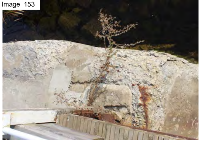
Disintegrating south abutment west side
