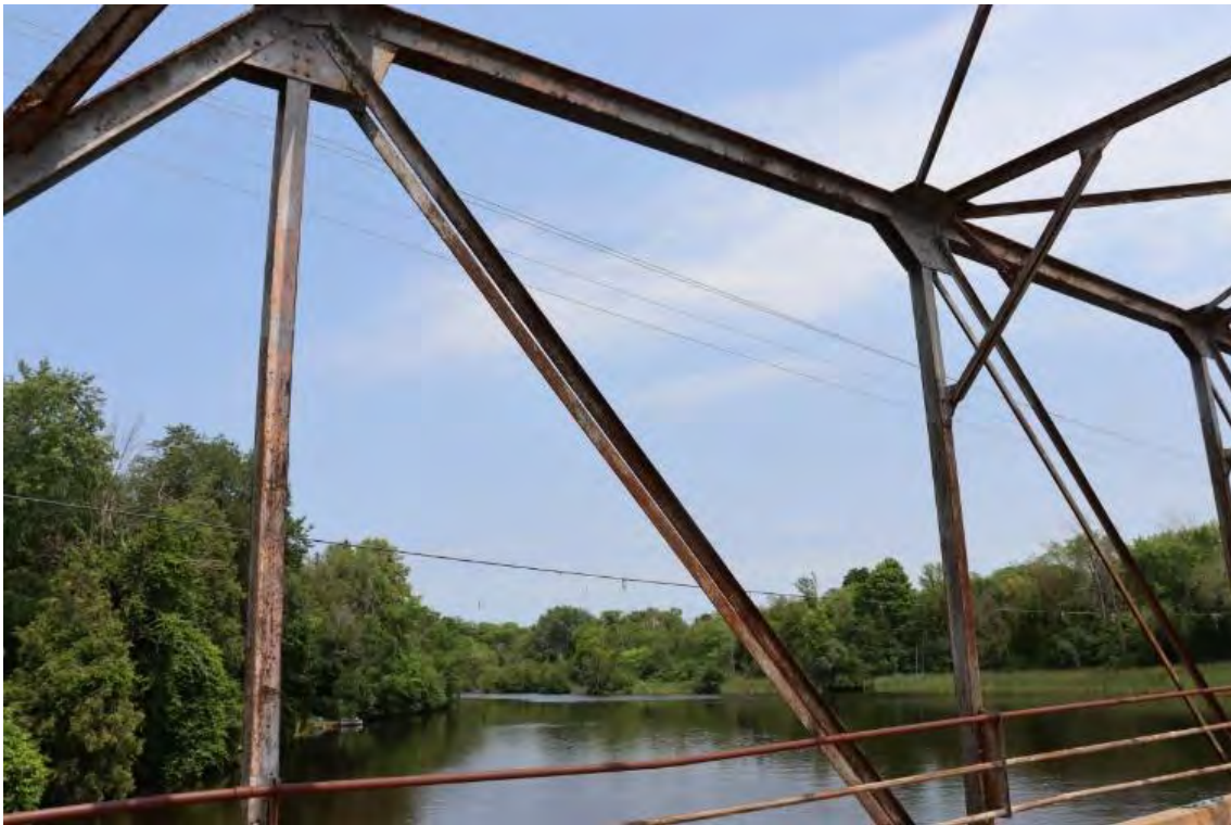
Figure 66: North truss section
