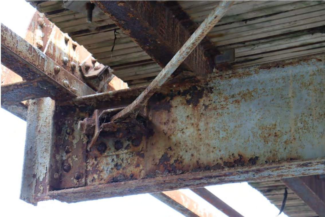
Figure 13: Floor beam 6 north end
