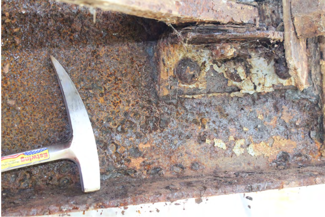
Image 3. South end of Floor Beam between Bays 1 & 2.
