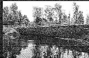
Single span slab-on-girder
