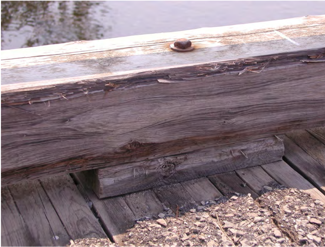
Photograph 33: Detail of curb on timber deck.
