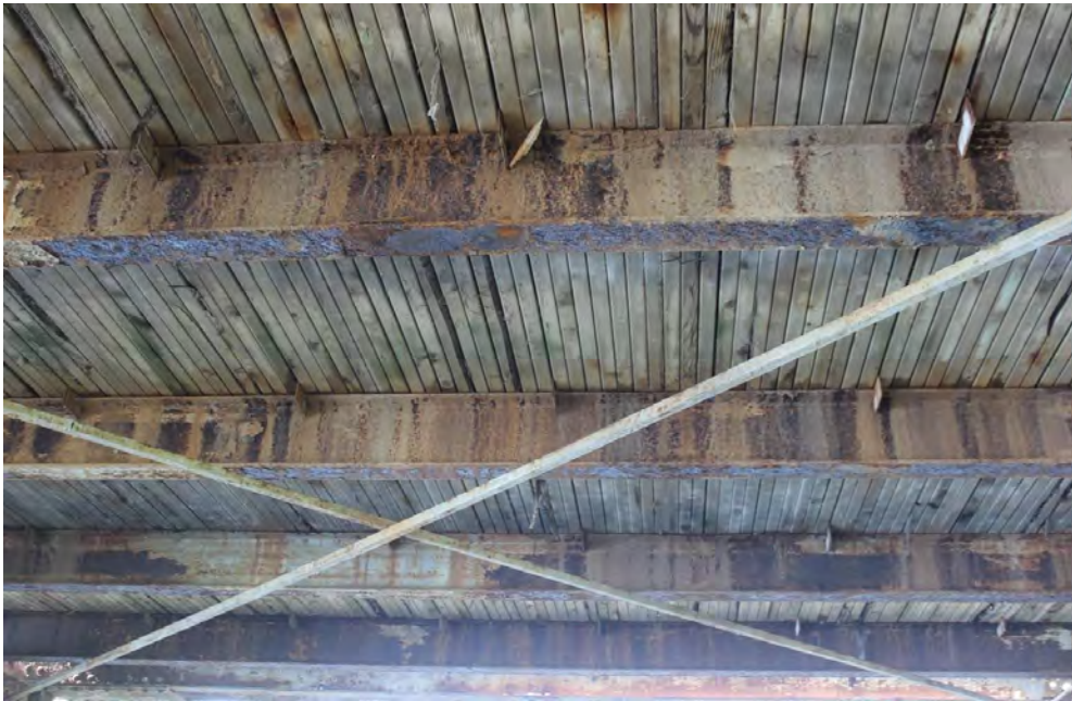
Image 4. Bay 3 looking south, Stringers 4,3,2,1 visible
