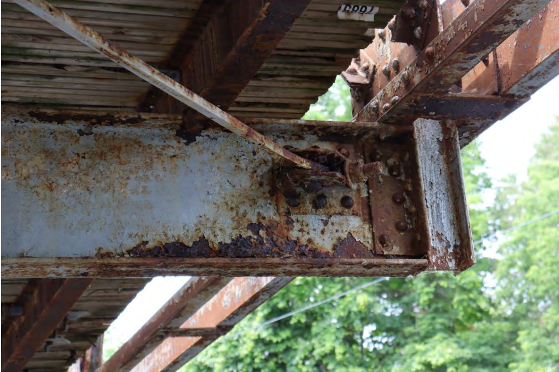
Figure 17: Floor beam 4 north end
