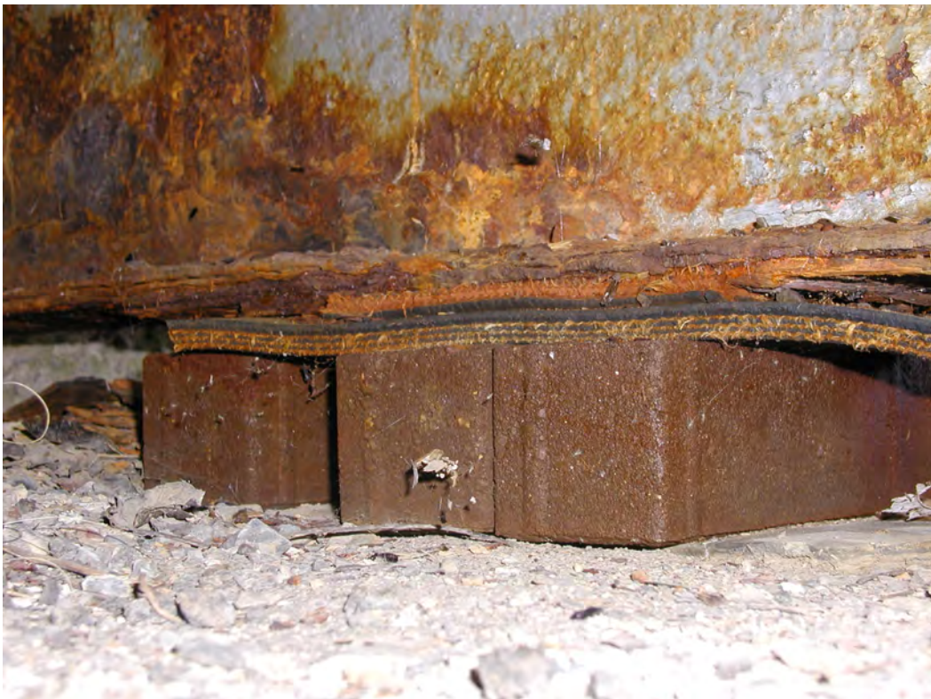
Photograph 24: Detail of bearing pads on interior girders, East and West Abutments.
