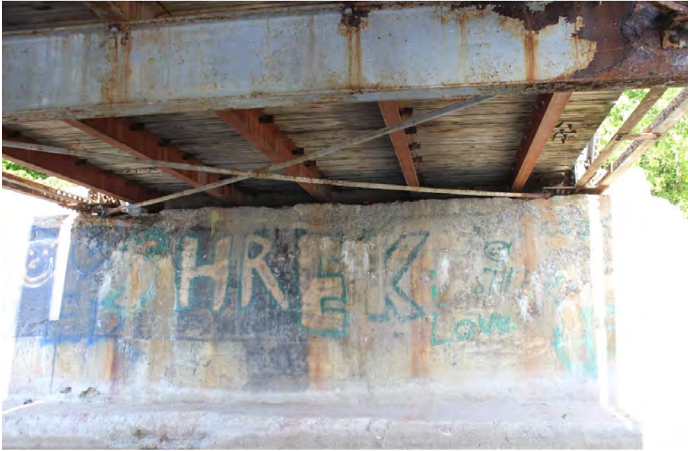
Image 1. West abutment and replaced Bay 1 stringers, Floor Beam 1 in foreground.
