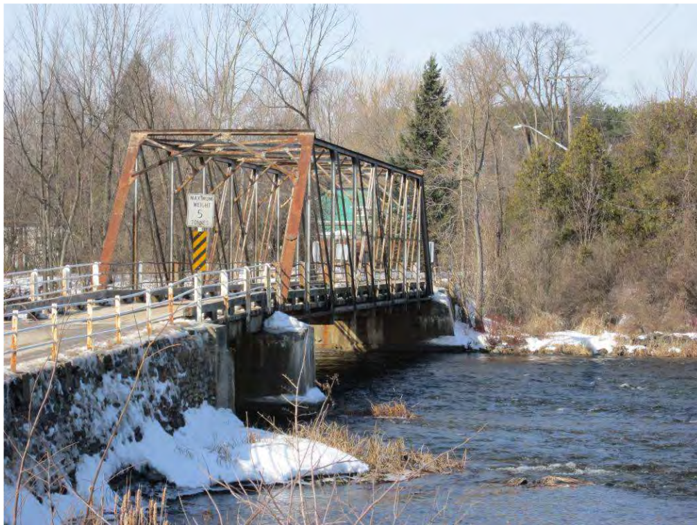
Photograph 1: East elevation, looking northwest.
