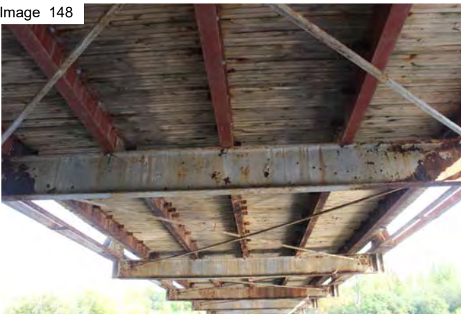
Curb timber decay on truss
