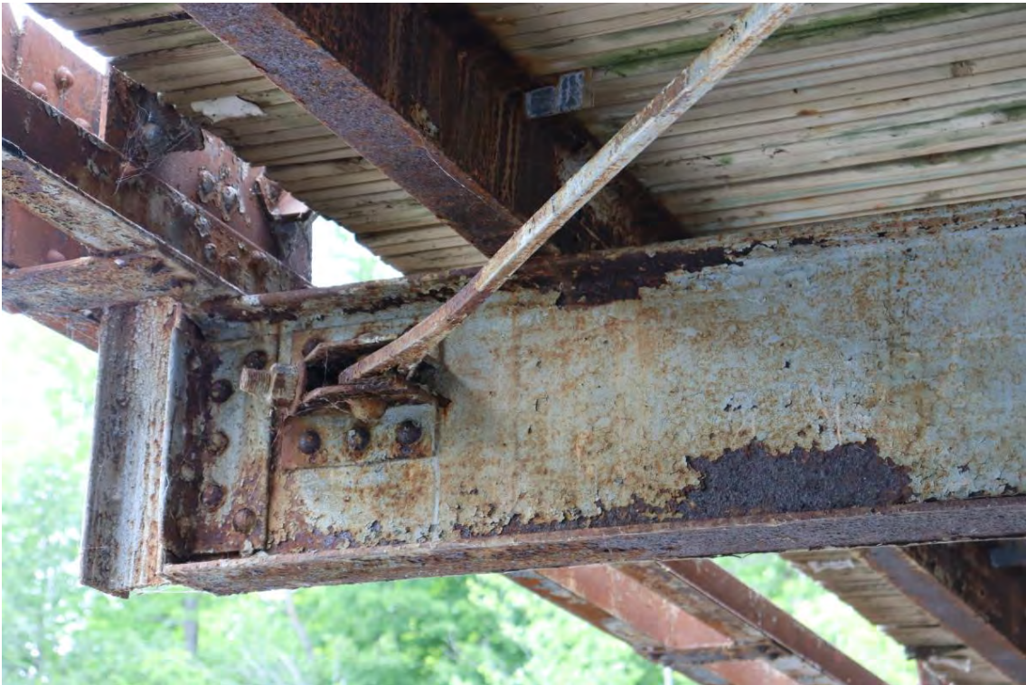
Figure 18: Floor beam 4 south end
