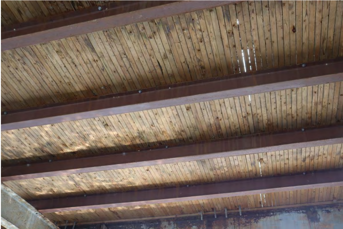
Figure 29: East span west end soffit
