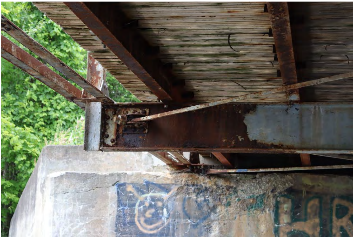
Figure 24: Floor beam 1 south end
