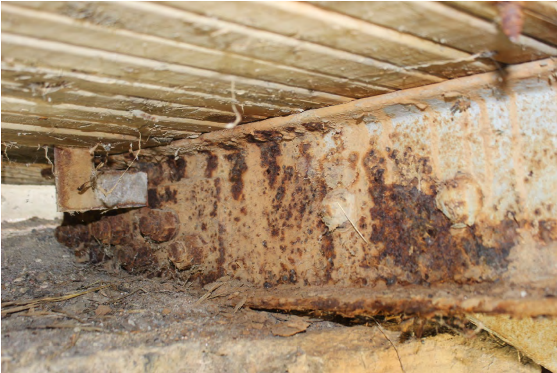
Image 30. Stringer 1 bearing area at east abutment
