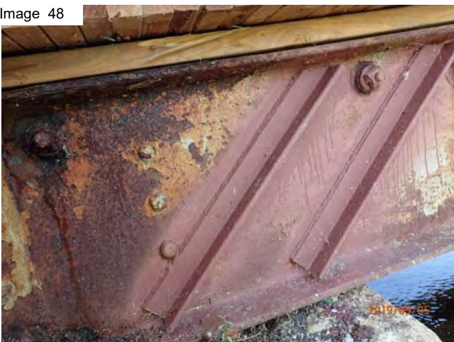
SE girder end web strengthening (2019)
