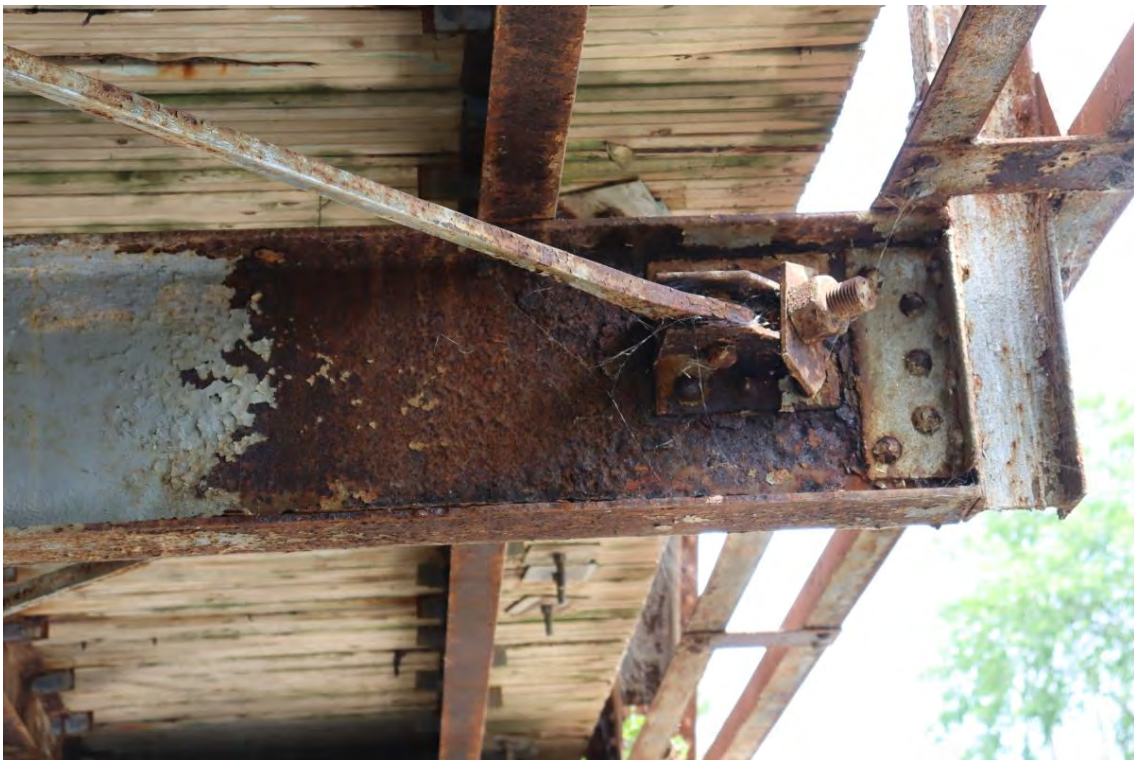
Figure 12: Floor beam 7 south end
