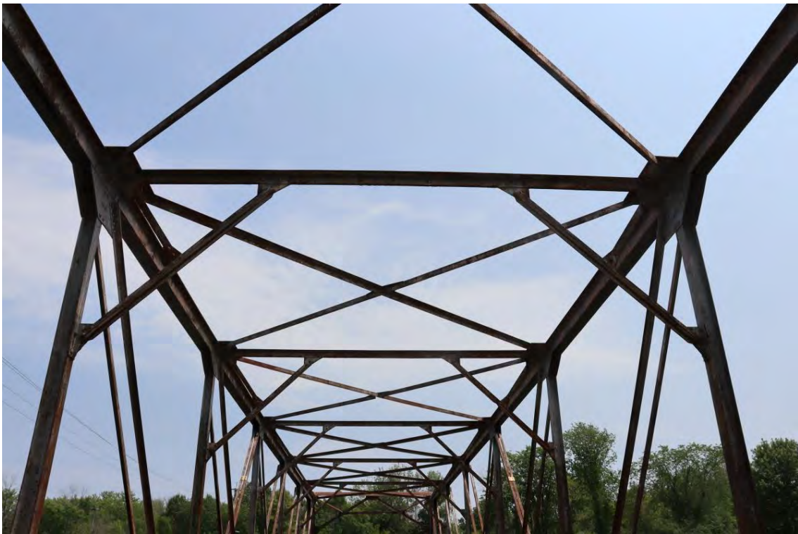
Figure 64: Wind and sway bracing
