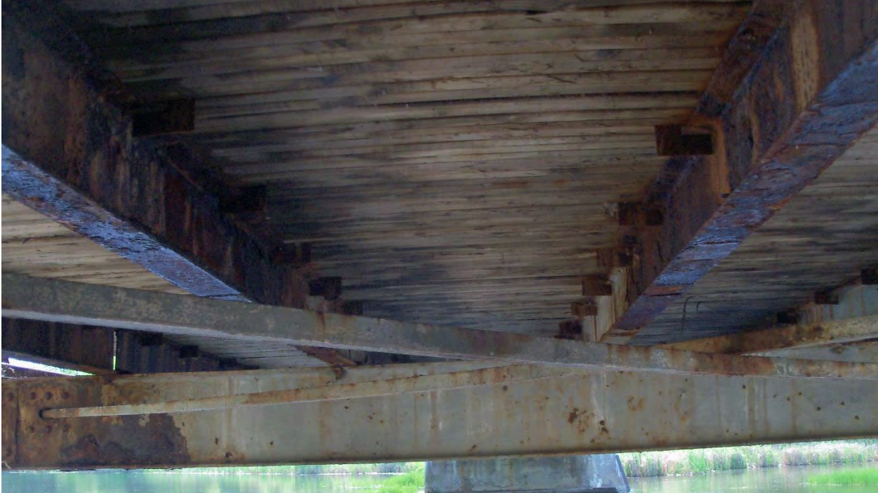
View of soffit and truss stringers and floor beams
