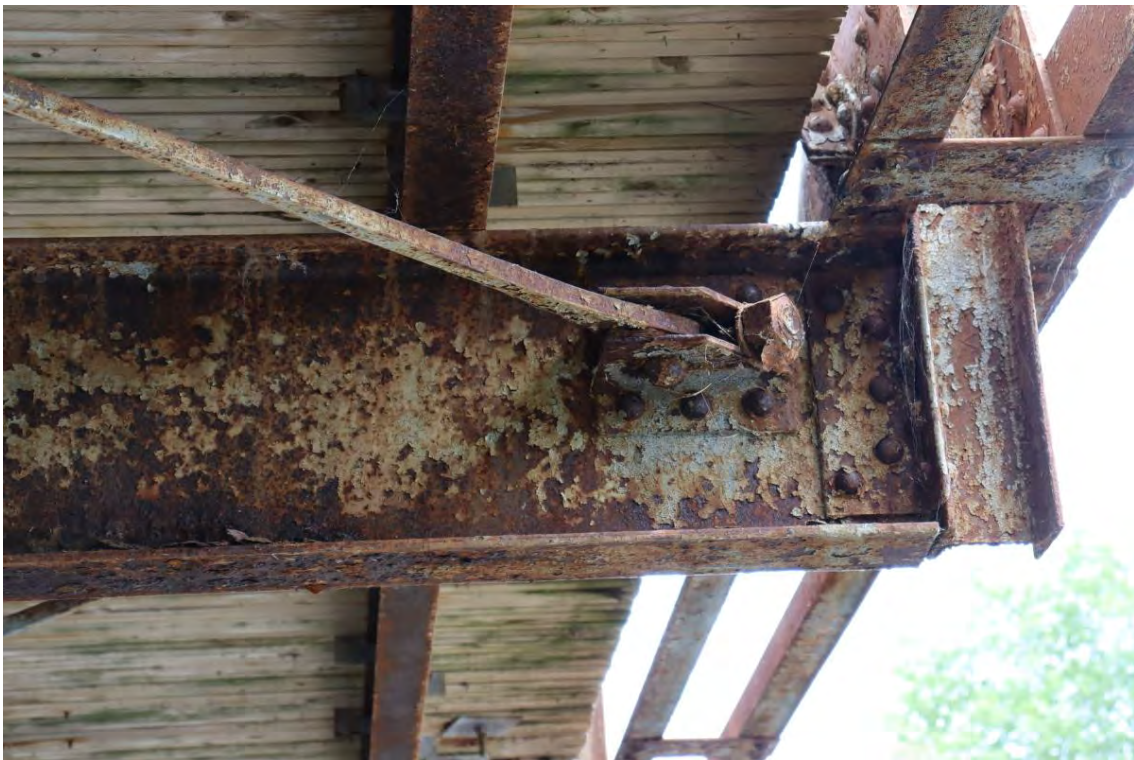
Figure 14: Floor beam 6 south end
