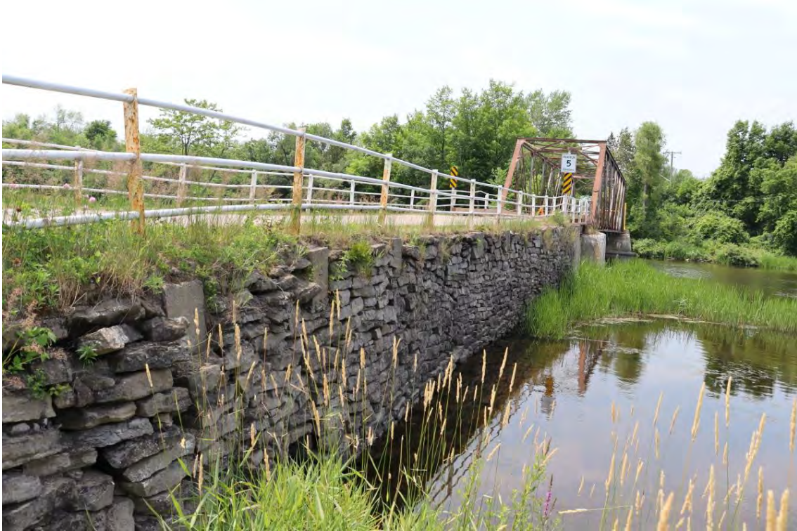
Figure 53: North dry-stone retaining wall east approach
