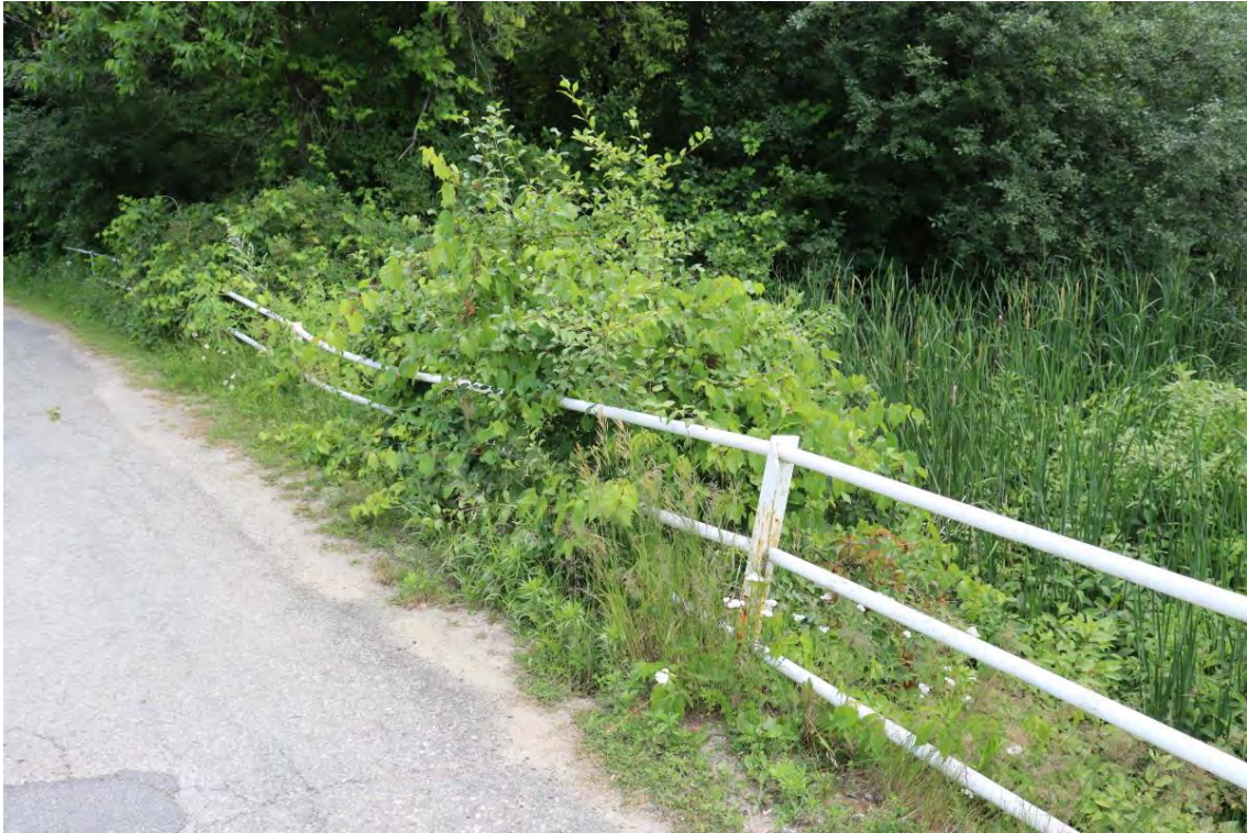
Figure 47: Railing south side of causeway
