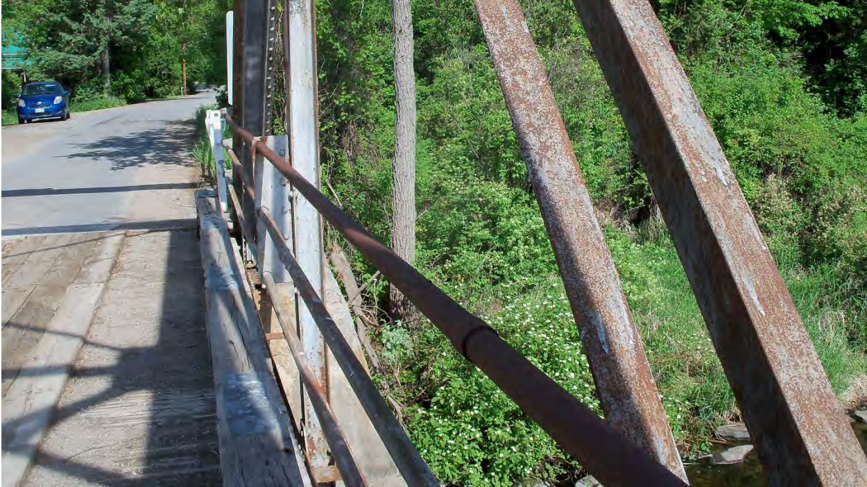
View of timber curb and railing system
