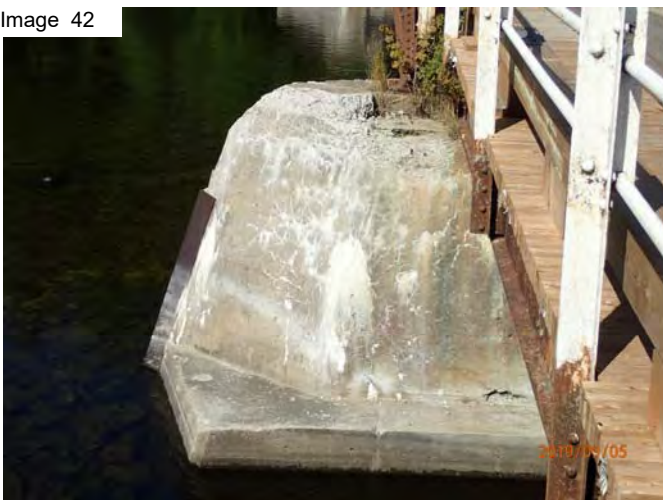
SW end of pier
