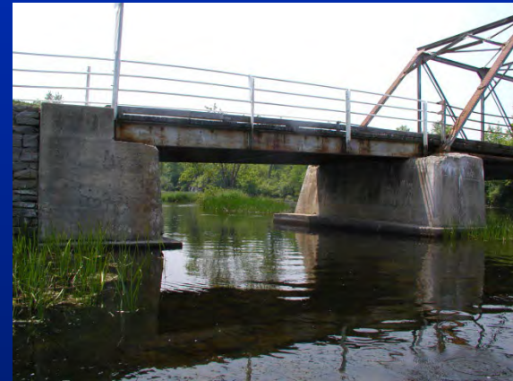
Single span slab-on-girder
