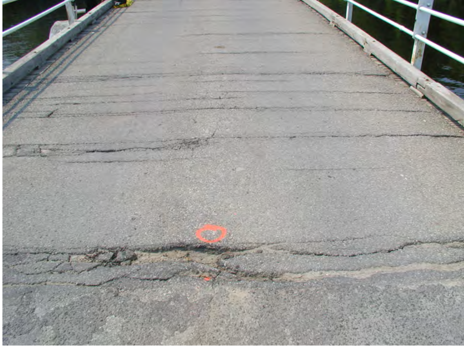
Photograph 7: View of west expansion joint, looking east.
