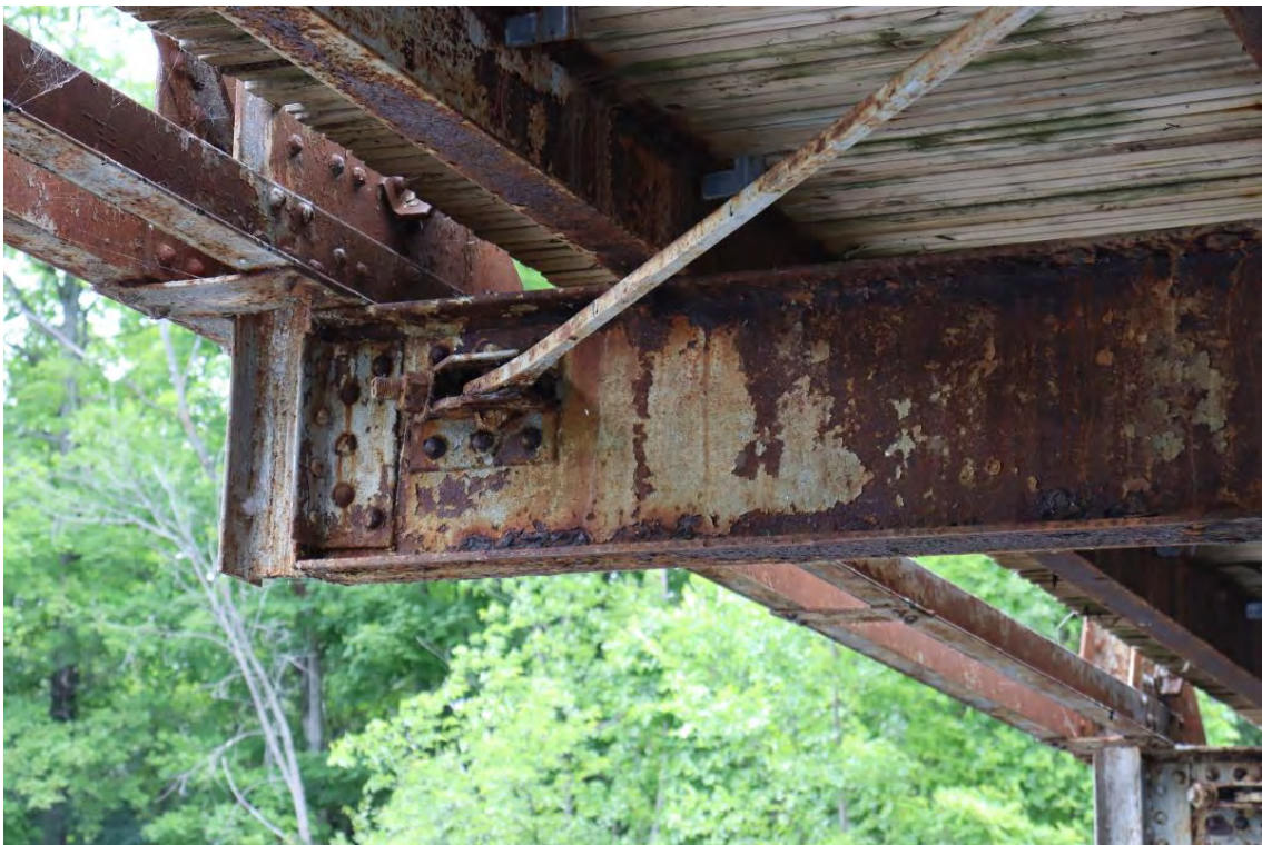
Figure 20: Floor beam 3 south end
