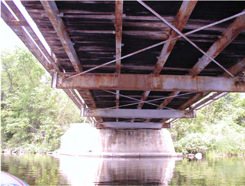
Photograph 13: Configuration of below-deck structural steel in truss span.
