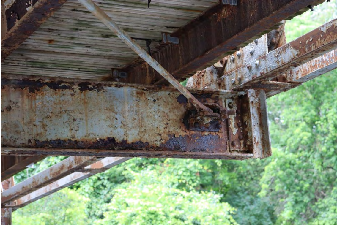
Figure 19: Floor beam 3 north end
