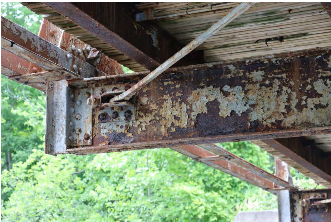
Figure 22: Floor beam 2 south end
