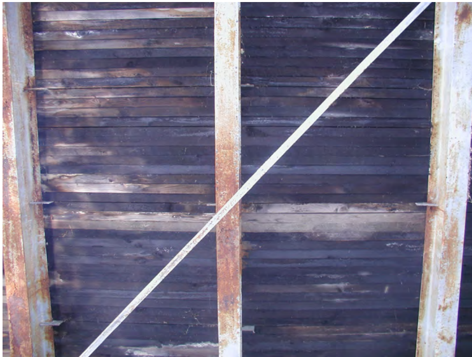
Photograph 10: Typical condition of underside of deck.
