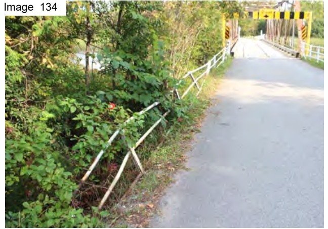
Damaged pipe railing NE quadrant
