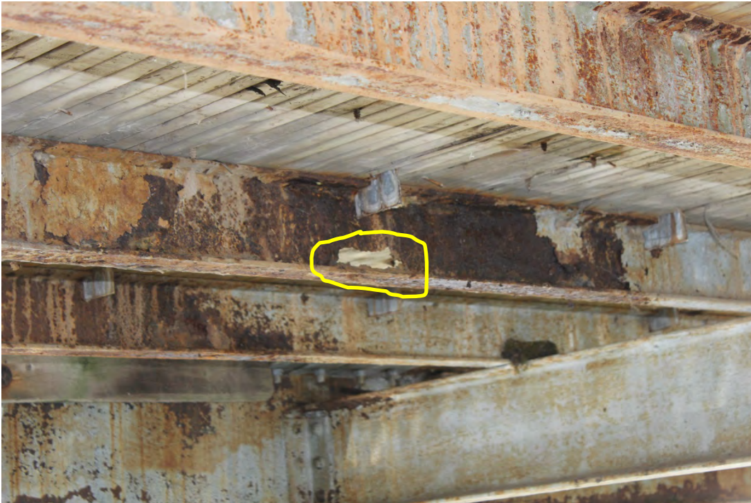
Image 34. Close-up of perforation shown in Image 33
