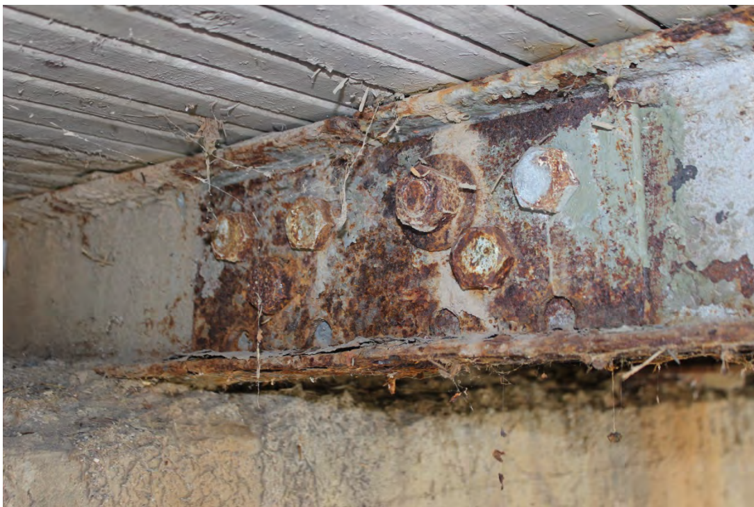
Image 26. Splice on Stringer 4 at east abutment
