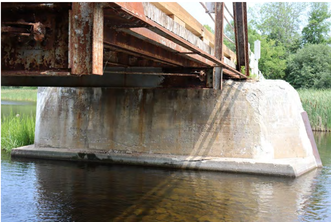
Figure 40: West face of pier
