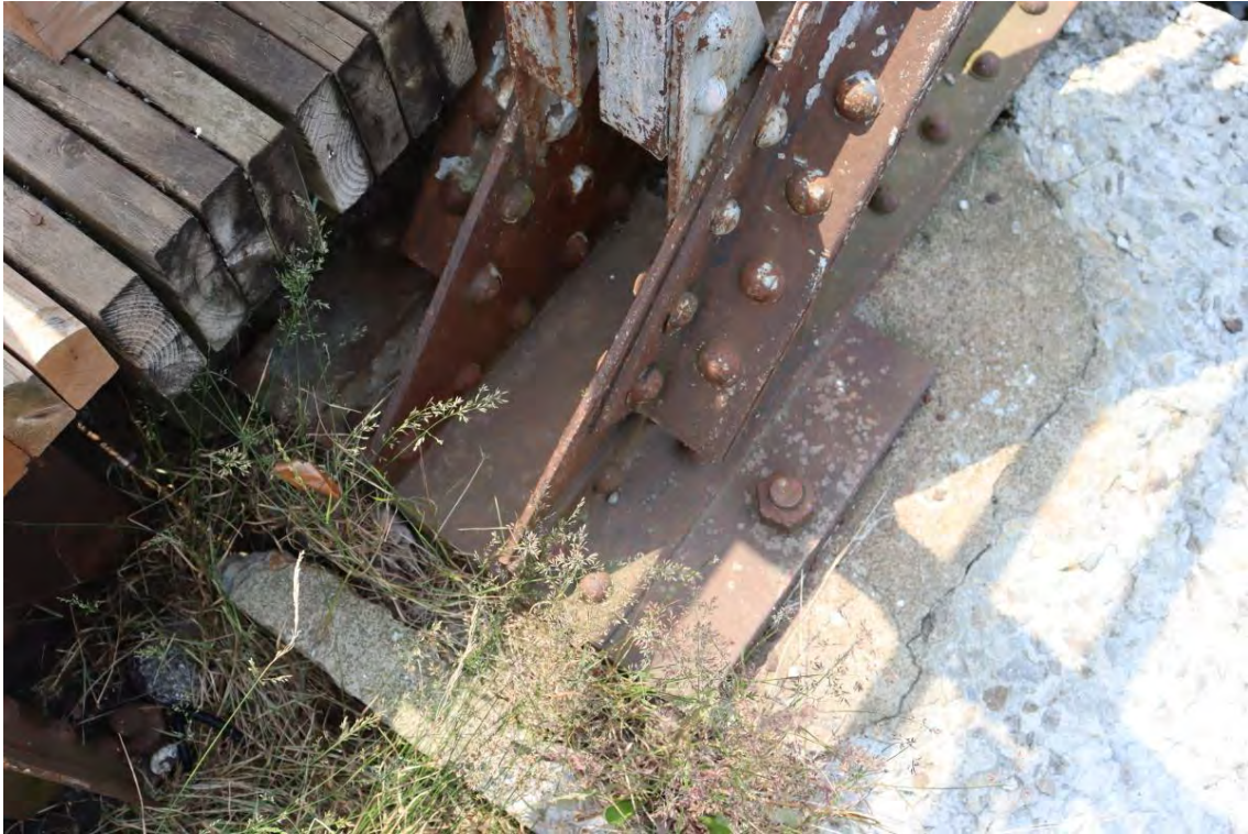
Figure 45: North pier truss bearing
