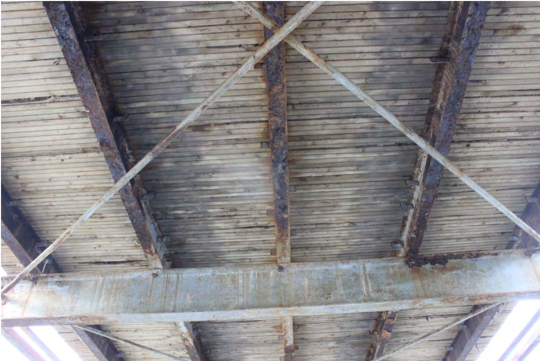
Image 16. Truss Bay 1 looking west
