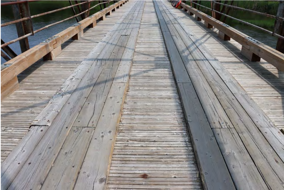
Figure 61: Deck surface looking west
