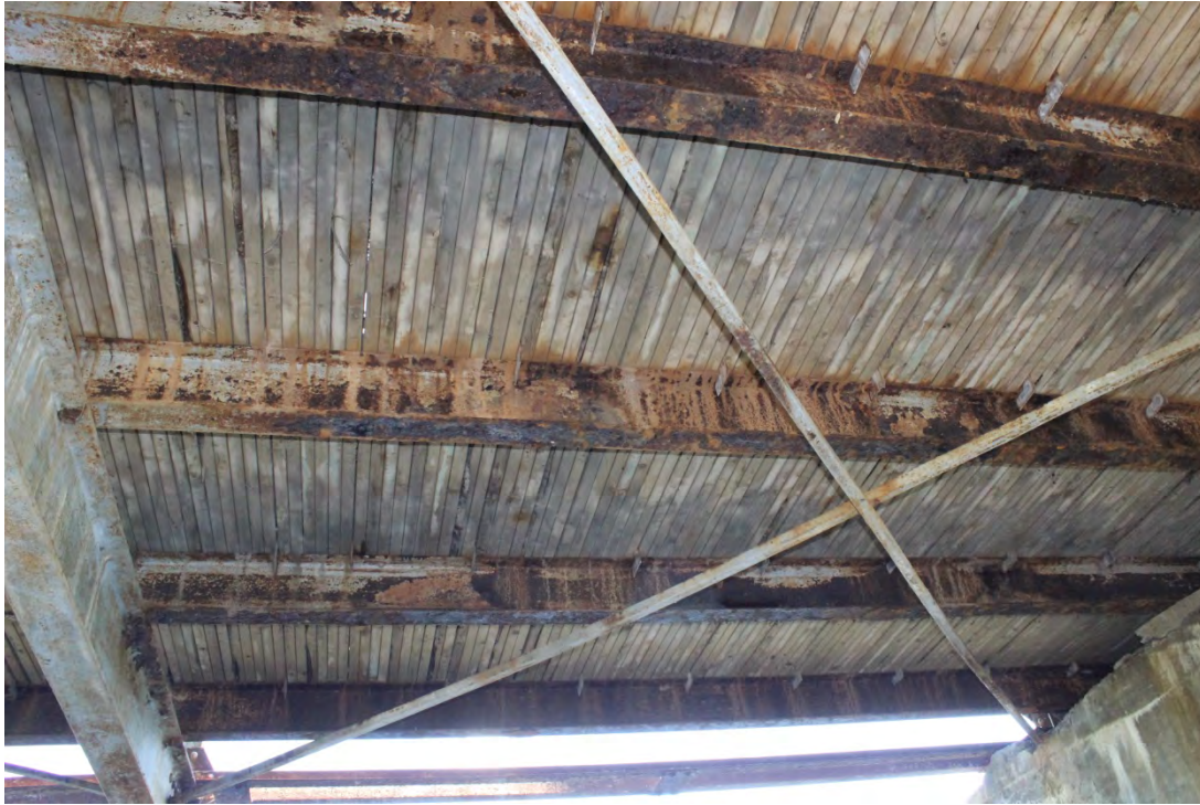
Image 5. Truss Bay 1 adjacent pier, looking downstream
