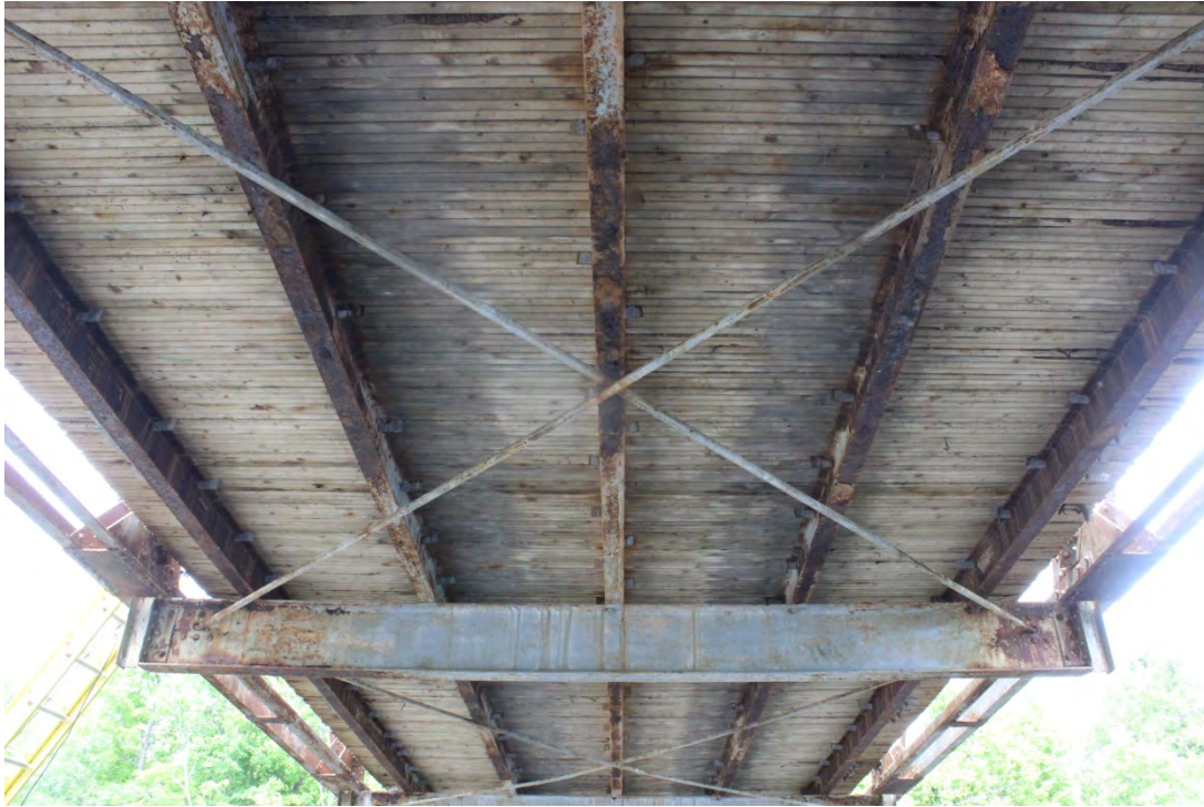
Image 17. Truss Bay 2 looking west
