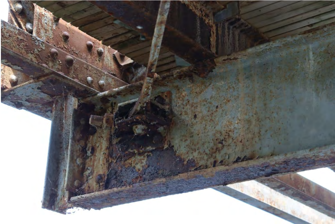
Figure 15: Floor beam 5 north end
