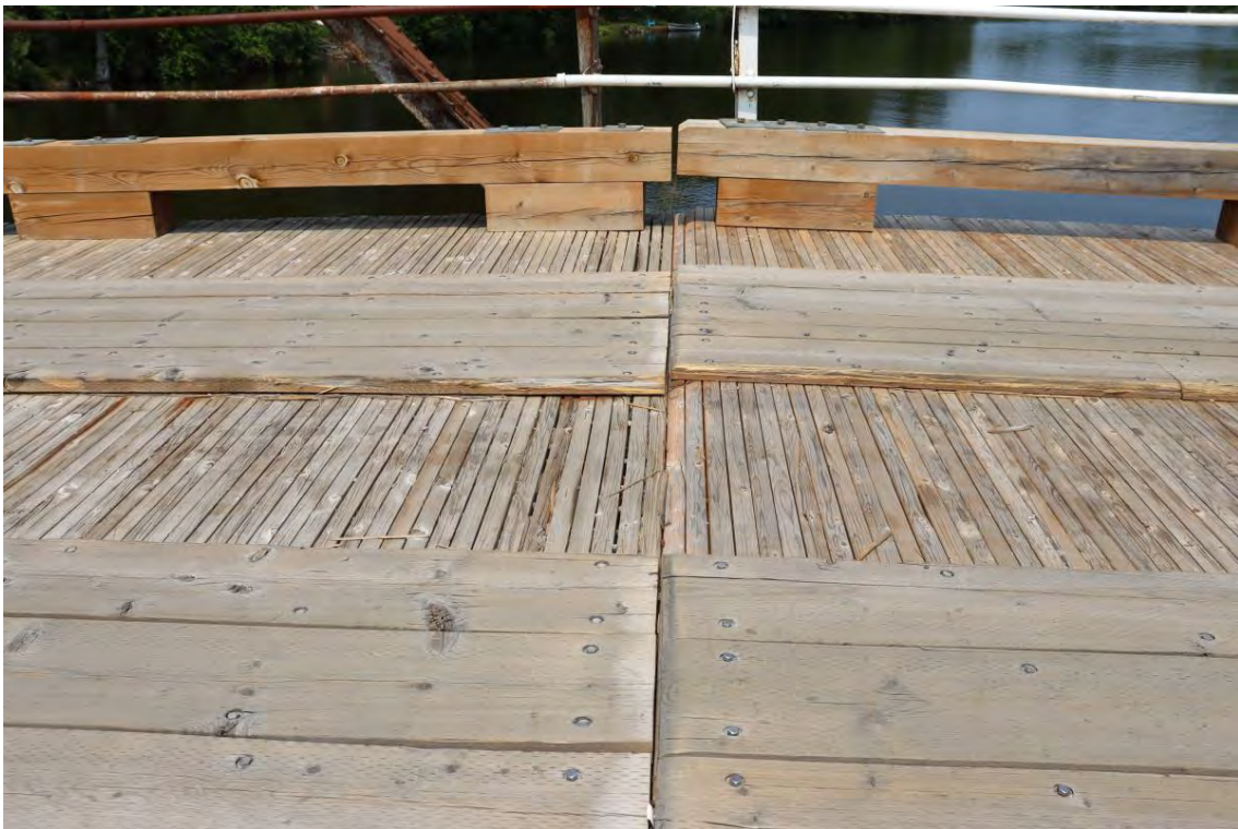
Figure 54: Grade change / bump over pier
