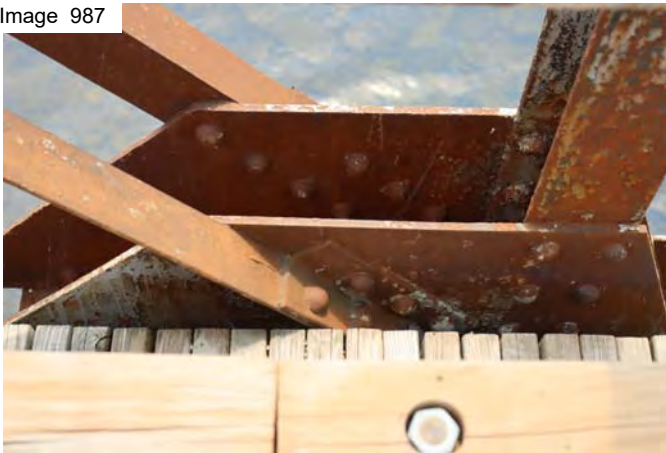
Running boards damage
