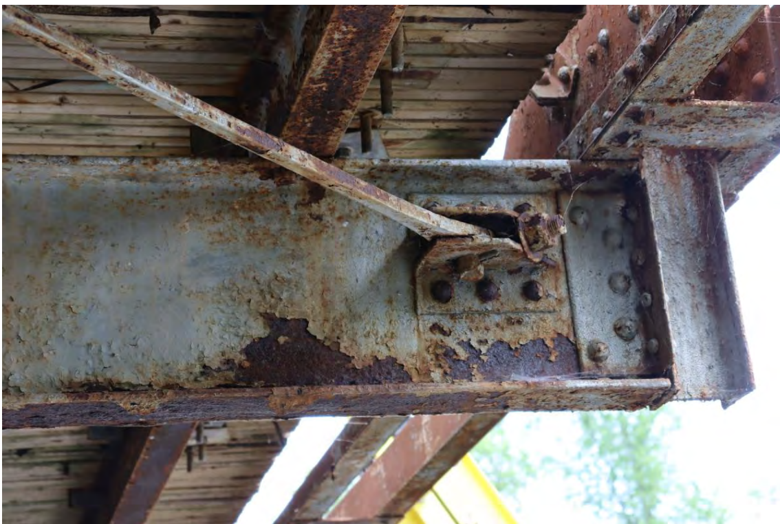
Figure 16: Floor beam 5 south end
