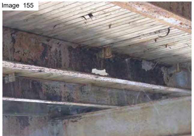
Disintegrating south abutment west side
