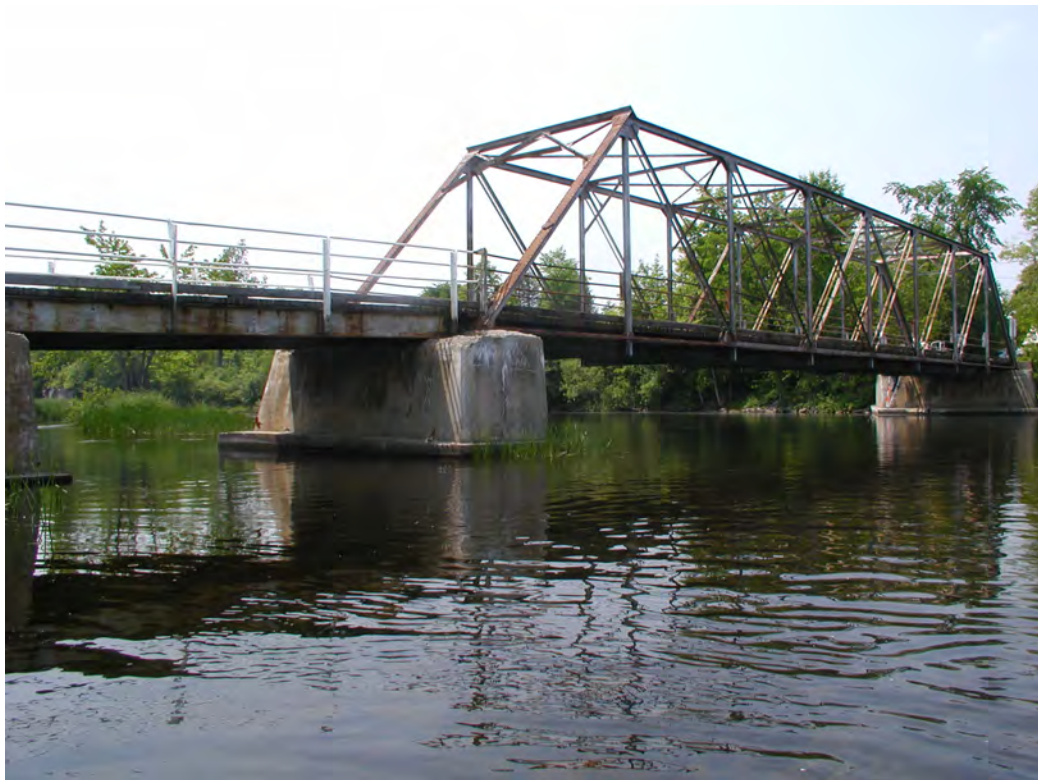
Photograph 2: Detail of truss span and slab on girder span.
