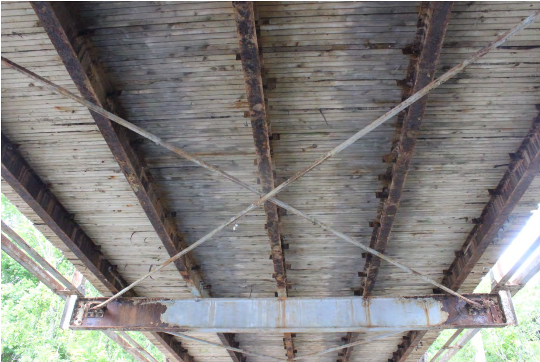
Image 22. Truss Bay 7 looking west
