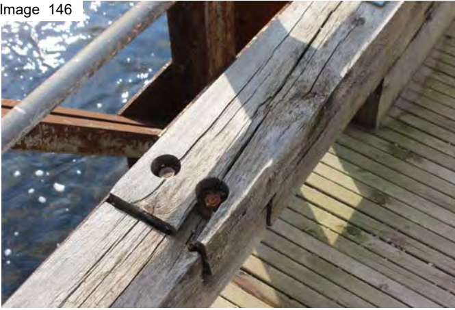
Curb timber decay on truss
