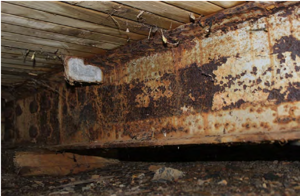
Image 12. North face of truss Stringer 3 at pier bearing
