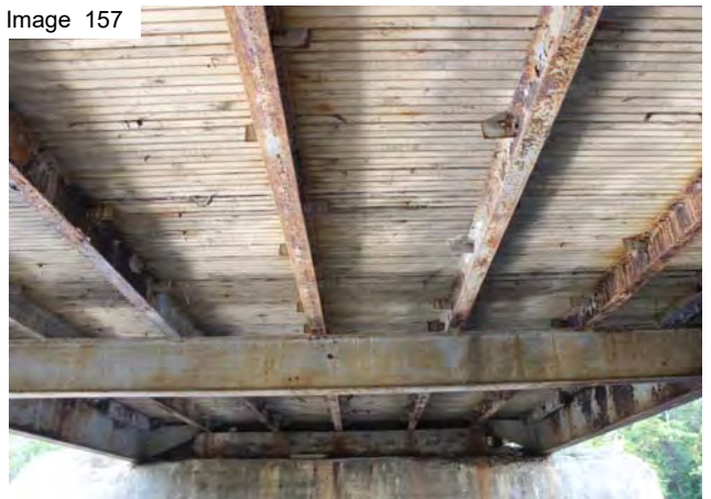
Perforation stringer 2 approach span south end
