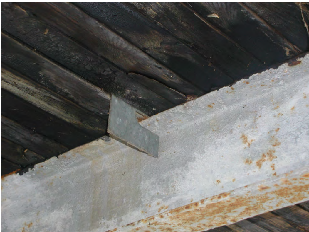
Photograph 18: Detail of clip attaching deck to stringer,
