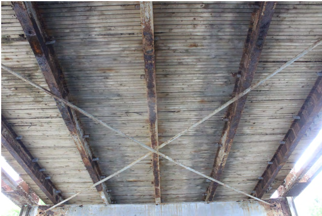
Image 18. Truss Bay 3 looking west
