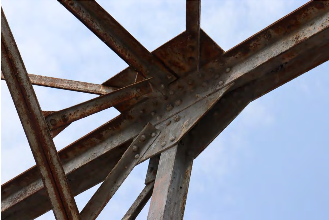
Figure 57: Typical top chord connection
