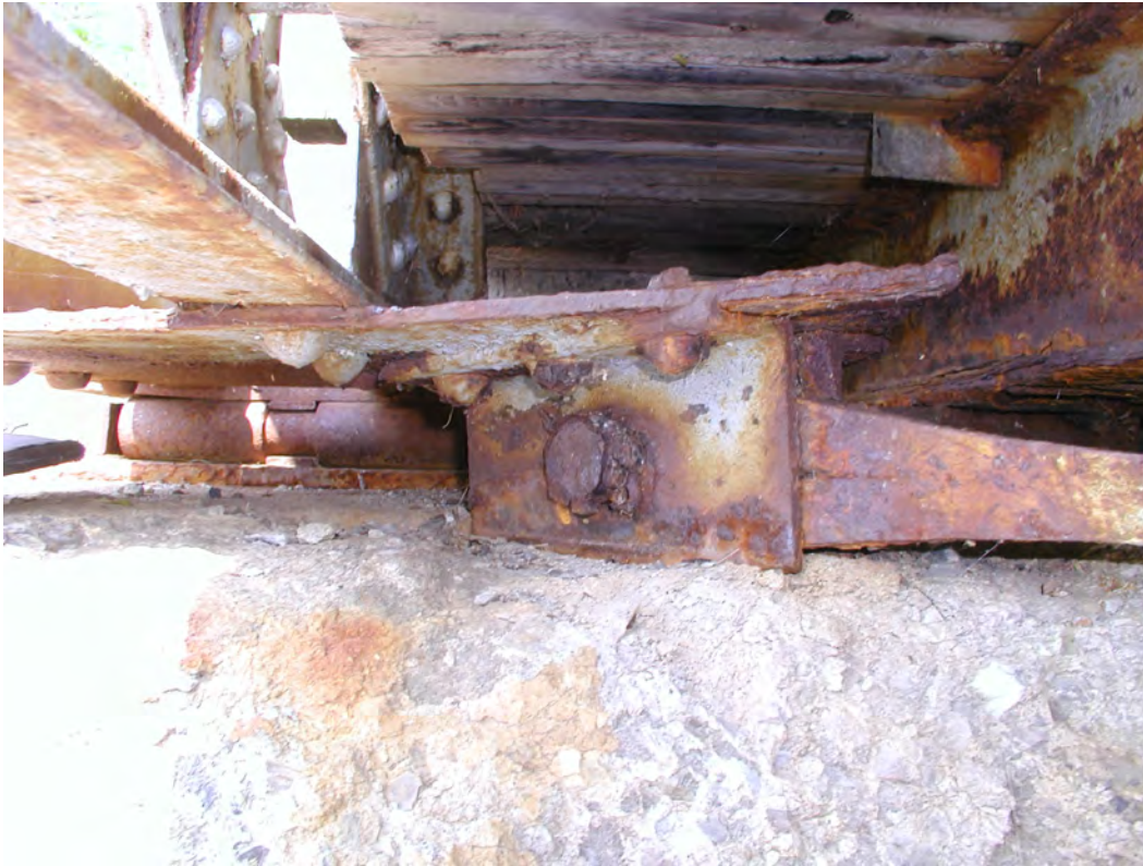
Photograph 23: Detail of south roller bearing at West Abutment.
