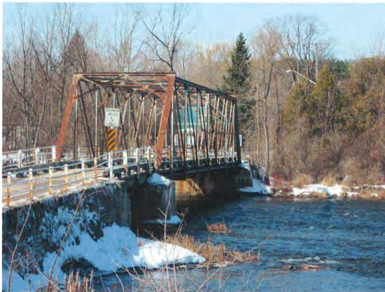
Photograph 1: East elevation, looking northwest.
