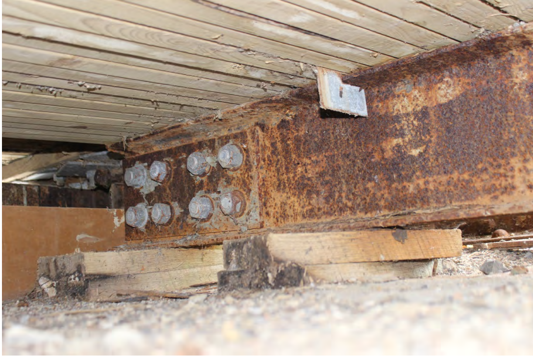
Image 7. Truss Stringer 1 at Pier Bearing
