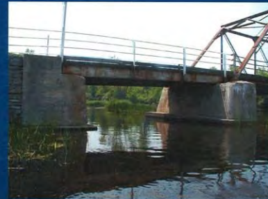
Single span slab-on-girder
