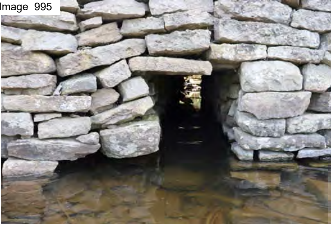
Culvert through causeway
