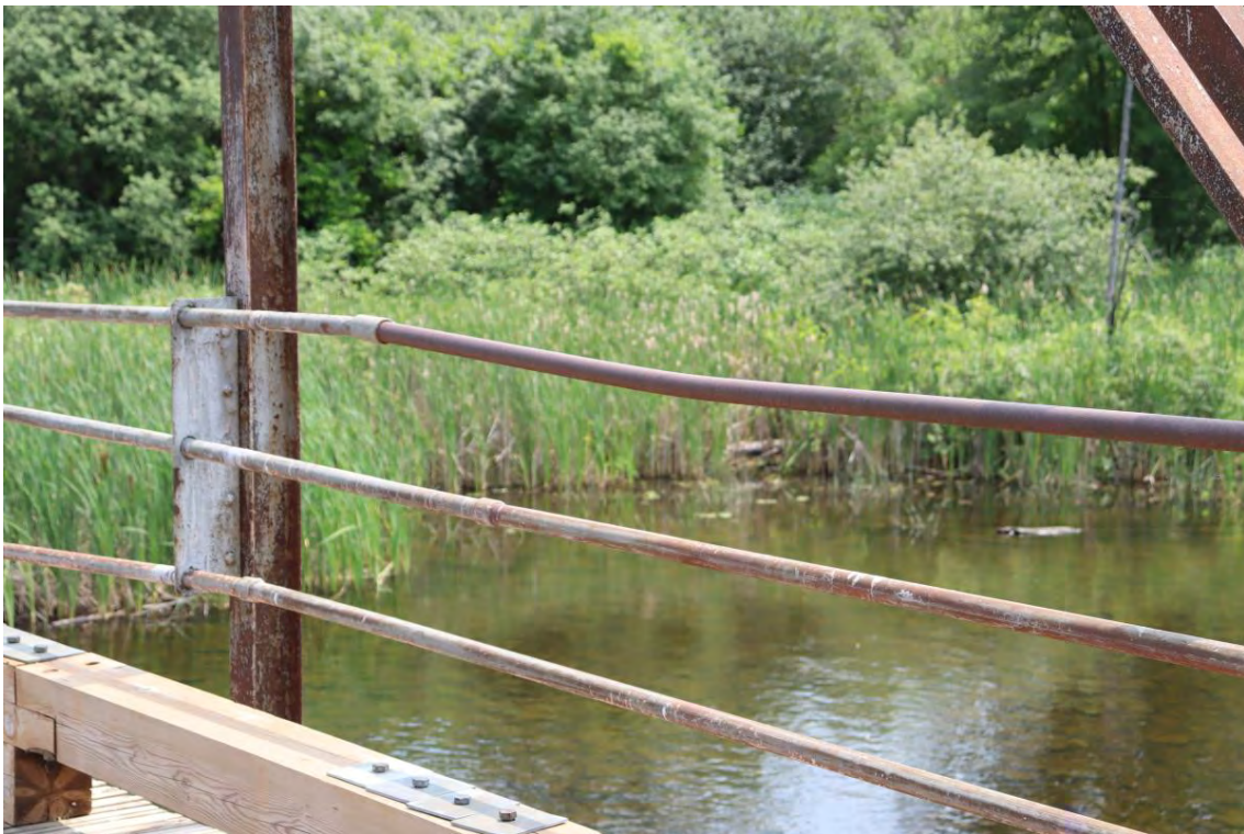
Figure 58: South pipe railing
