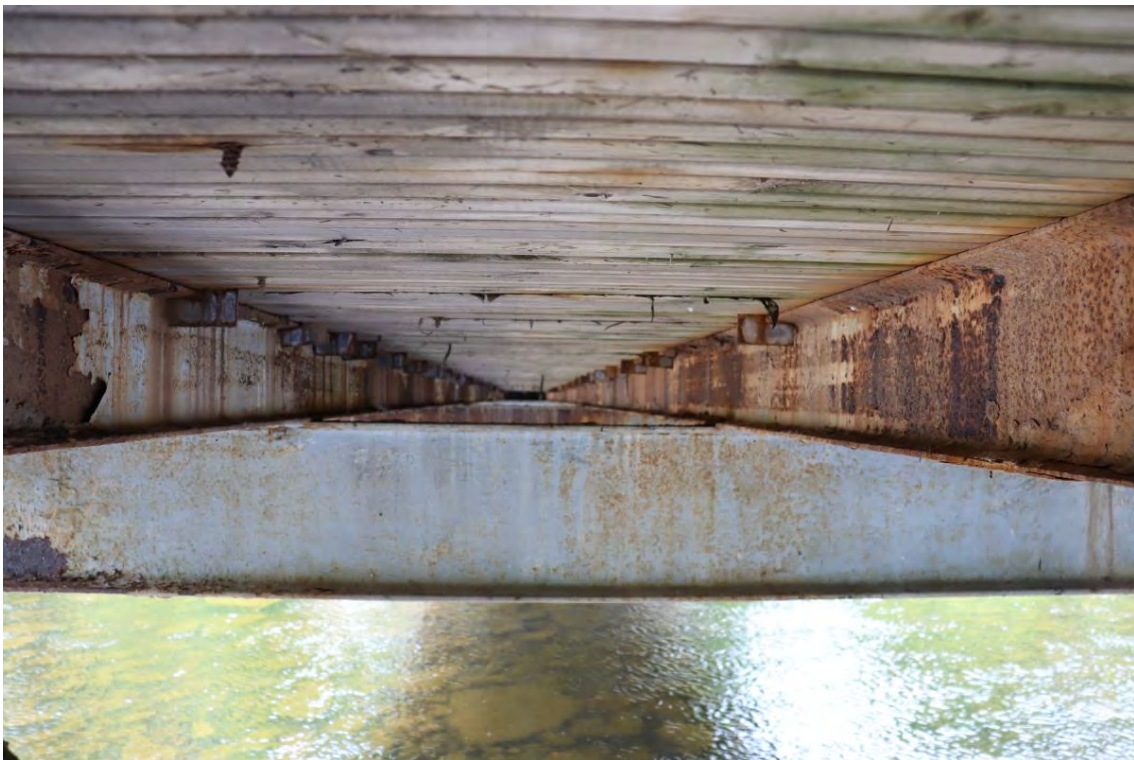
Figure 38: Looking west between stringers 2 and 3
