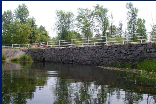
Single span slab-on-girder
