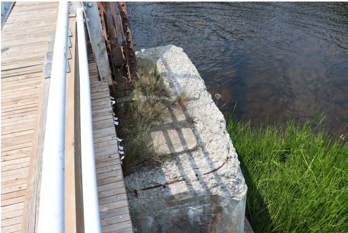
Figure 46: Pier top north end
