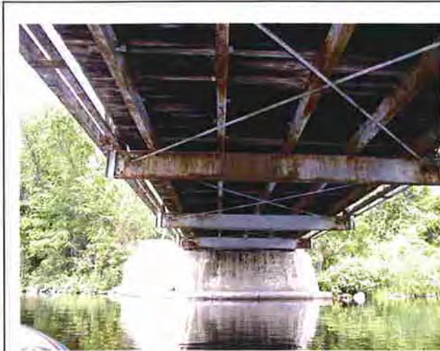
Photograph 6: Typical condition of below-deck structural steel in truss.
