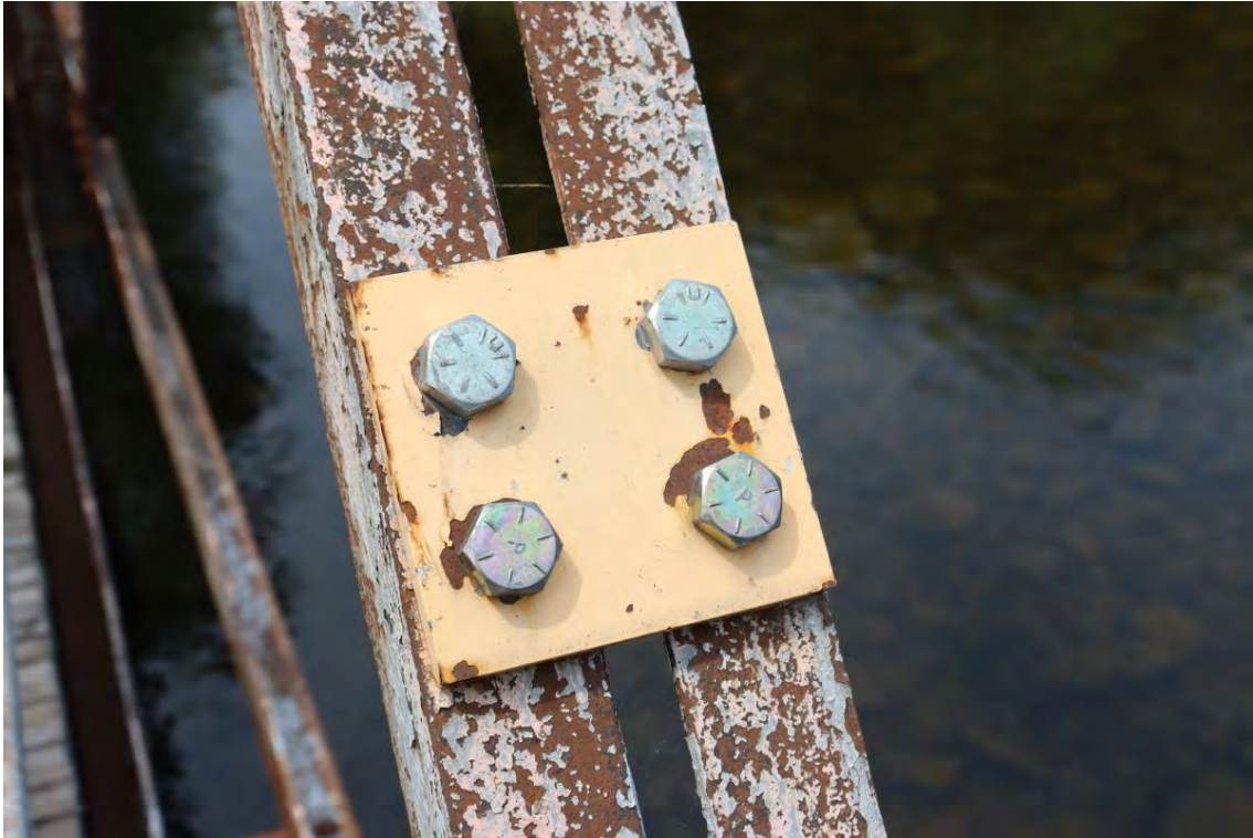
Figure 59: Typical compression diagonal bracing tie plate
