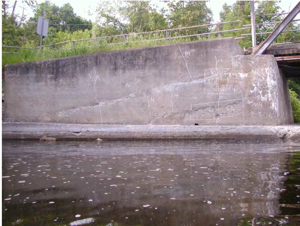
Photograph 27: Elevation of south wingwall at West Abutment.
