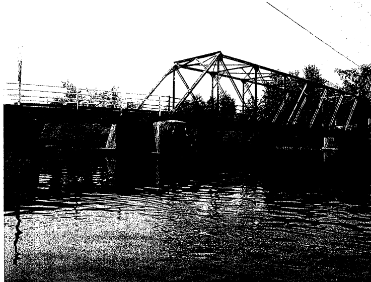
Photograph 1: South elevation of Andrewsville Bridge as viewed from the southeast quadrant.
