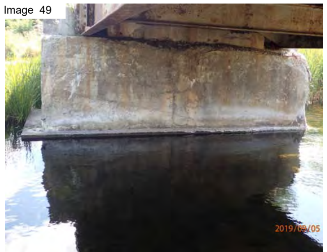
East abutment wall
