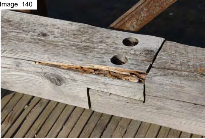
Decay in curb timber
