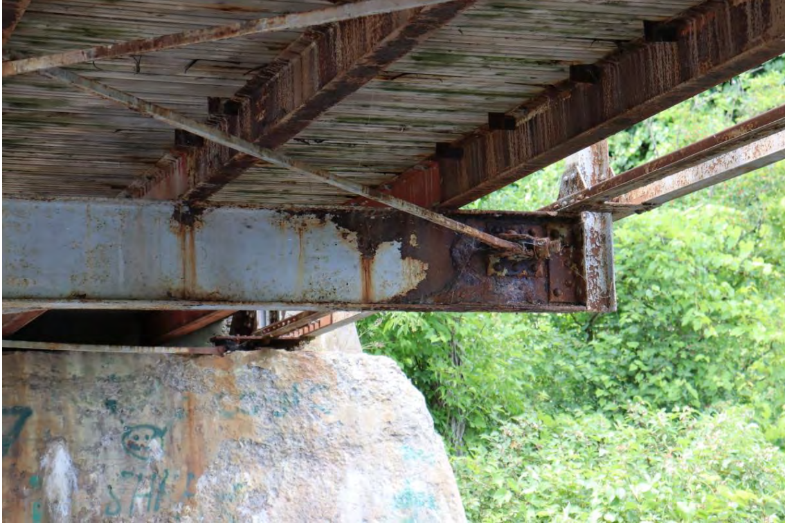
Figure 23: Floor beam 1 north end
