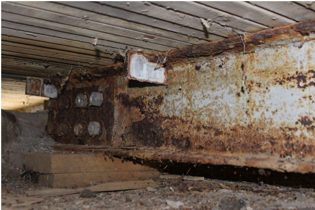
Image 8. Truss Stringer 2 at Pier Bearing
