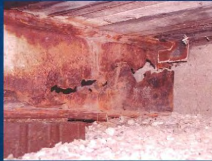
Condition of stringer, June 2005
