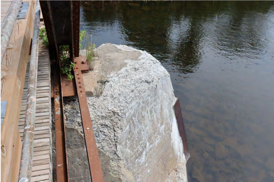
Figure 55: Pier top south side from west
