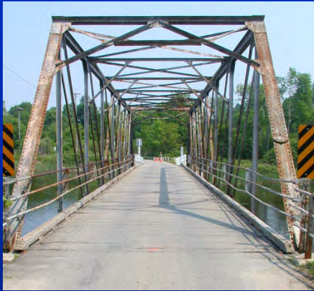
Single span steel truss
