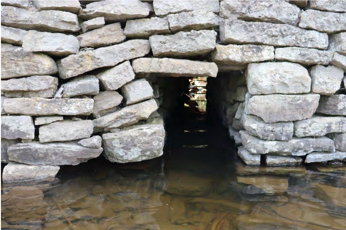
Figure 51: Drainage opening through causeway
