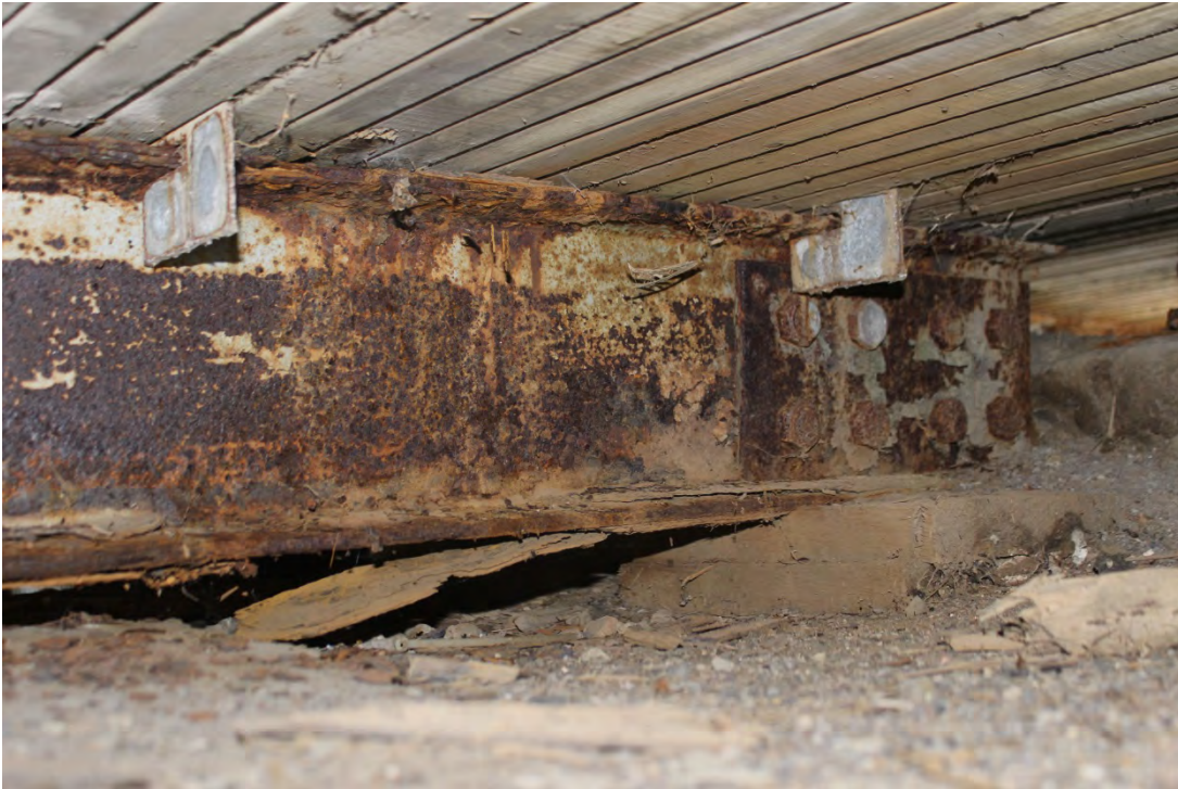
Image 10. Truss Stringer 4 at Pier Bearing
