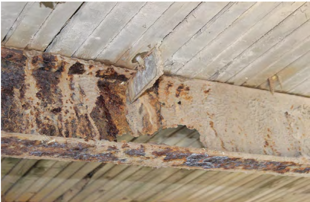
Image 14. Perforated Stringer 2 west end approach span, looking north
