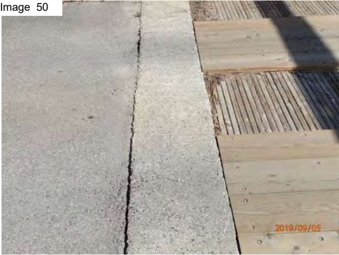
West end of deck
