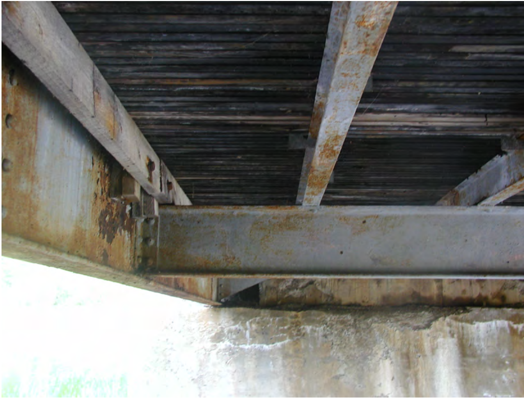
Photograph 17: Configuration of below-deck structural steel in slab-on-girder span.
