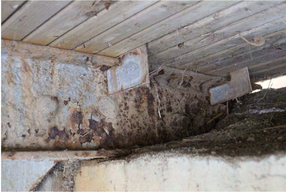
Image 25. Stringer 5 bearing area at east abutment
