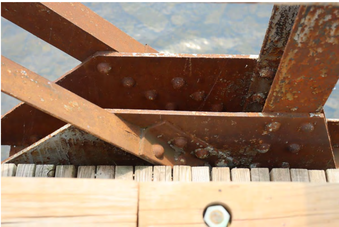
Figure 56: Typical bottom chord connection
