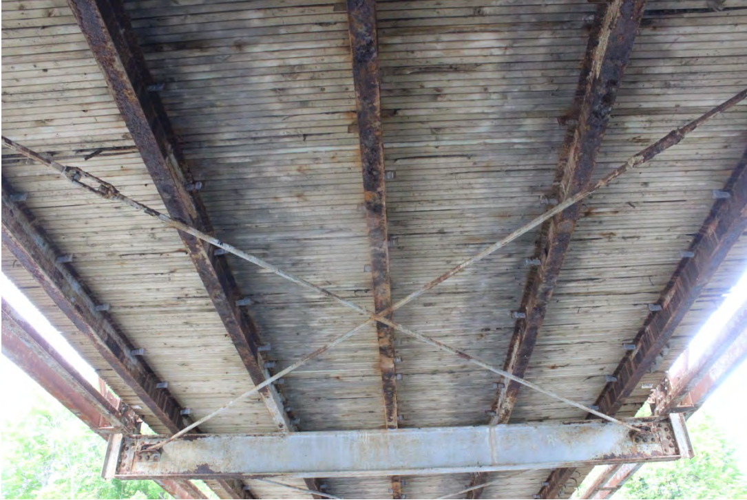
Image 19. Truss Bay 4 looking west
