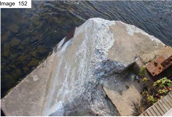
Disintegrating pier nosing
