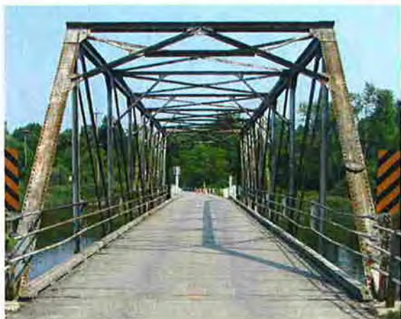
Photograph 2: View across truss, looking east.
