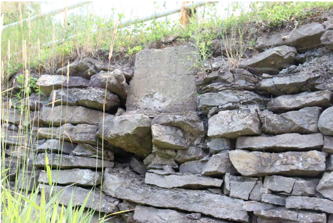
Figure 50: North-east quadrant dry-stone retaining wall
