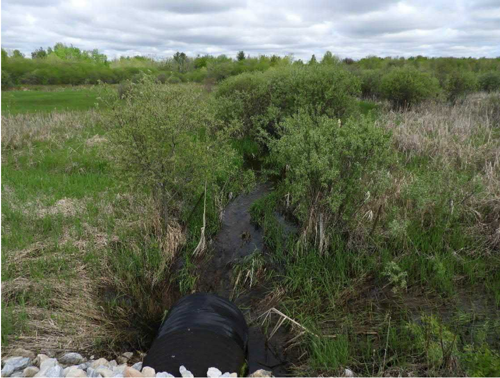
Photo 35: Culvert inlet on North Street conveying a tributary of Tay River within the Cattail Graminoid Organic Meadow Marsh (MAMO1-2) vegetation community in the southeast end of the study area. 24 May 2019.
