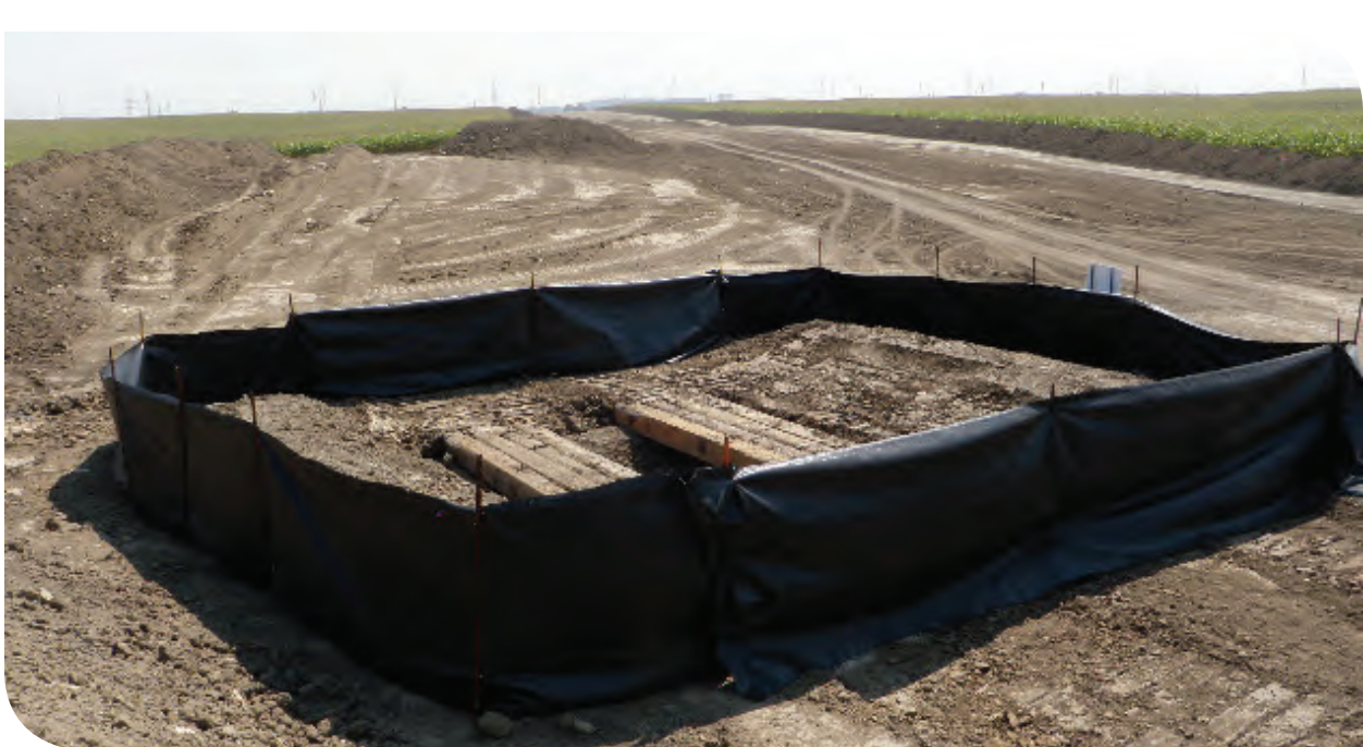
Cleaning station at construction site.
