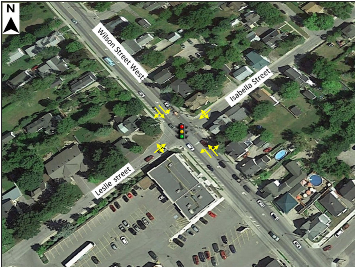
Figure 3.2.8 Intersection of Wilson Street and Isabella Street/Leslie Street (Source: Google Earth)
