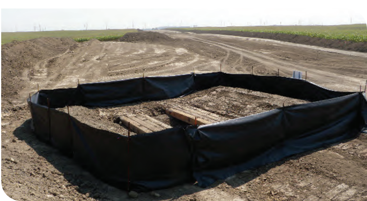
Cleaning station at construction site.
