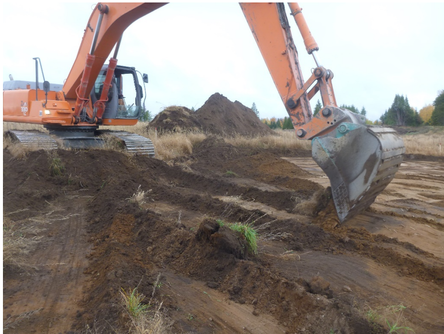
Image 4: Excavator conducting mechanical topsoil removal view northeast.
