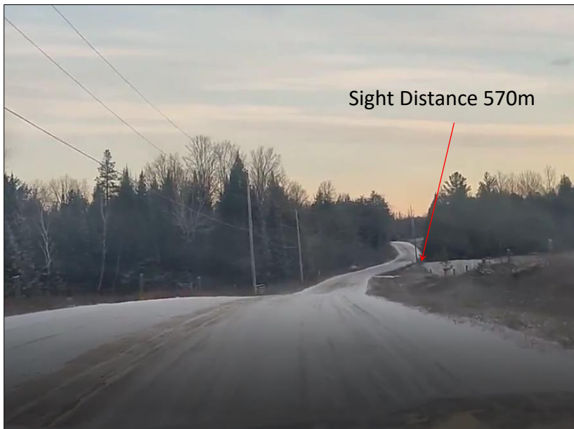
Exhibit 5-12: Alternative Access 2 (EA1) Location Looking East (570m)
