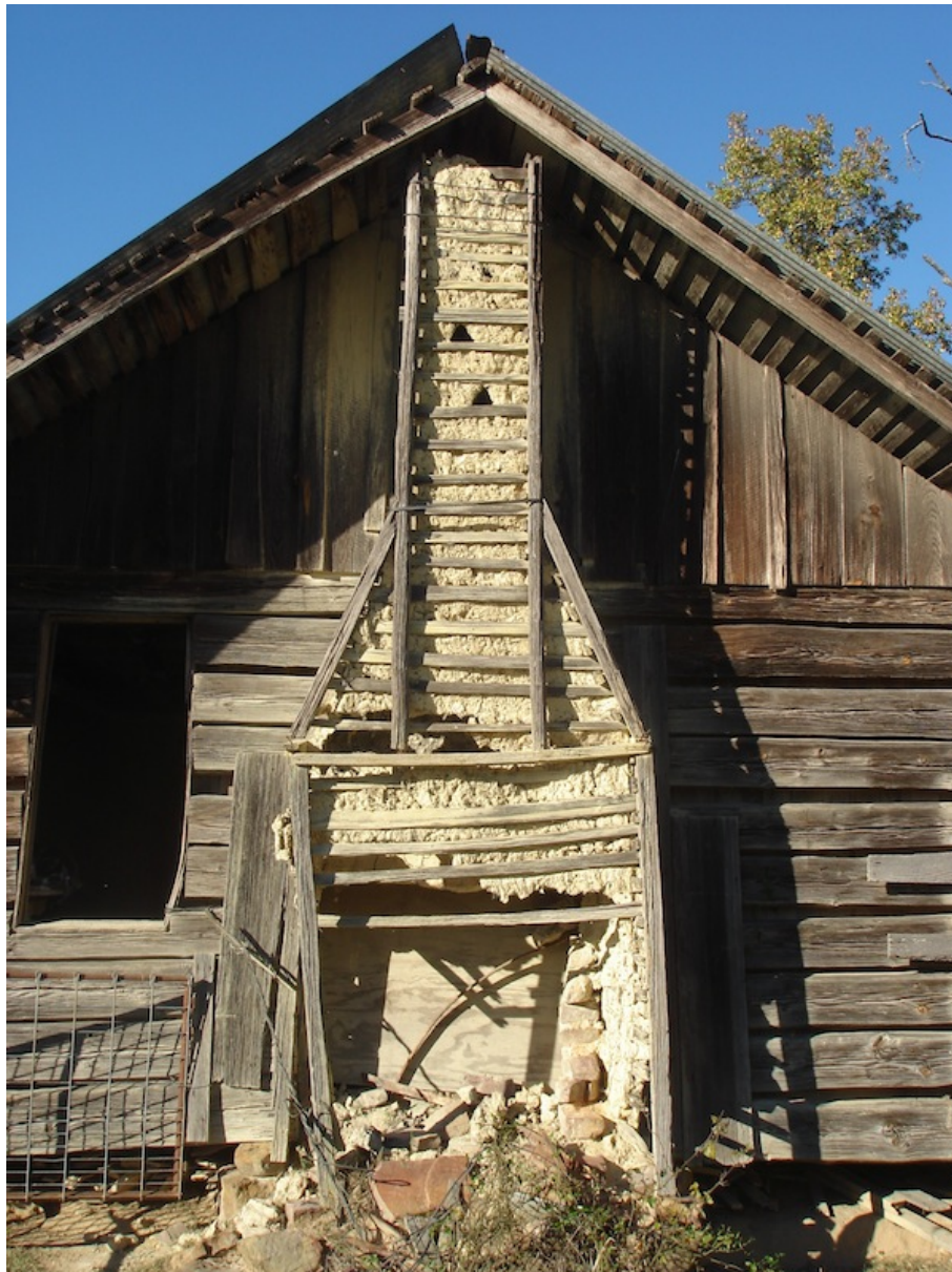
Image 59: Photo of a stick and mud chimney from a historic log house (Caddo Heritage Productions 2013). Note the field stones used in the construction of the base.
