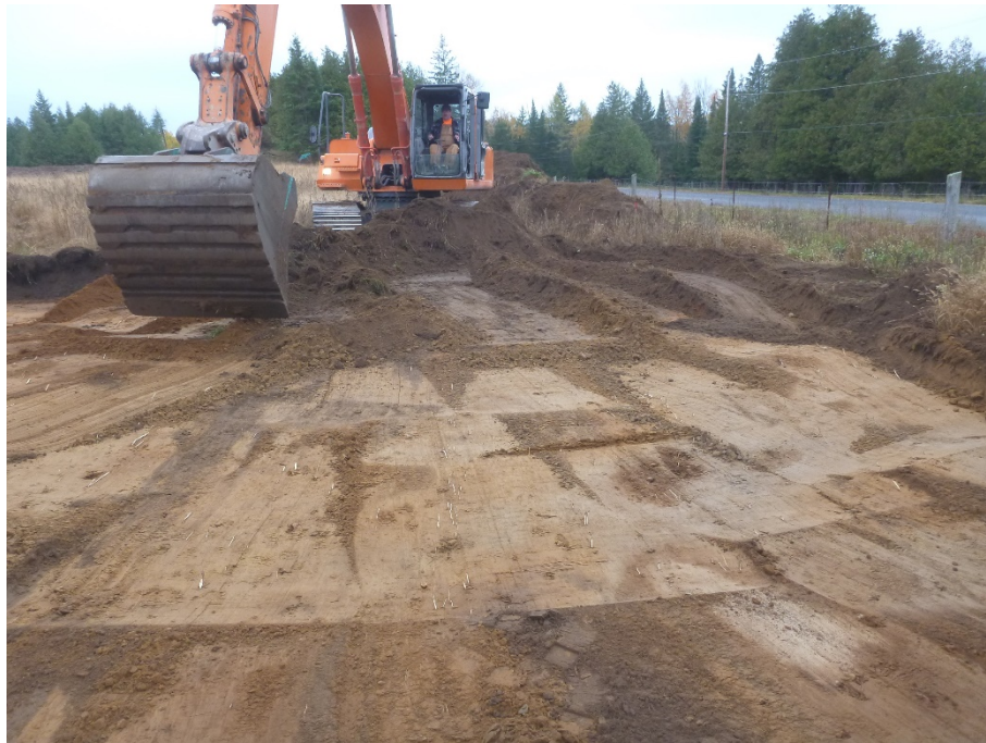
Image 3: Excavator conducting mechanical topsoil removal along the property fenceline, view southwest.
