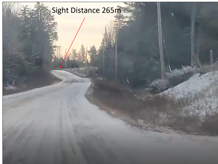
Exhibit 5-10: Alternative Access 1 (EA1) Looking East (265m SD)
