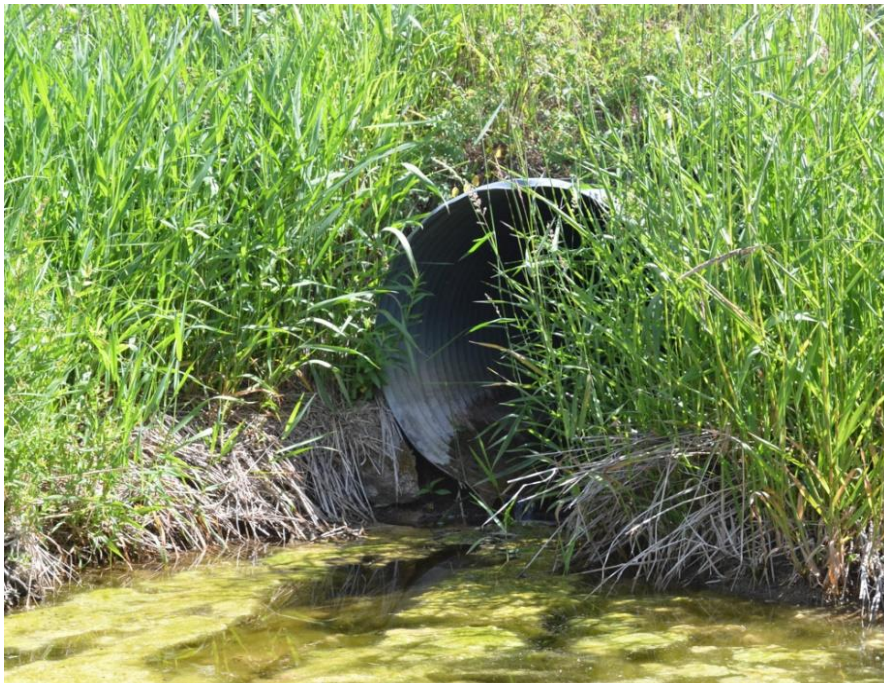
Photo 12 – South of the site, the culvert under Old Almonte Road is perched at the downstream (west) end. View looking east
