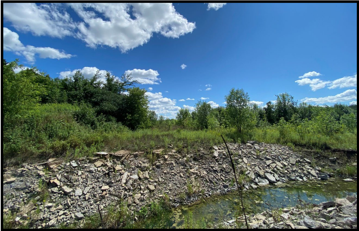
Figure 1: Overview from northeast corner (PA1189-D01).
