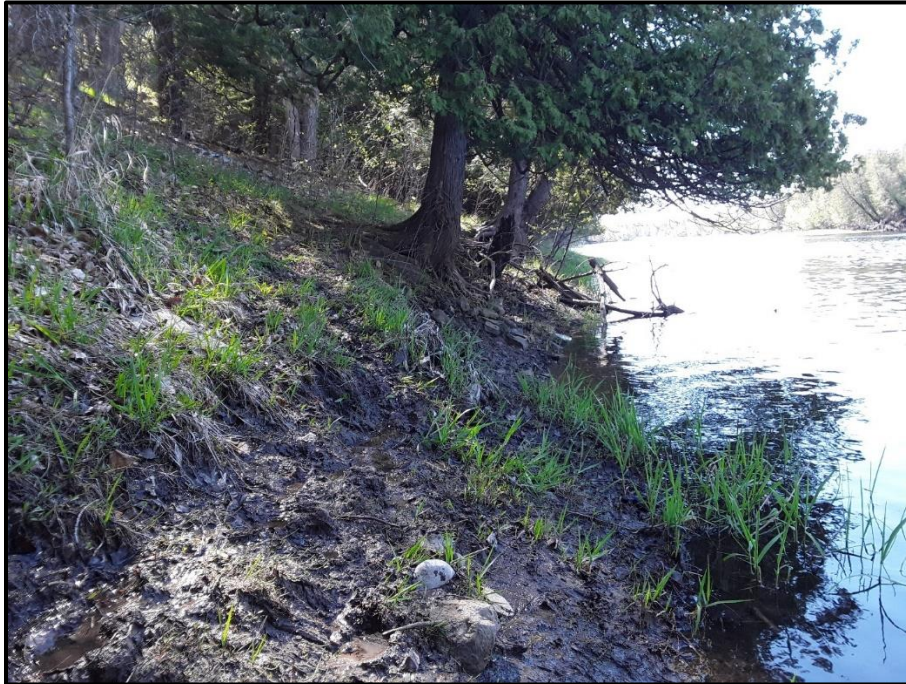
Image 19. View of the steep slope down to the river with wet soils at the foot, facing southeast. (PR21-011D020)
