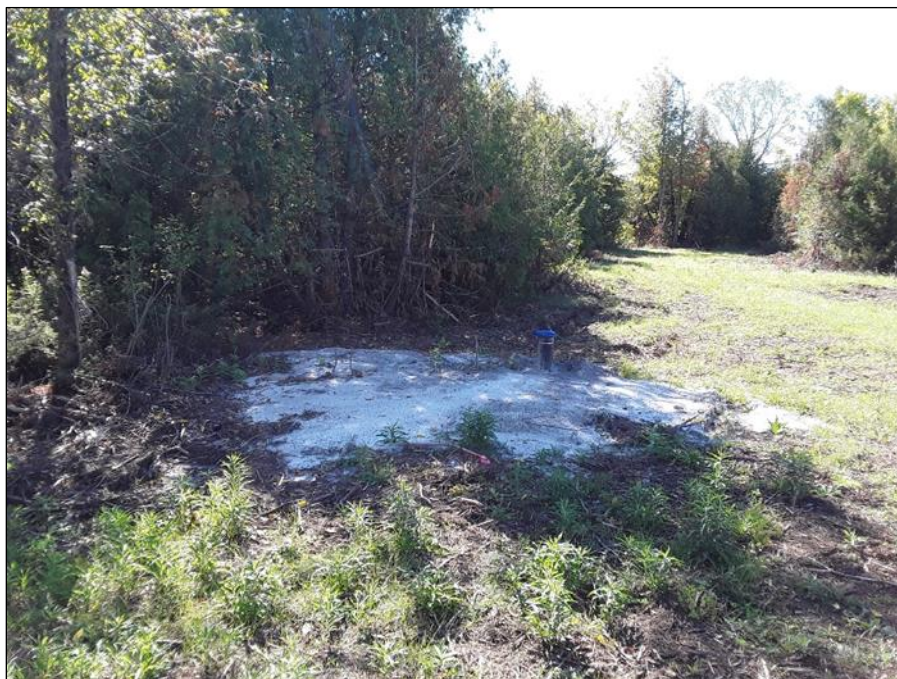
Image 14. View of a recently drilled well within a former agricultural field in the southern portion of the study area, facing east. (PR21-040D017)
