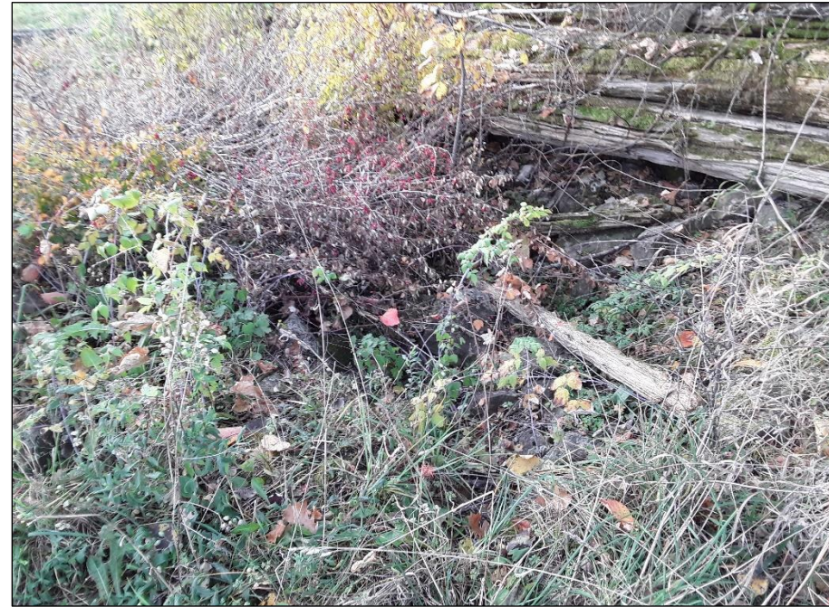
Image 33. View of fallen wood beams associated with stone foundation located along the western edge of the study area, looking north. (PR20-030D108)
