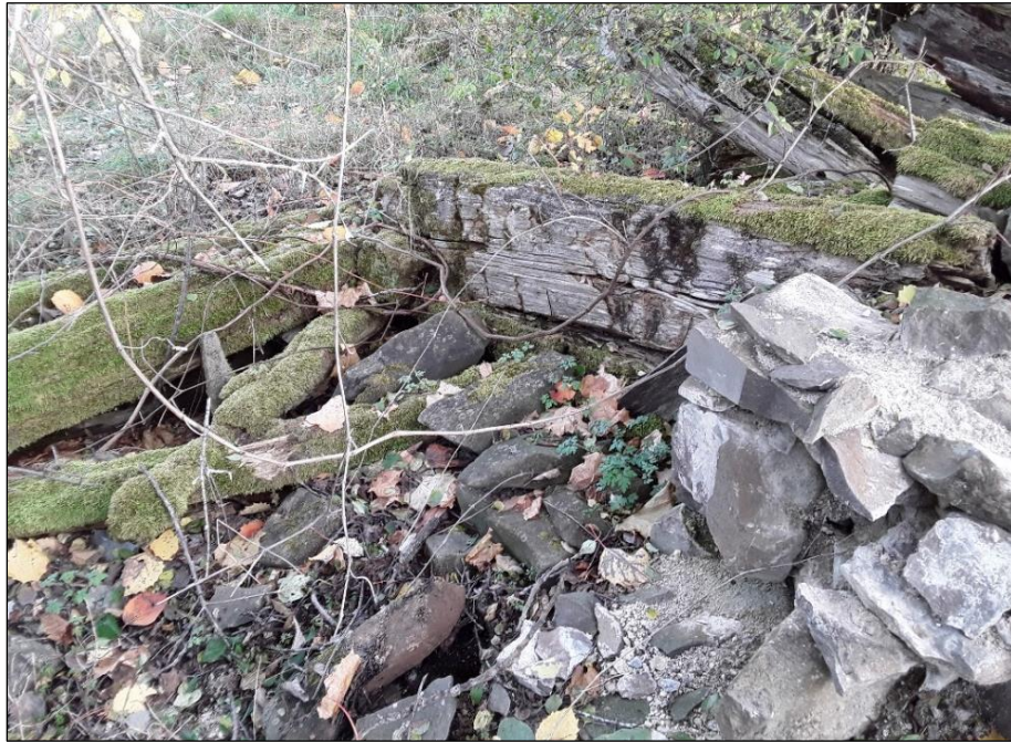
Image 31. View of stone foundation found along the western edge of the study area, looking north. (PR20-030D105)
