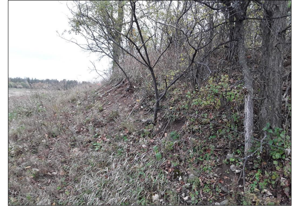
Image 23. View of steep slope along the northwestern edge of former quarry pit in the southeastern section of the study area, looking northeast. (PR20-030D072)
