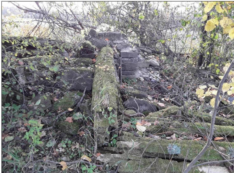
Image 32. View of stone foundation found along the western edge of the study area in the general location of outbuilding identified in historic mapping, looking southeast. (PR20-030D106)
