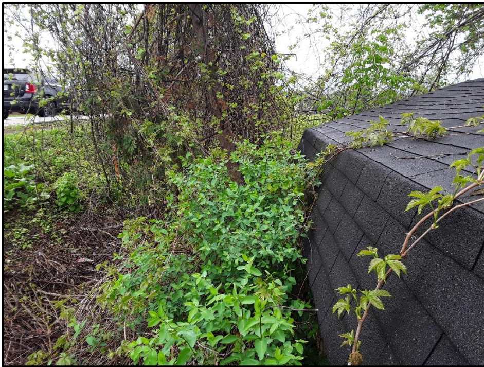
Image 20. View of the northeastern corner of property, facing northeast. (PR22-022D053)
