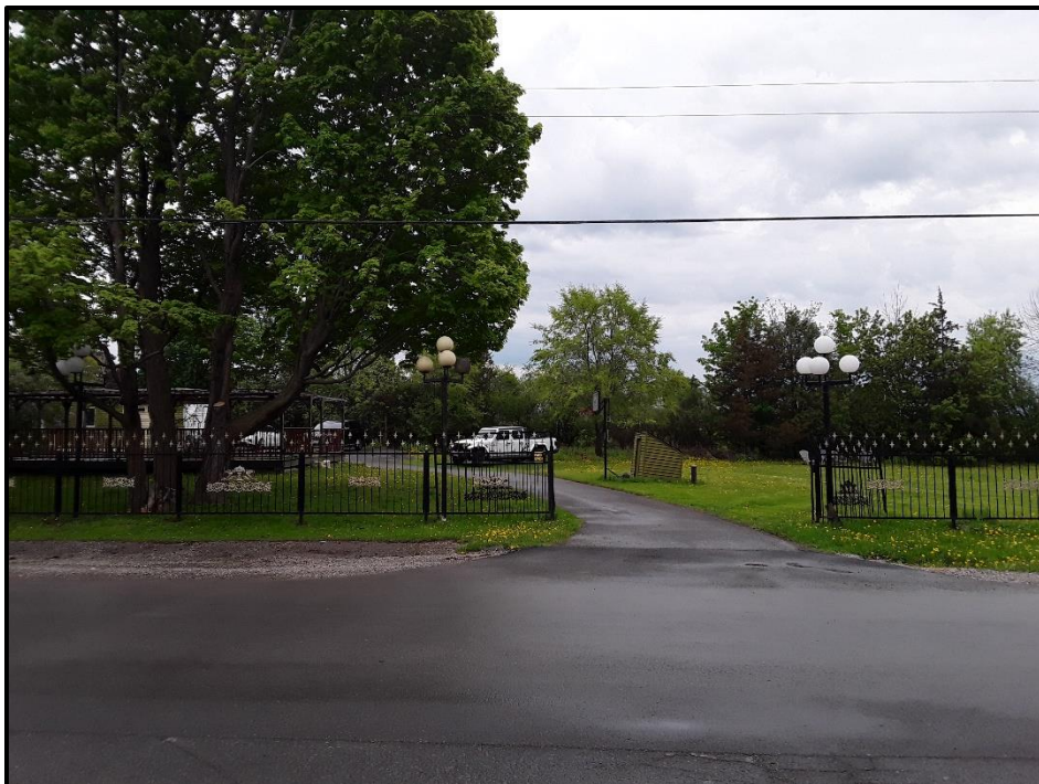
Image 22. View of the central curved driveway, facing east. (PR22-022D057)
