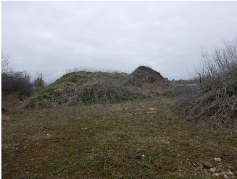
Photo 4: Soil Stockpiles (May 3, 2022).
