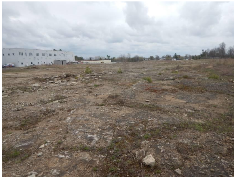
Photo 1: Cleared Area (May 3, 2022).
