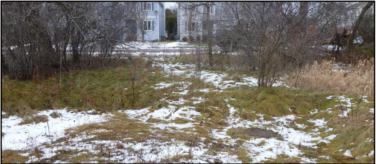
Image 12. Remains of a concrete foundation within a shallow depression, showing Boyd Street in the background, looking northeast. (PR20-39D023)
