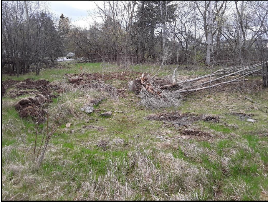
Image 23. View of the buried residential foundations with an exposed concrete corner, looking east. (PR20-39D082)
