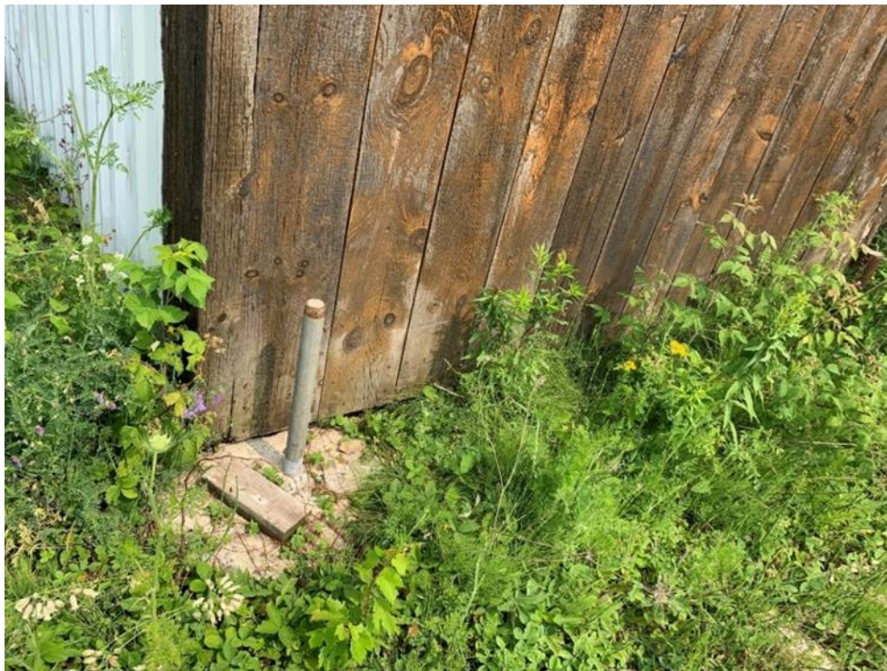
Photo 10: A view of the bottom of the structure in the western portion of the study area (potential snake hibernacula), June 29, 2023.
