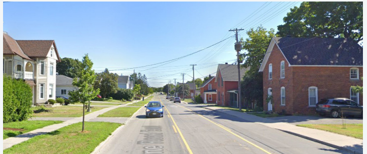
Figure 5: Detached homes along townline road east (2022)
