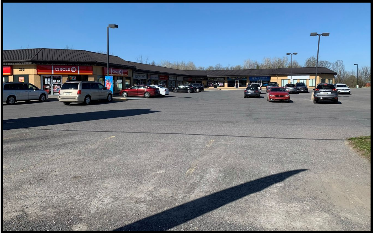
Figure 1: Overview of strip mall and parking lot area (D32).
