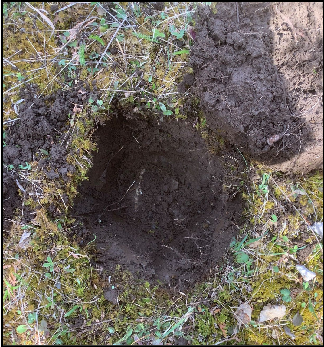
Figure 13: Test pit showing shallow bedrock (D14).
