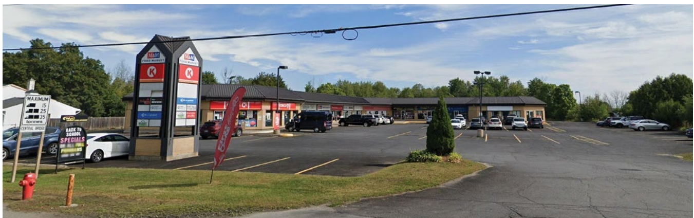
Figure 2: Street view of the subject property looking north on Franktown Road.
