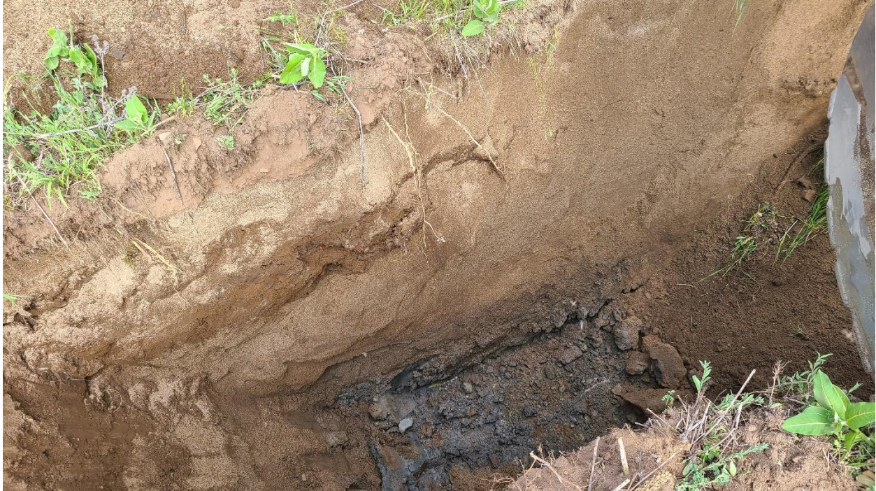
Photo 1: Subsurface Profile in Test Pit No. 2
